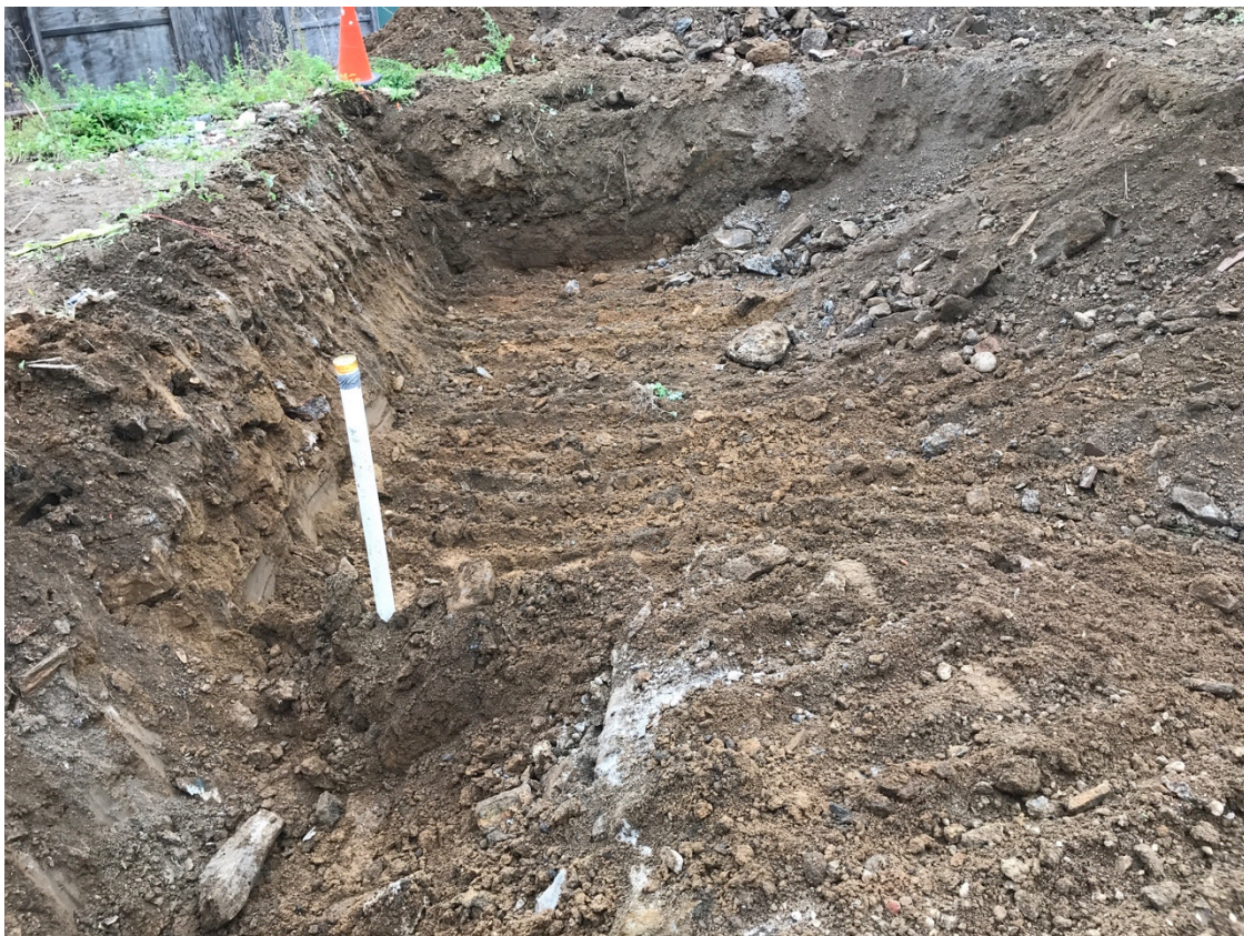
Photograph 8. Bedrock Shelf Exposed to the Right of Monitoring Well in Trench C.
