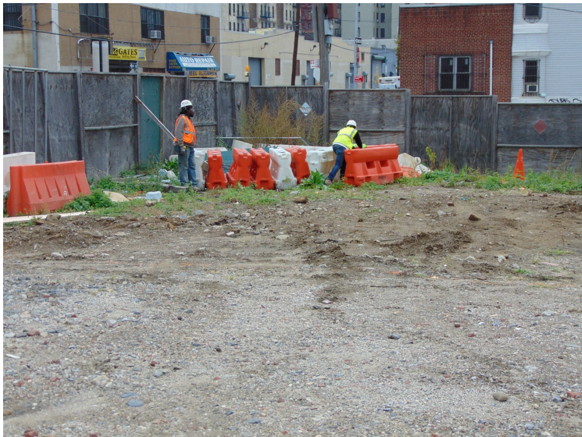
Photograph 6. View of the Location of Trench C.
