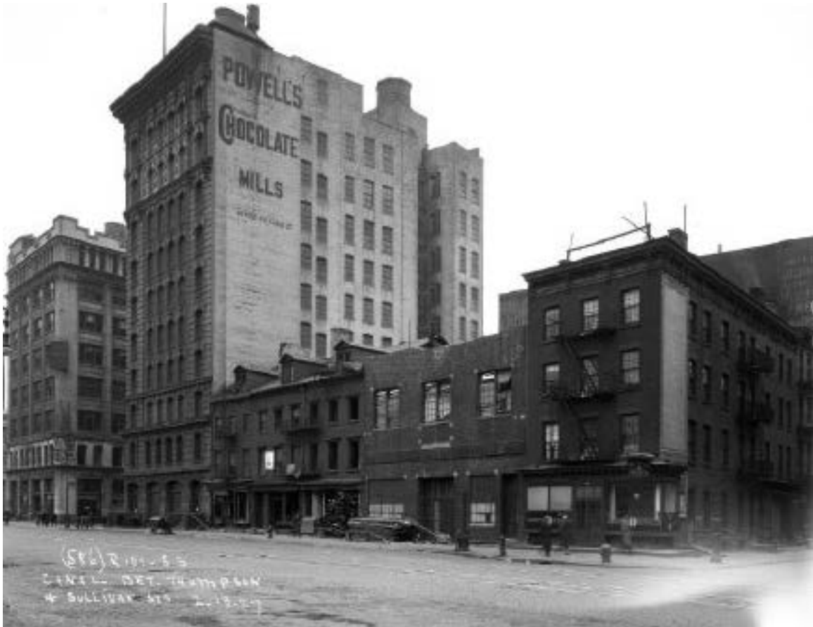
Figure 15. Block 227 (including the Option 1 Archaeological Area of Potential Effect) on the north side of Canal Street between Thompson Street and Sullivan Street, February 13, 1927, prior to demolition for the Sixth Avenue Extension and Eighth Avenue Subway, facing northwest. Museum of the City of New York.
