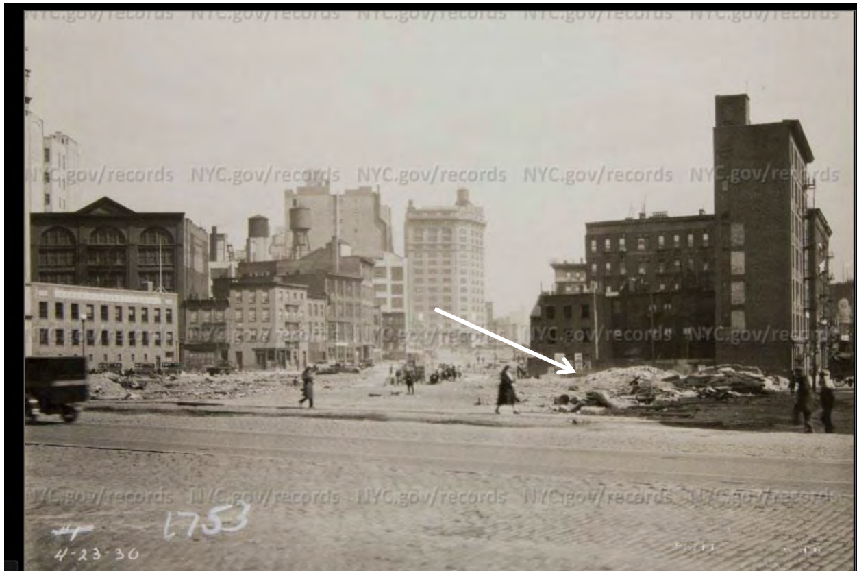
Figure 17. Looking north from Canal Street during construction of the Sixth Avenue Extension, April 23, 1930. Arrow points to Block 227, Option 1 Archaeological Area of Potential Effect. New York City Municipal Archives.
