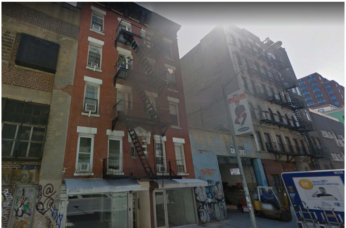
Photograph 16: Buildings on east side of Thompson Street north of Grand Street dating to the 1910s and 1920s, facing southeast from Thompson Street.
