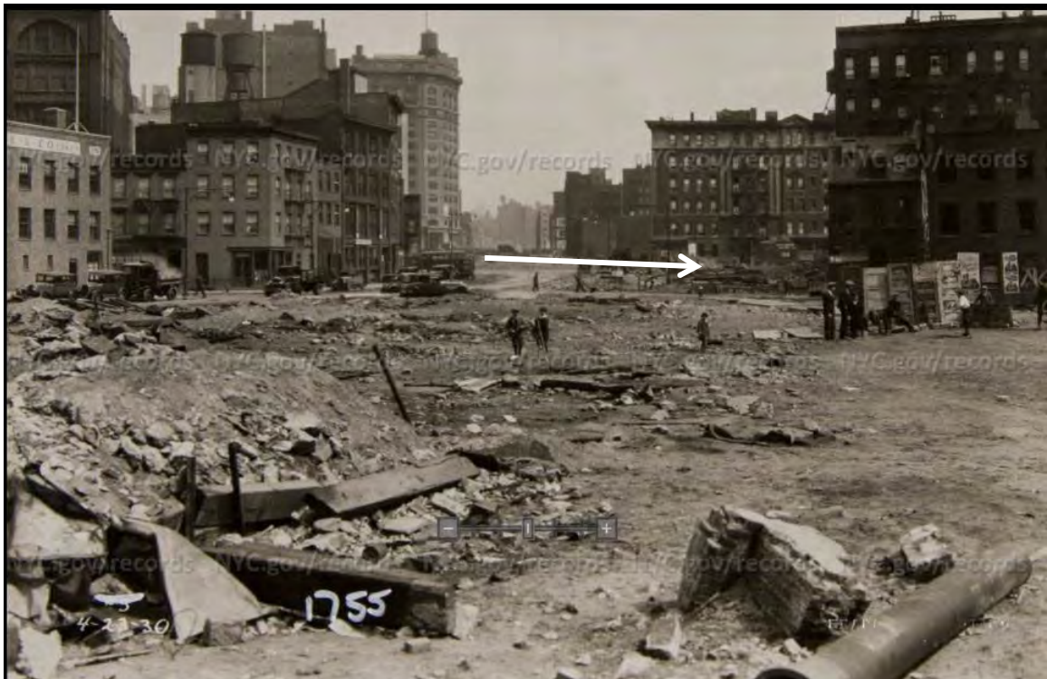
Figure 16. Looking north from Canal Street to route of Sixth Avenue Extension demolition. Arrow points to Block 227, Option 1 APE. New York City Municipal Archives.
