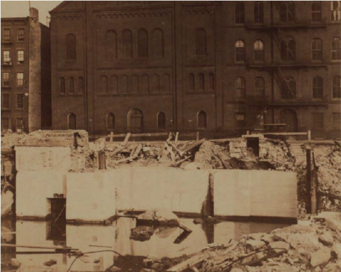
Figure 19. Close up of Block 227 Lots 62, 61, 60, and 59 (Option 1 Archaeological Area of Potential Effect) during construction of the Sixth Avenue Extension and the Eighth Avenue Subway. Photograph is facing east toward Option 1 APE, with Option 2 Archaeological Area of Potential Effect in Thompson Street to the east (between lots and Church). Note the car traveling or parked on Thompson Street, and standing water in front of the retaining walls that were presumably installed to stabilize demolition debris (Sperr, September 9, 1927).
