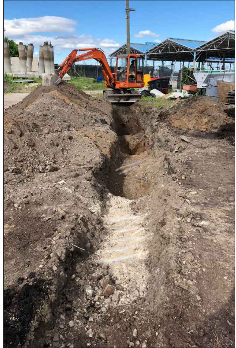
View of Trench 1 after excavation, showing two sets of utilities in foreground and brick footer in background 2
