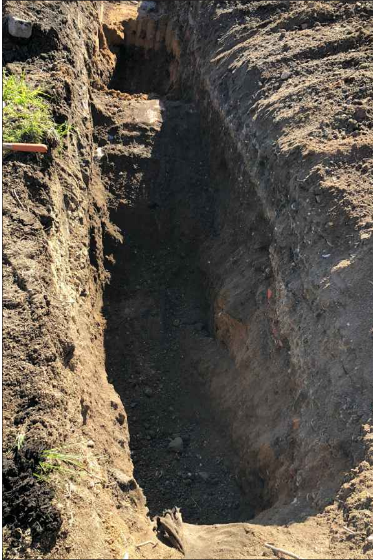
Looking northeast at Trench 1, showing sandy fill in foreground and utility lines in background 3
