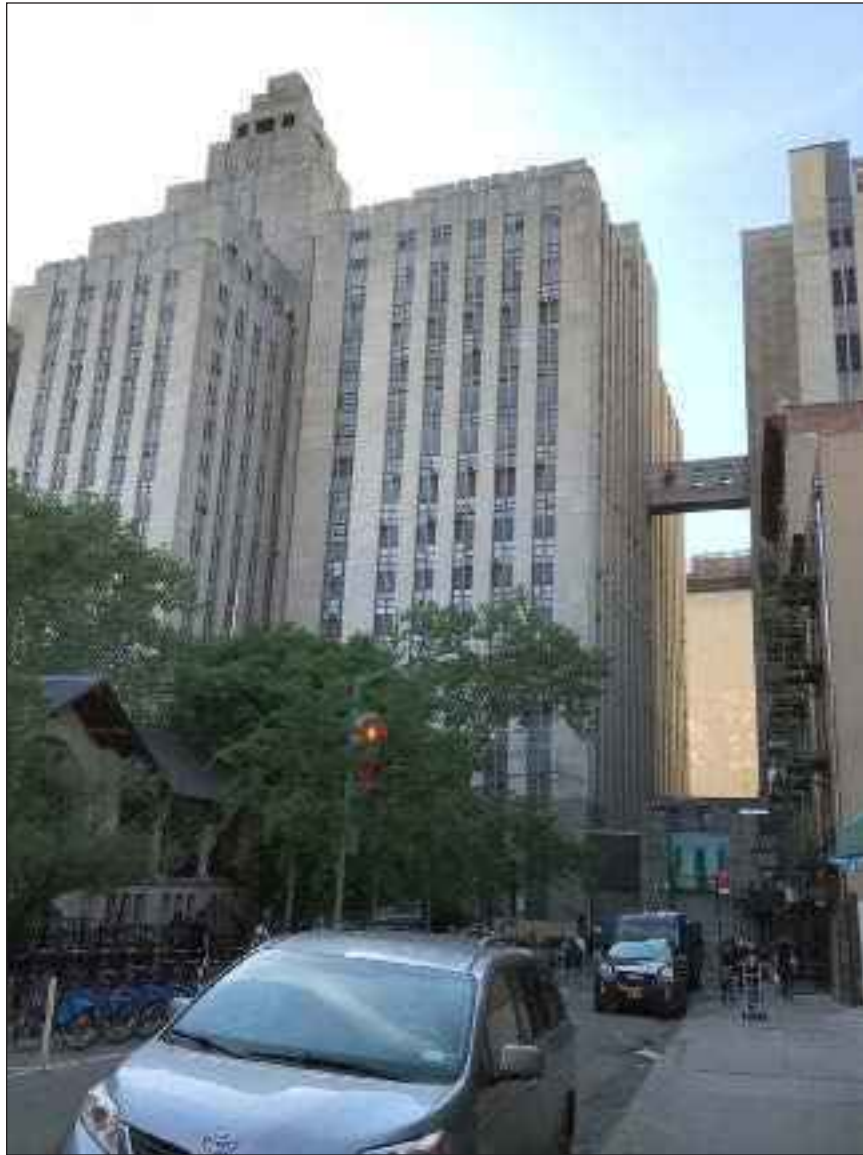
View west at the court building (at left) and the prison at 125 White Street (at right) from Bayard Street, showing the connections between the two buildings 5
