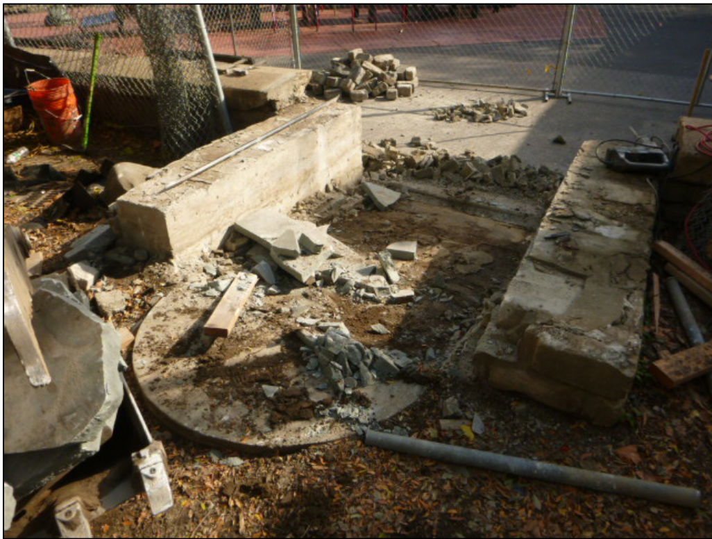
Image 06: Bluestone slab removal, looking south.
