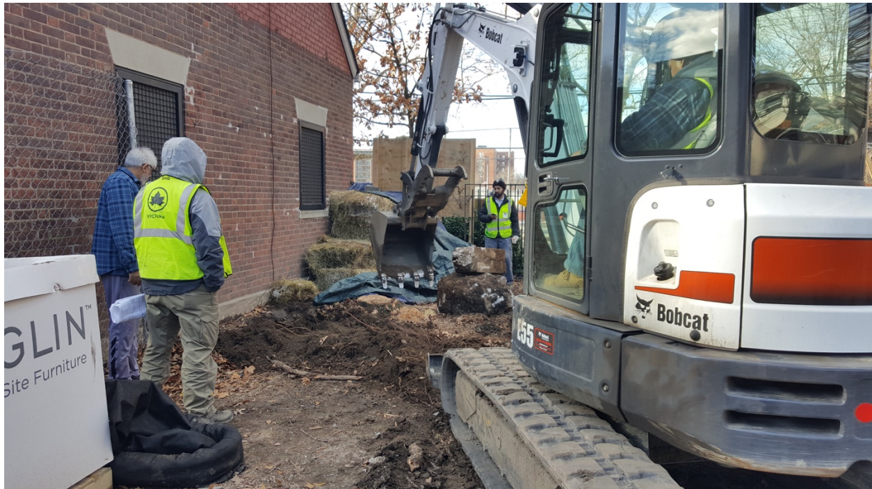
Image 17: Pit 2 excavation in progress.
