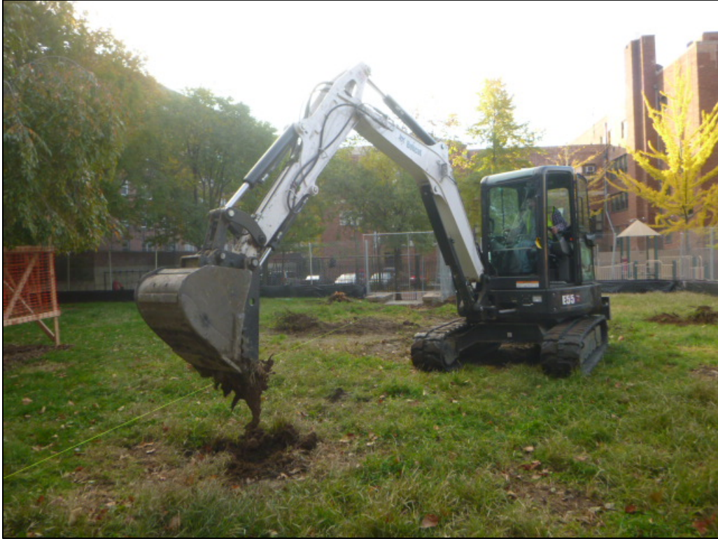
Image 26: Tree removal, Zone 2, looking south.
