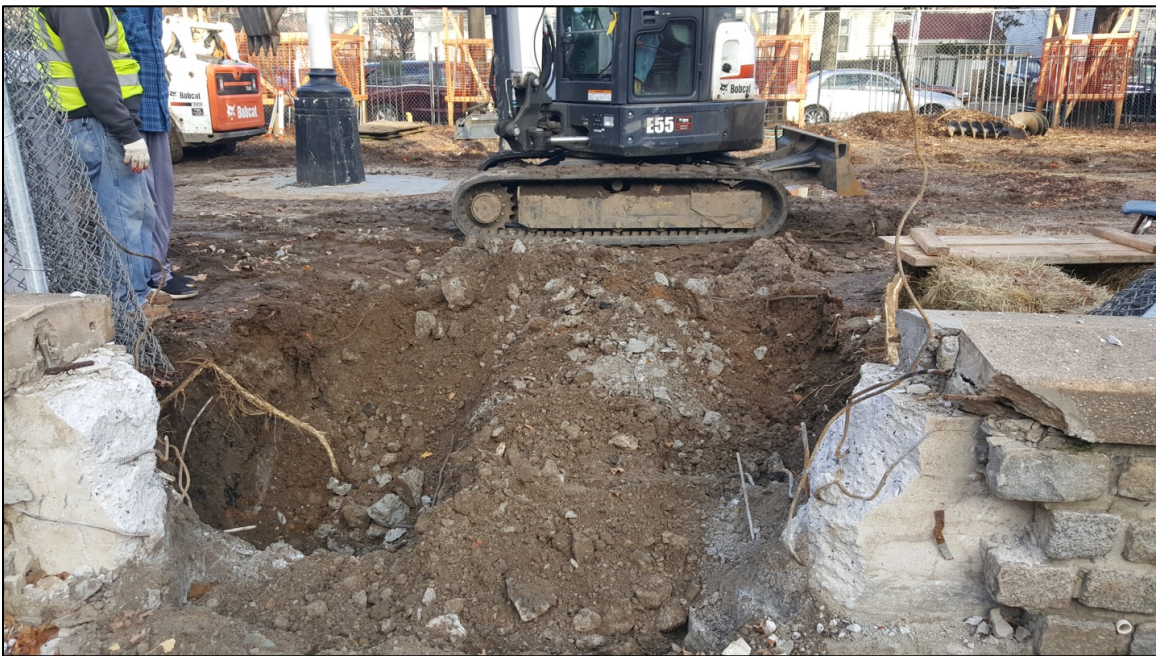
Image 16: Pit 1 excavation in progress.
