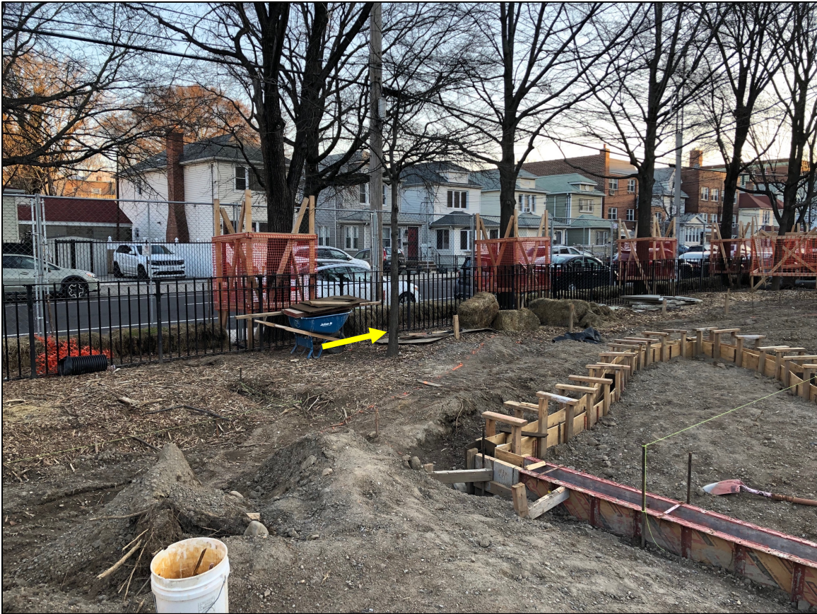
Image 24: Area overview of March tree removal, looking northeast.
