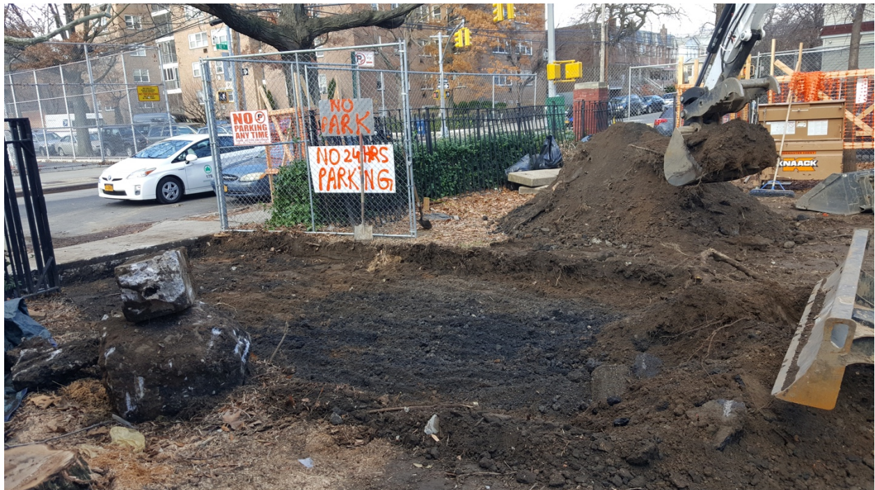
Image 15: Mass excavation in progress at 92 nd Street gate.
