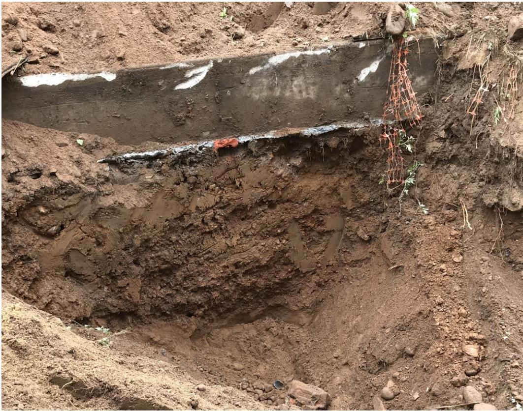
Photograph 9. Section of the Concrete Pathway and Drain Cover Exposed at the West End of the North Wall.
