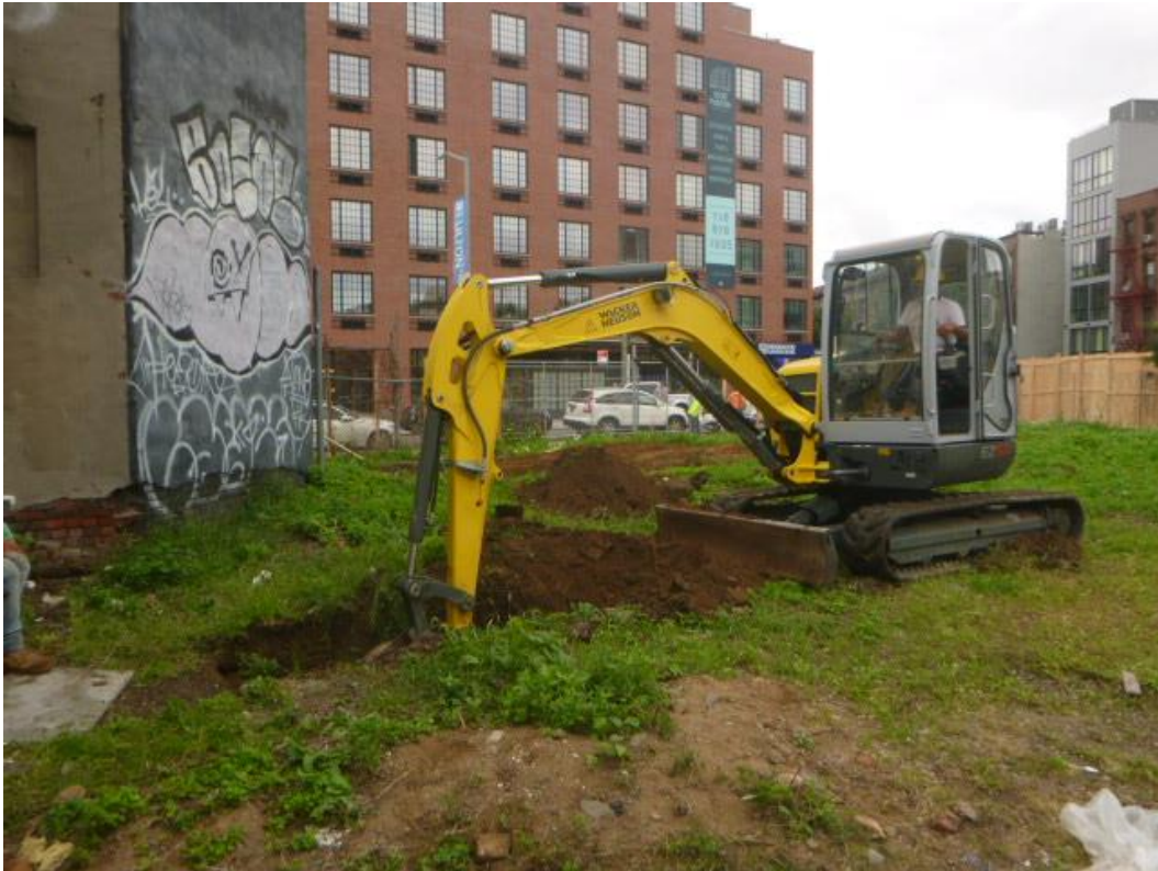
Image 04: Excavation in progress, Trench 02 (looking east).
