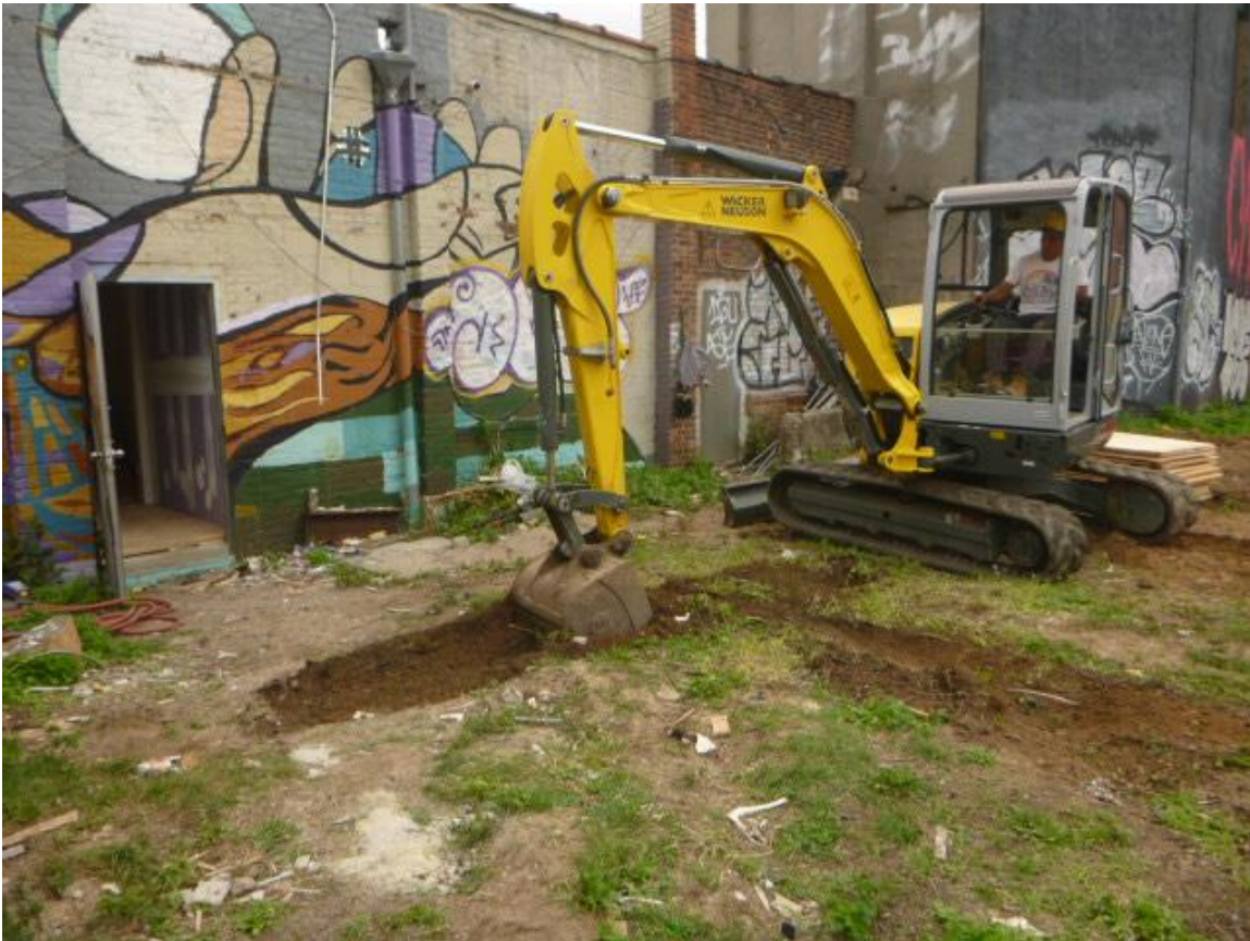
Image 17: Location of Trench 03, excavation in progress (looking north).
