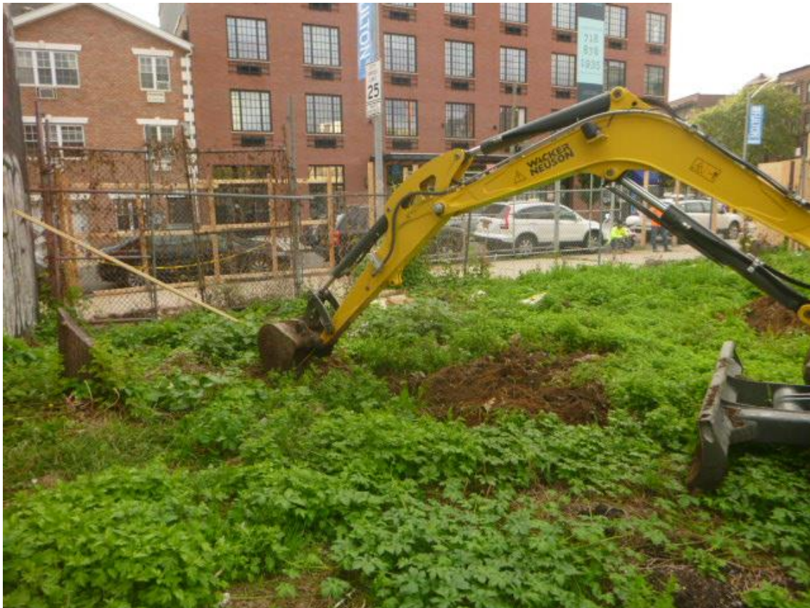
Image 01: Location of Trench 01 (looking east).
