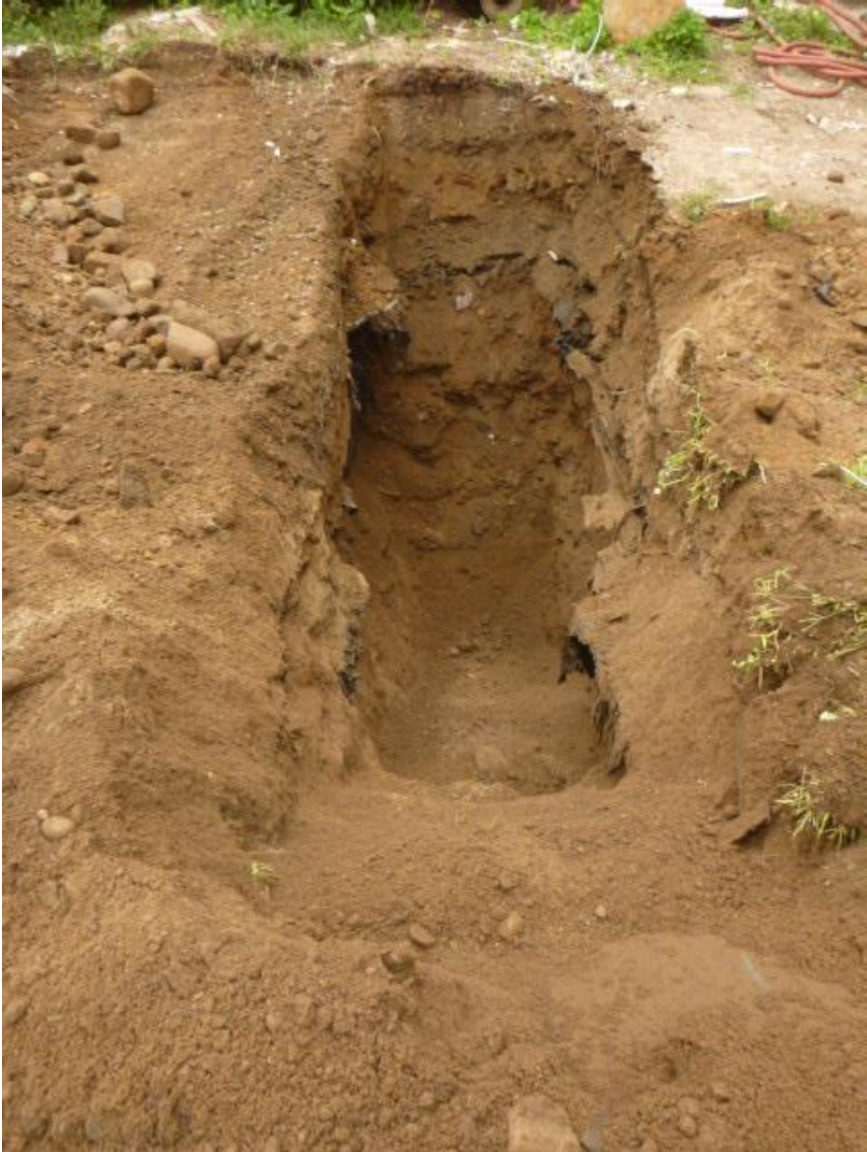
Image 19: Trench 04, post-excavation (looking west).
