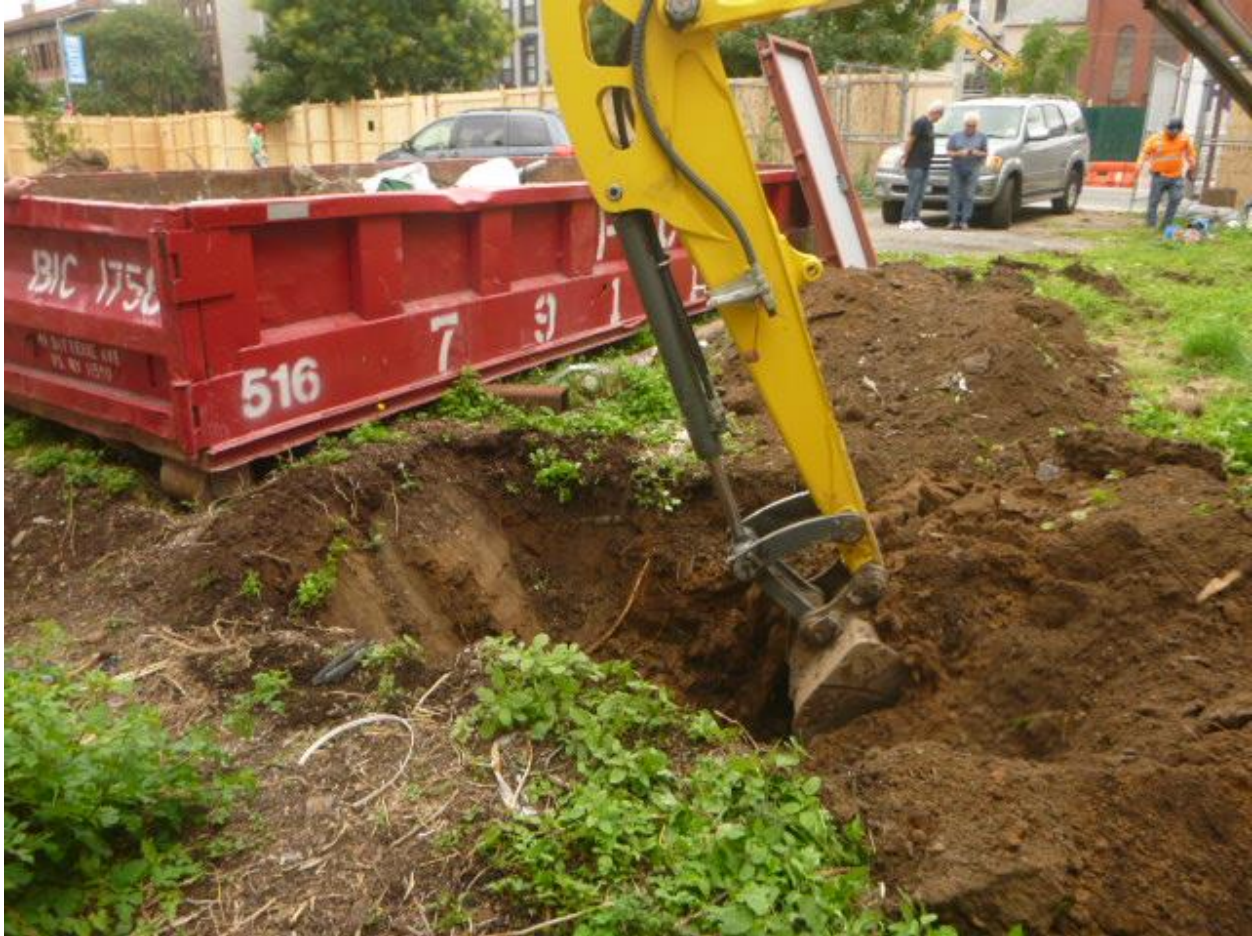
Image 22: Trench 05, excavation in progress (looking south).
