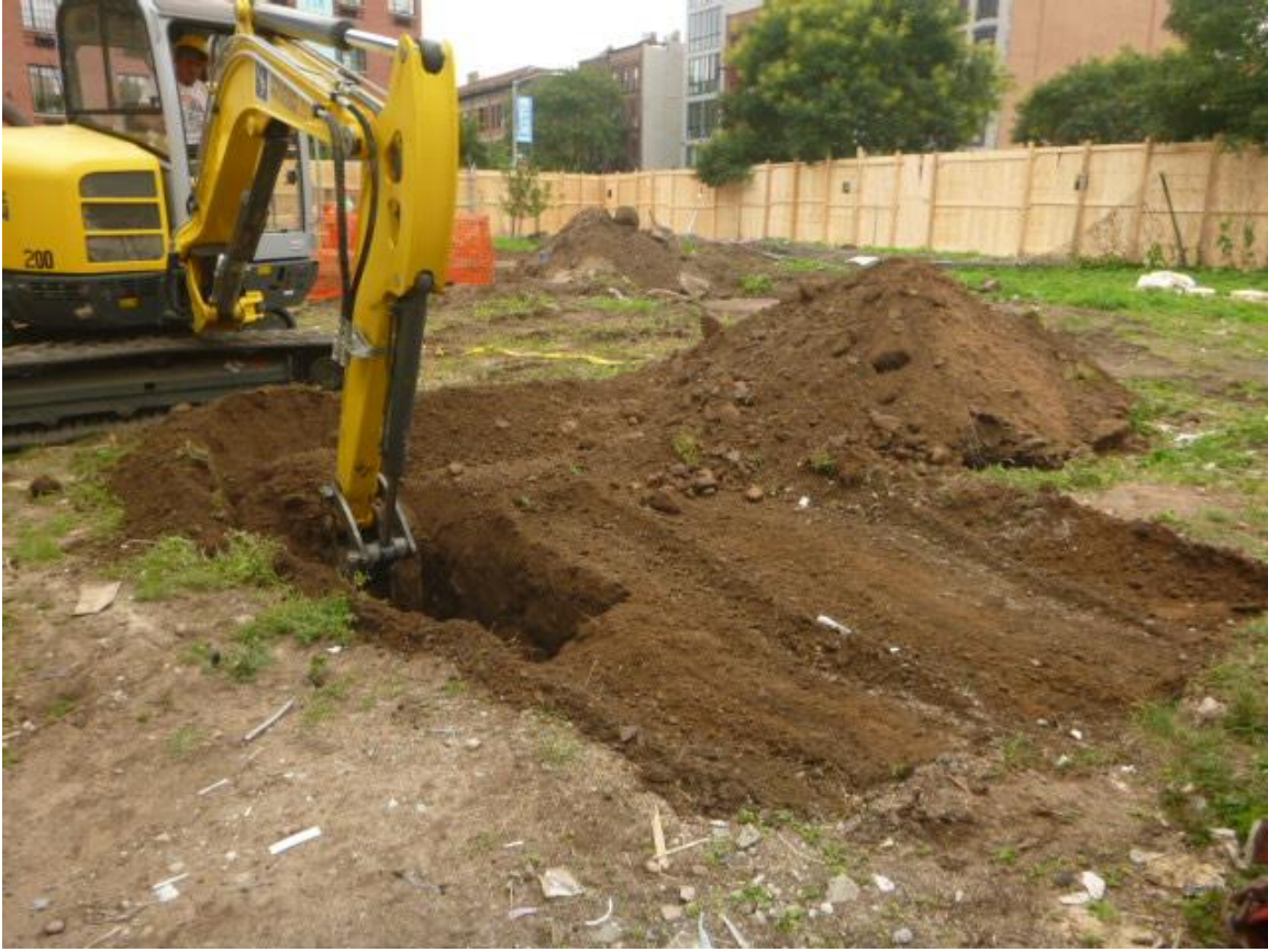
Image 18: Compact gravel layer impacting the excavation of Trench 04 (looking southeast).
