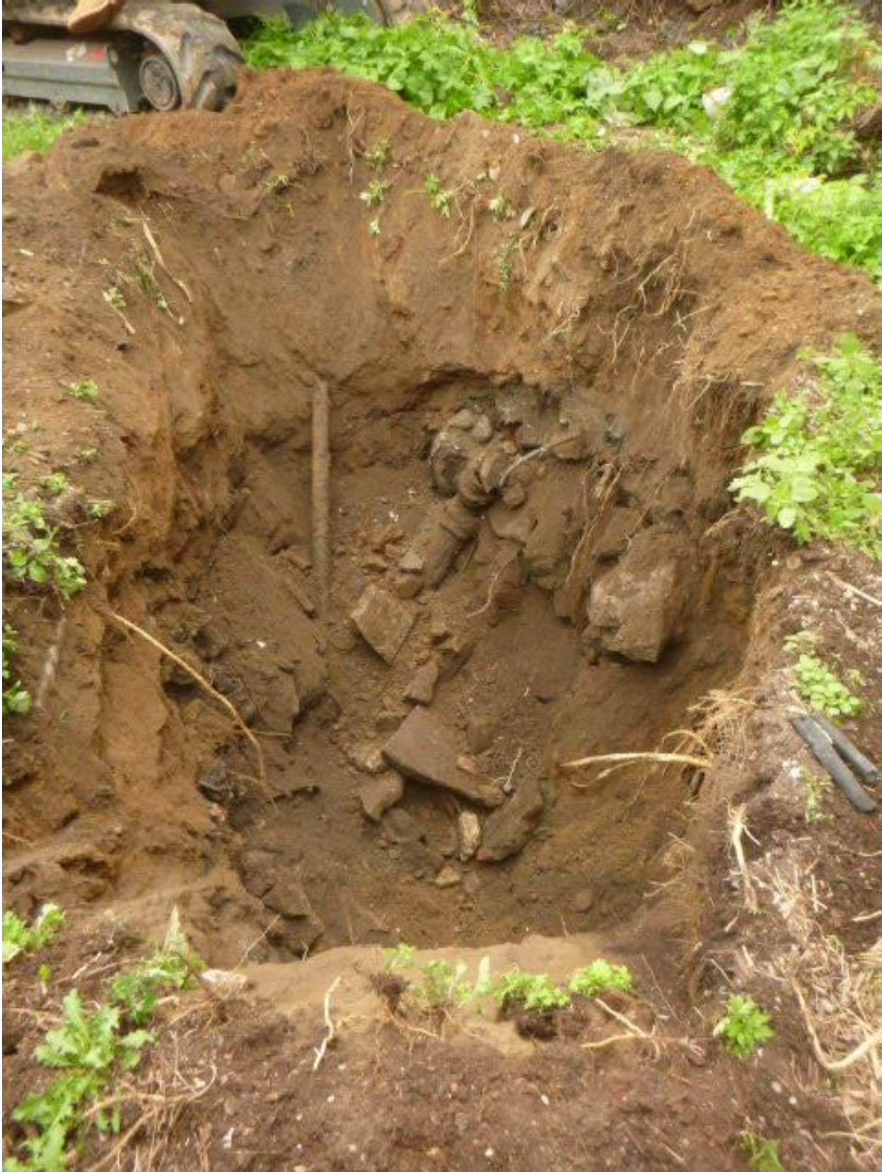
Image 24: Concentration of demolition materials in Trench 05.
