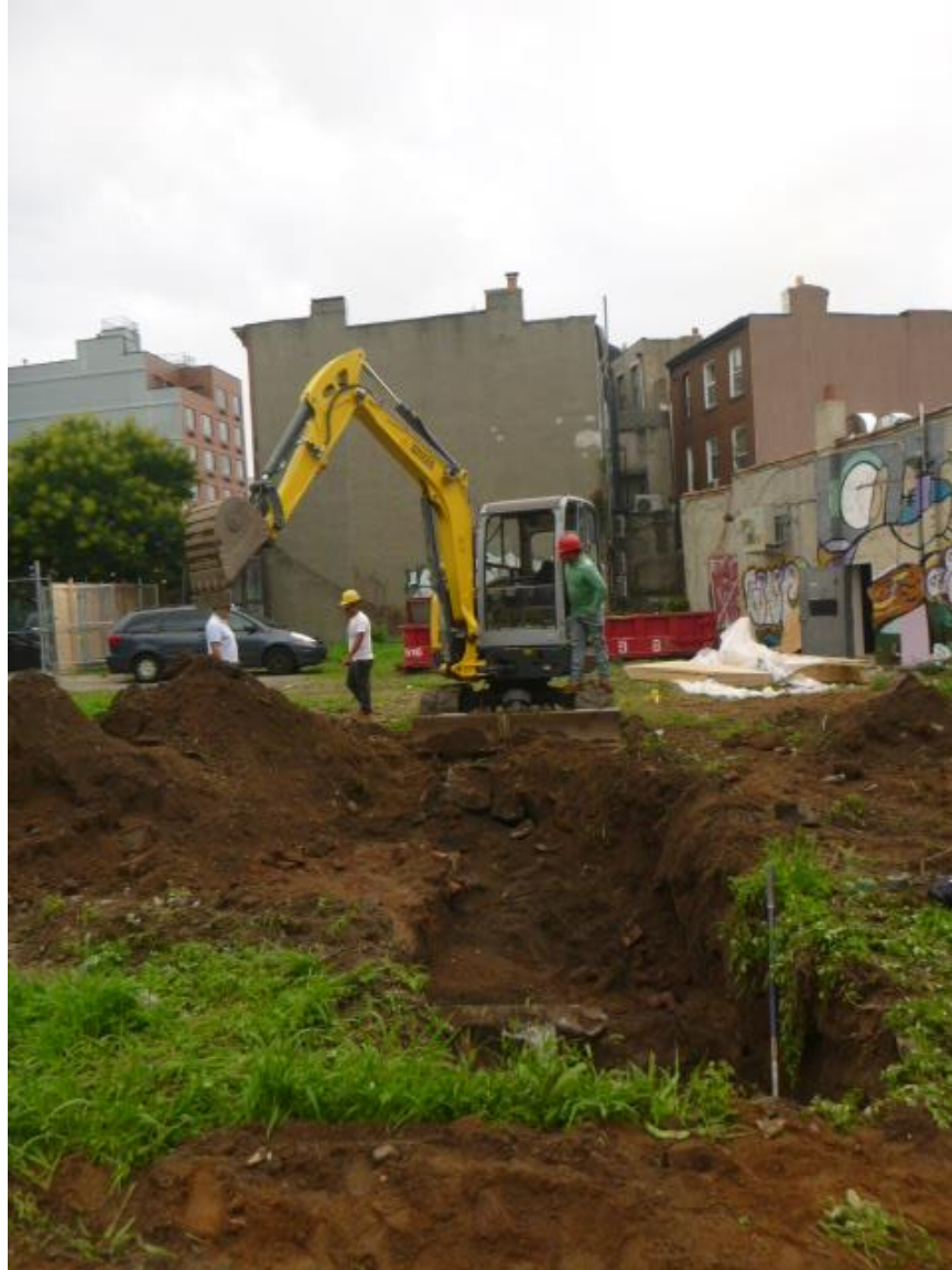
Image 07: Dimensions of Trench 03 (looking west).
