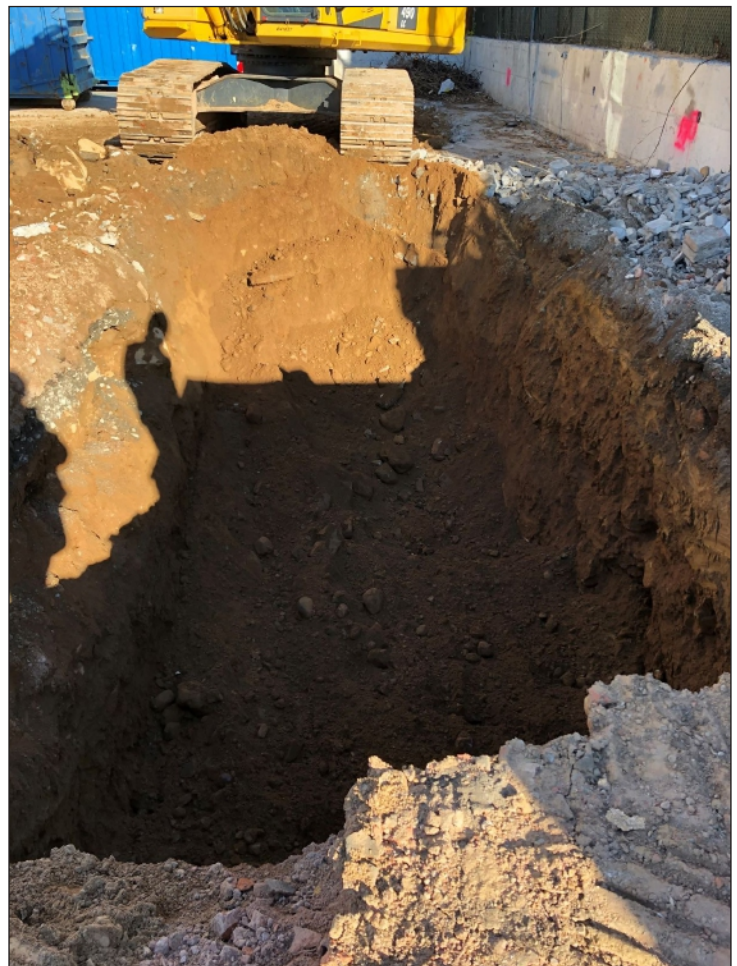
Looking north at Trench 2, excavated to a depth of nine feet 2
