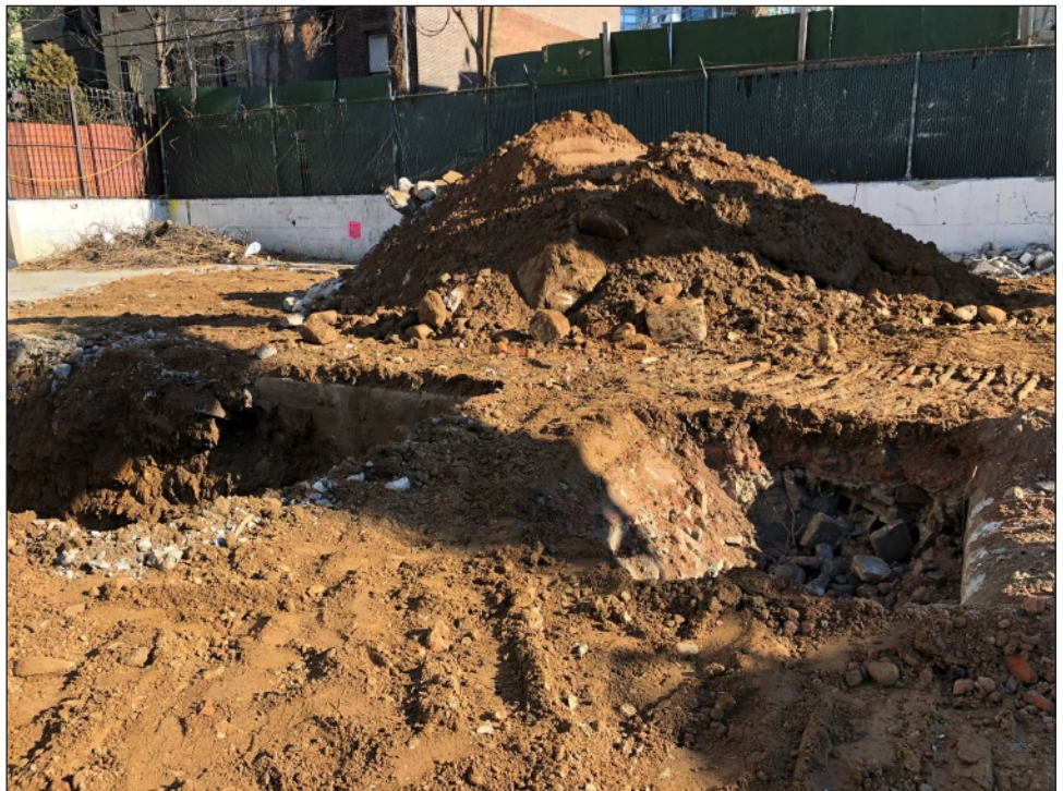
Looking east at the southern end of Trench 3 (left) and the abandoned Trench 4 (right) 4
