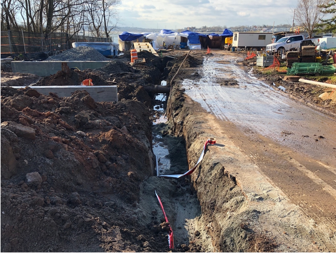
Image 43: Trench 11, overview, looking west.
