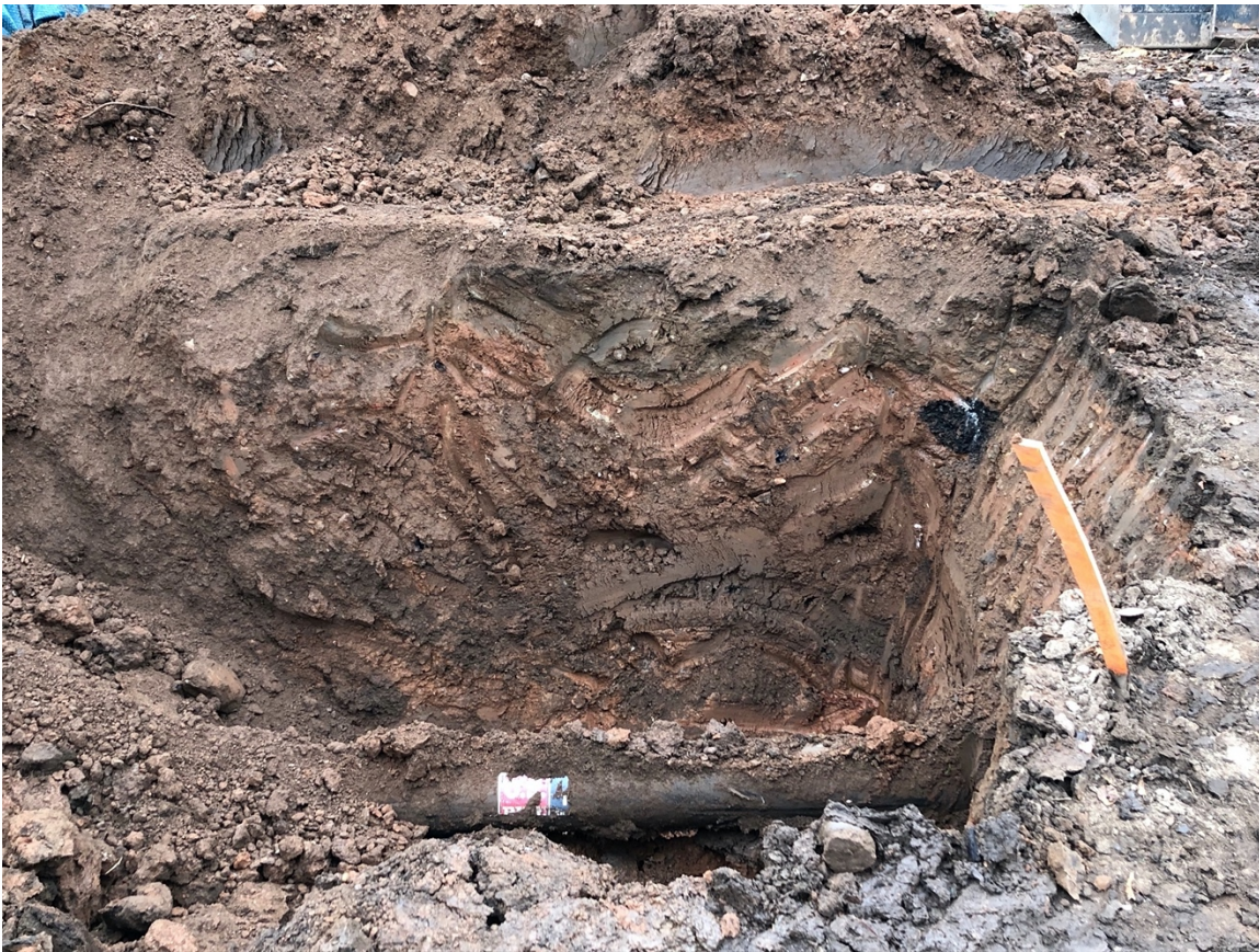
Image 51: North wall profile, Trench 14.
