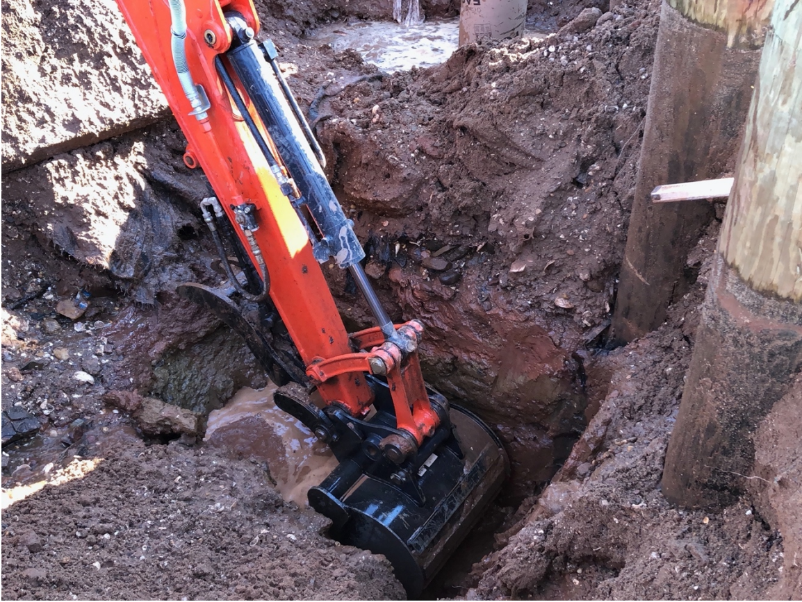
Image 75: Trench 25, excavation-in-progress, looking east.
