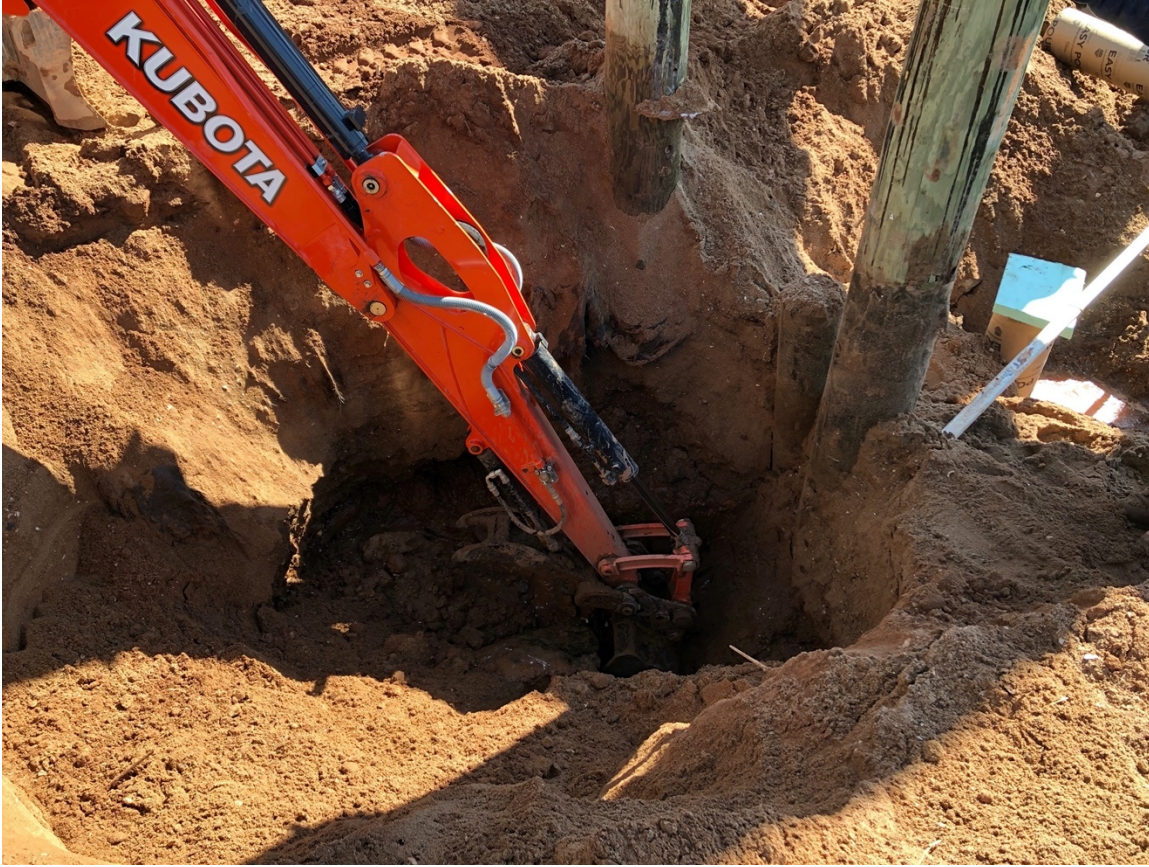
Image 77: Trench 28, excavation-in-progress, looking south.
