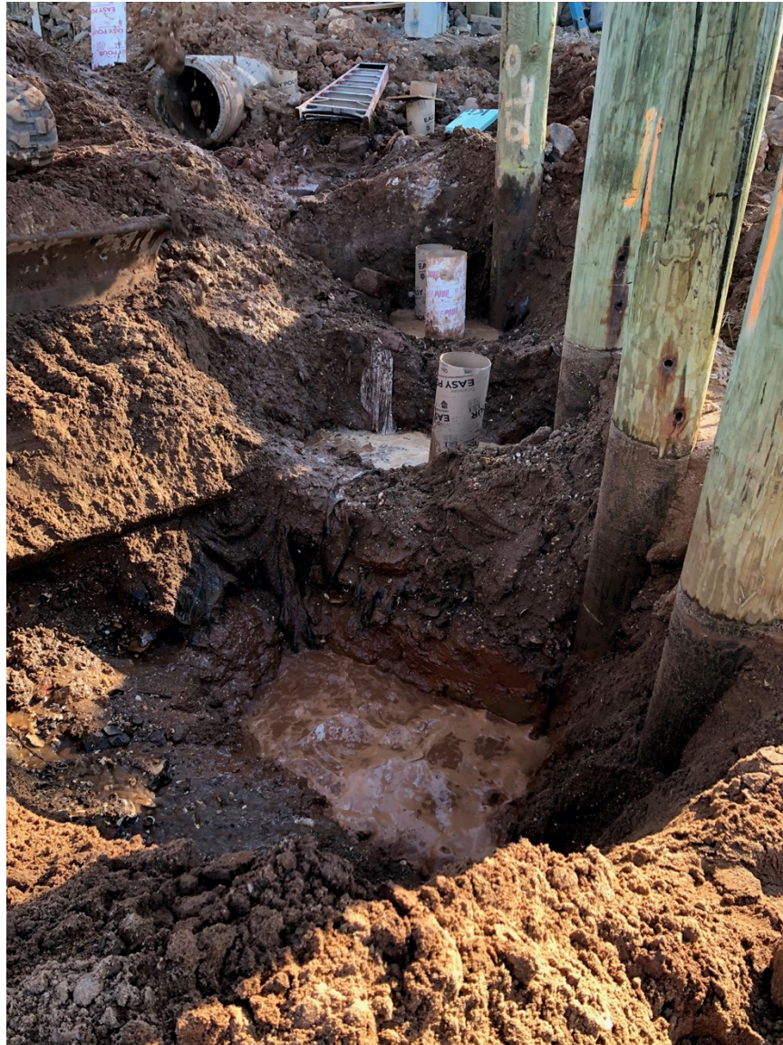
Image 69: Trenches 23-25, along the southernmost line of east-west oriented main wooden support beams.
