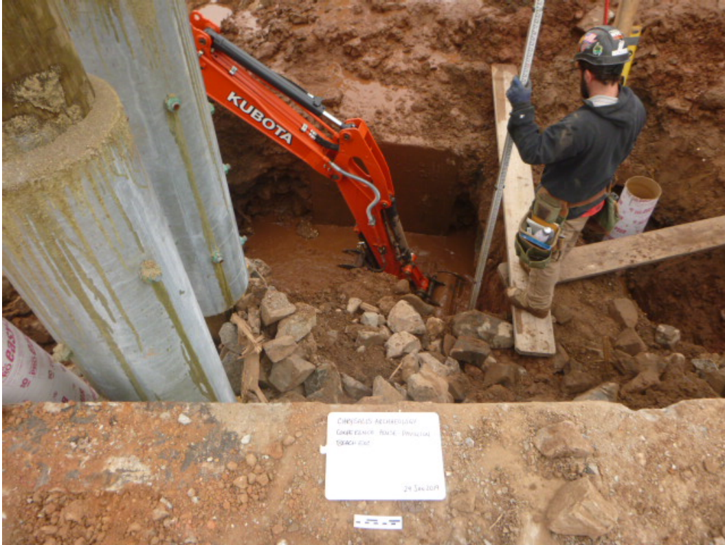
Image 59: Trench 17, excavation in progress.
