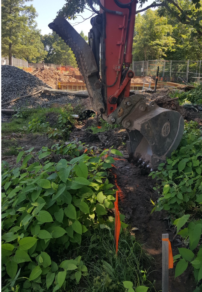
Image 29: Location of TP 3, looking east.
