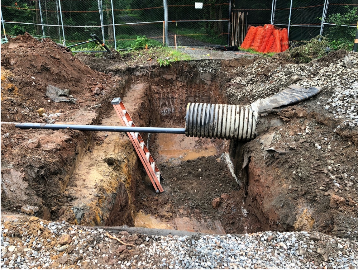
Image 19: Trench 04 post excavation, looking south.
