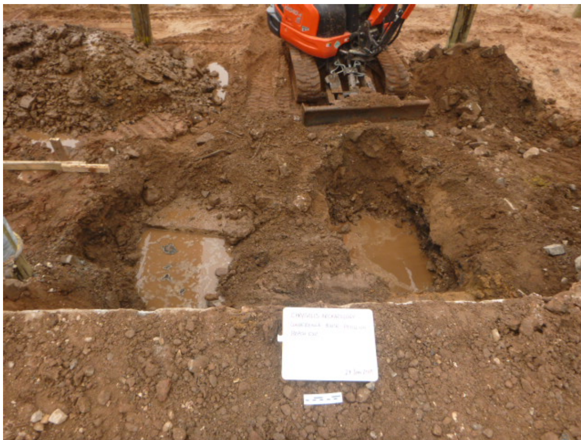
Image 61: High water table in Trenches 19 and 20.
