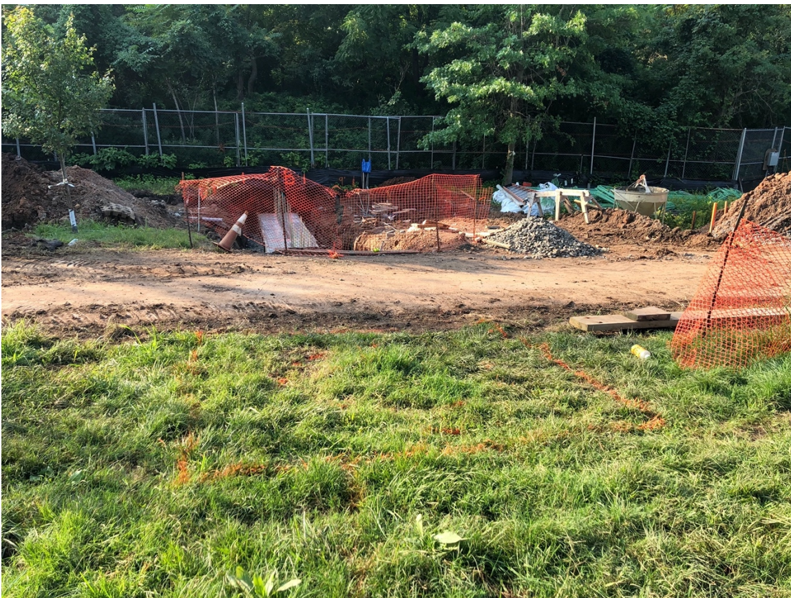
Image 25: Catch Basin 1/TP 1 pre-excavation, looking south with Trench 05 in background.
