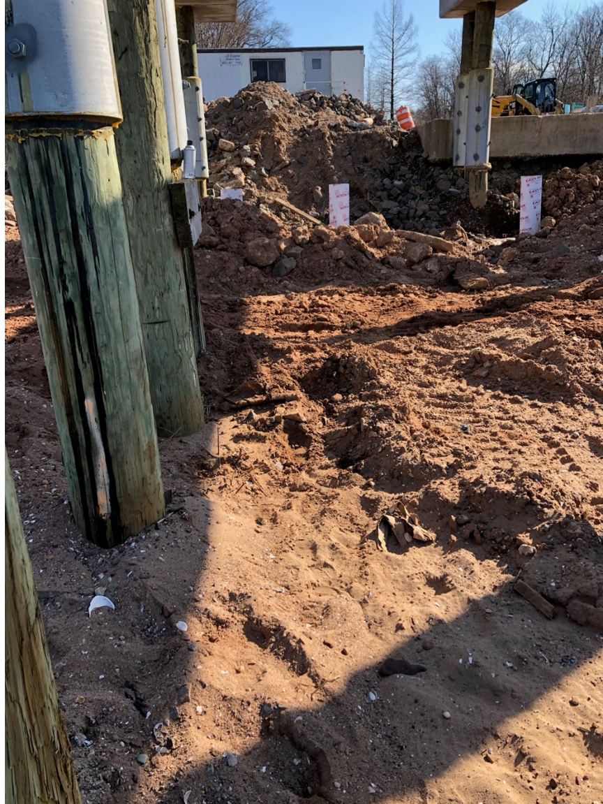
Image 71: Unexcavated area due to concrete flooring.
