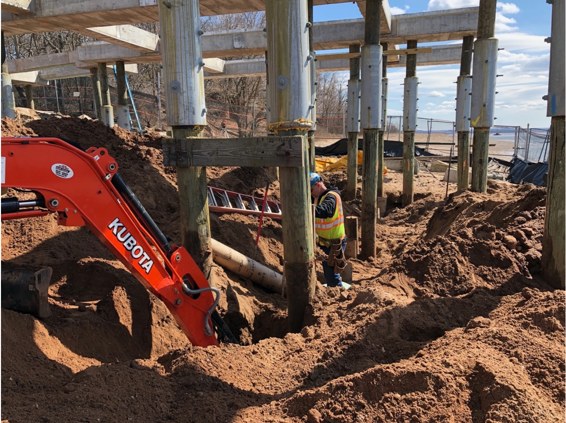
Image 70: Trenches 26-31, running south to north along the western edge of the main support beams.
