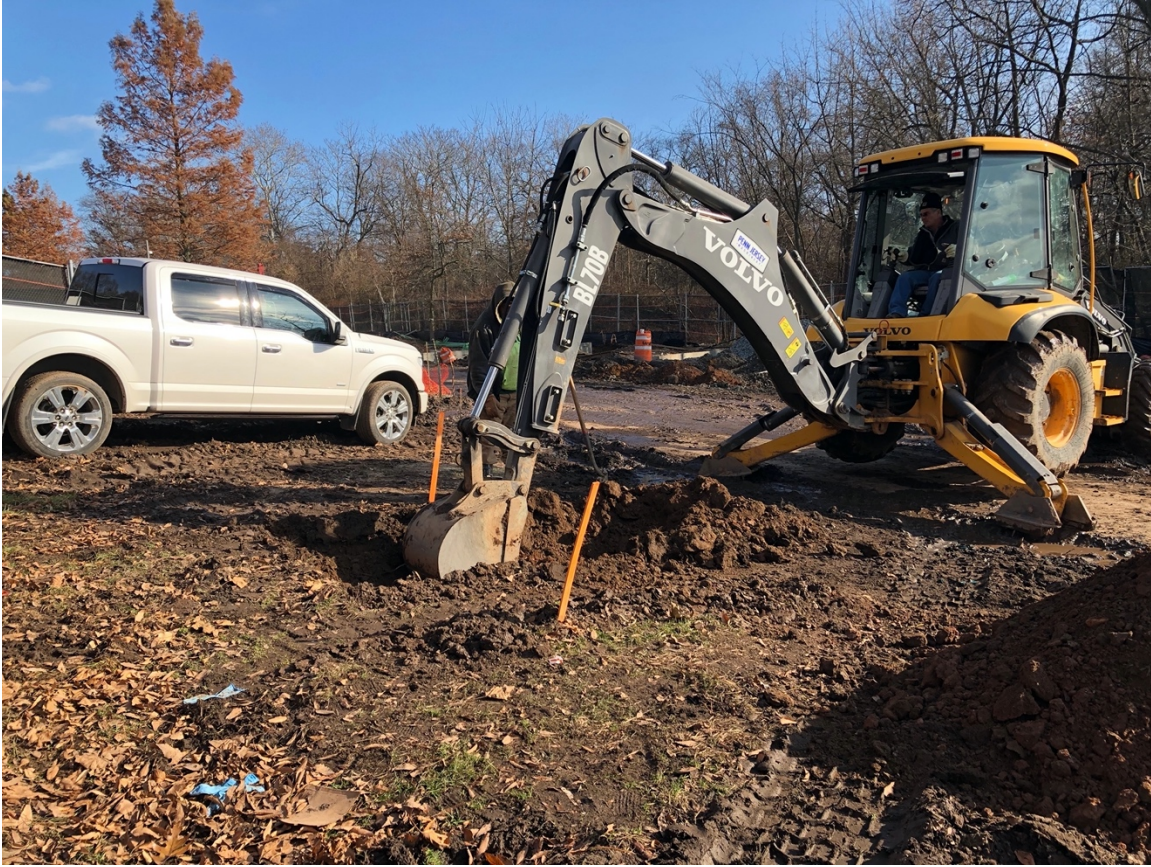
Image 45: Trench 12, excavation in progress, looking southeast.
