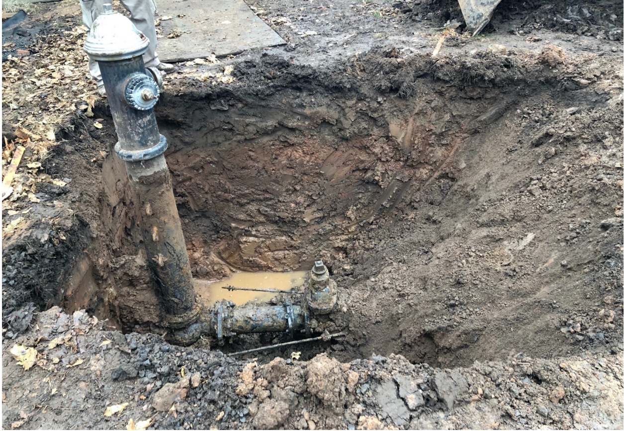
Image 48: Fire hydrant elements exposed, Trench 13.
