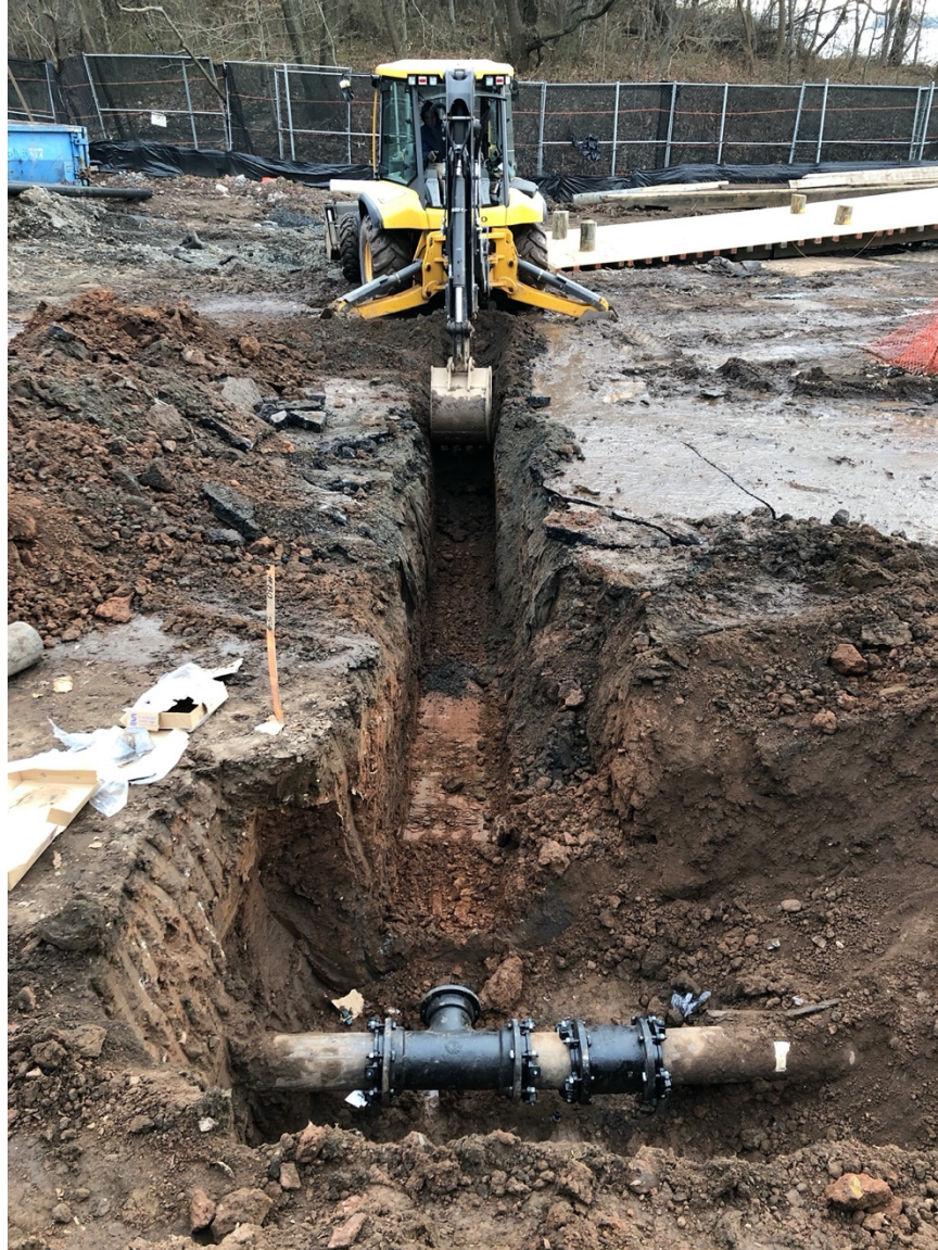
Image 52: Trench 15, excavation in progress, looking south with Trench 14 in foreground.
