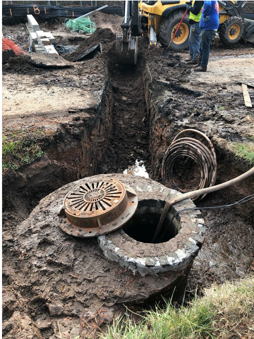
Image 41: Trench 10, excavation in progress, looking south.
