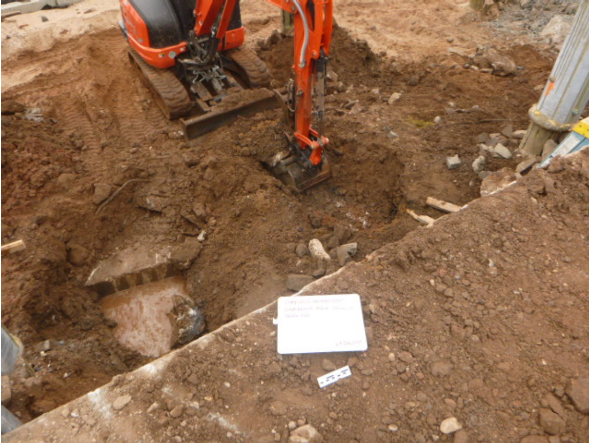
Image 64: Discovery of second concrete layer during excavation of Trench 20.
