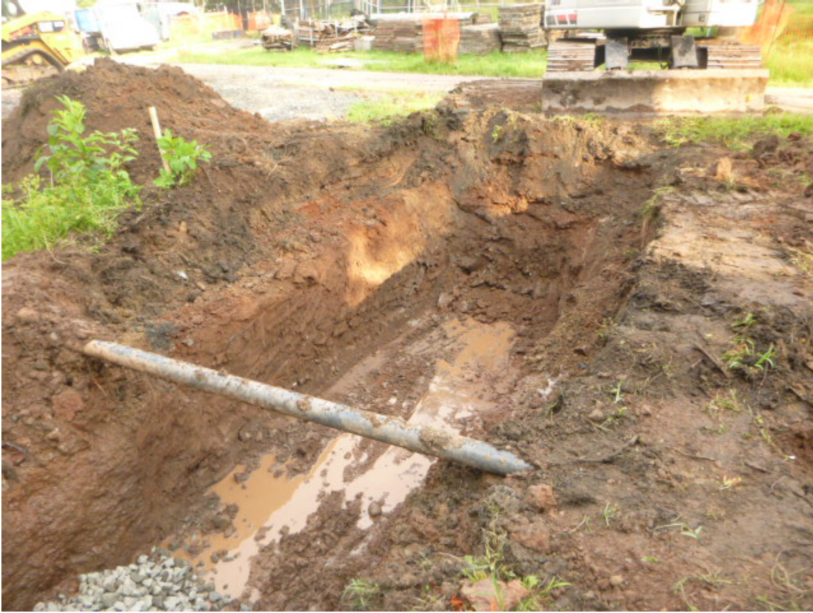
Image 18: Trench 03, post-excavation, looking north.
