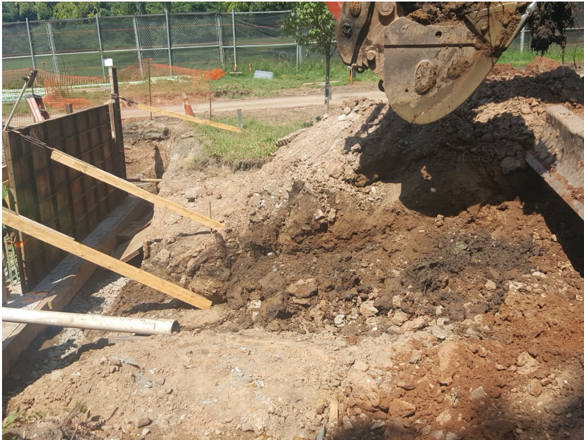
Image 22: Excavation-in-progress, Trench 09A, looking north.
