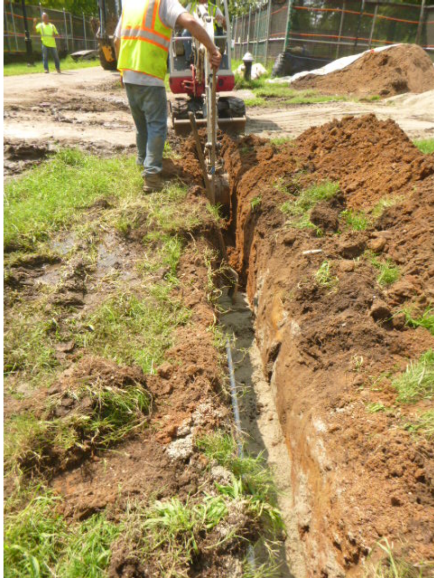
Image 13: Trench 02, excavation in progress to the west of Feature 01.
