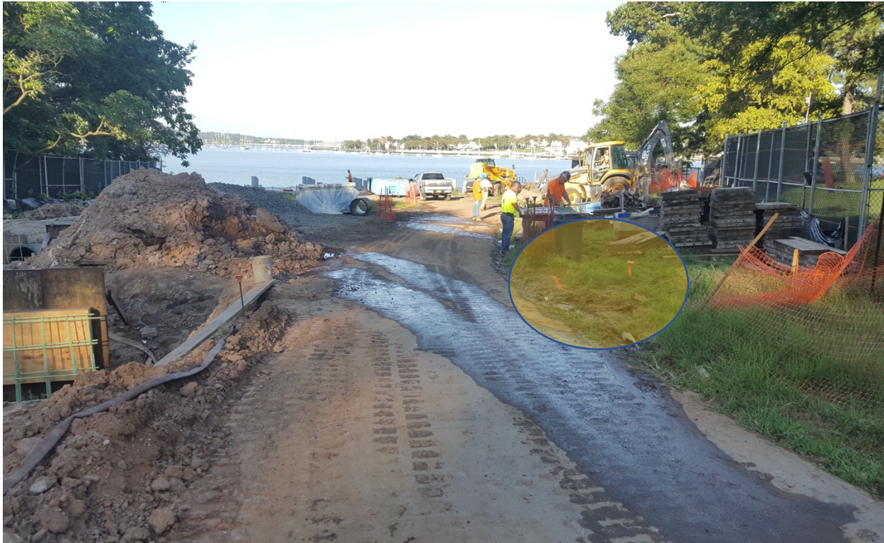
Image 27: Location of TP 2 (highlighted) with Trench 03 on left, looking west.
