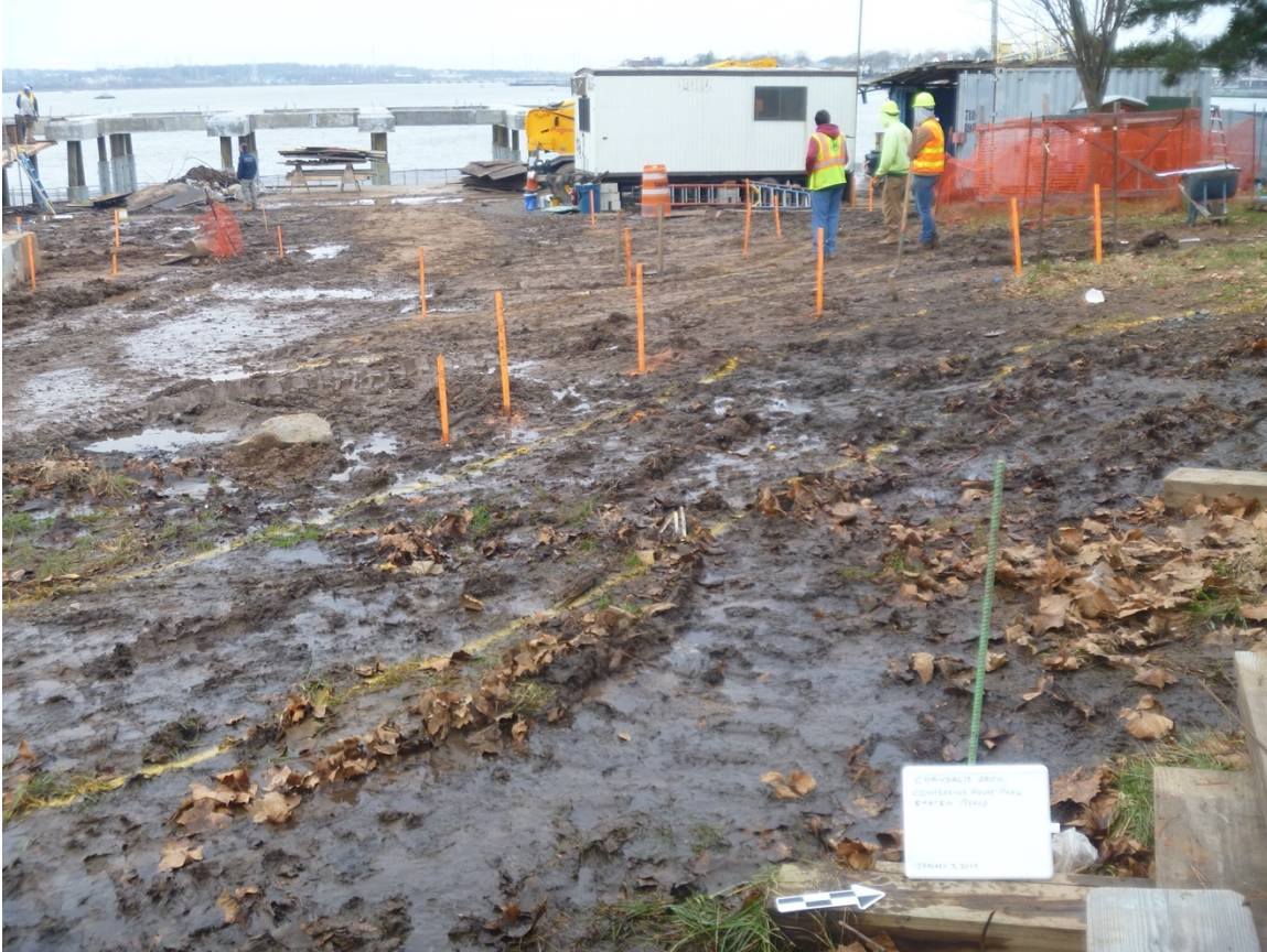
Image 80: Seawall locations laid out, looking west.
