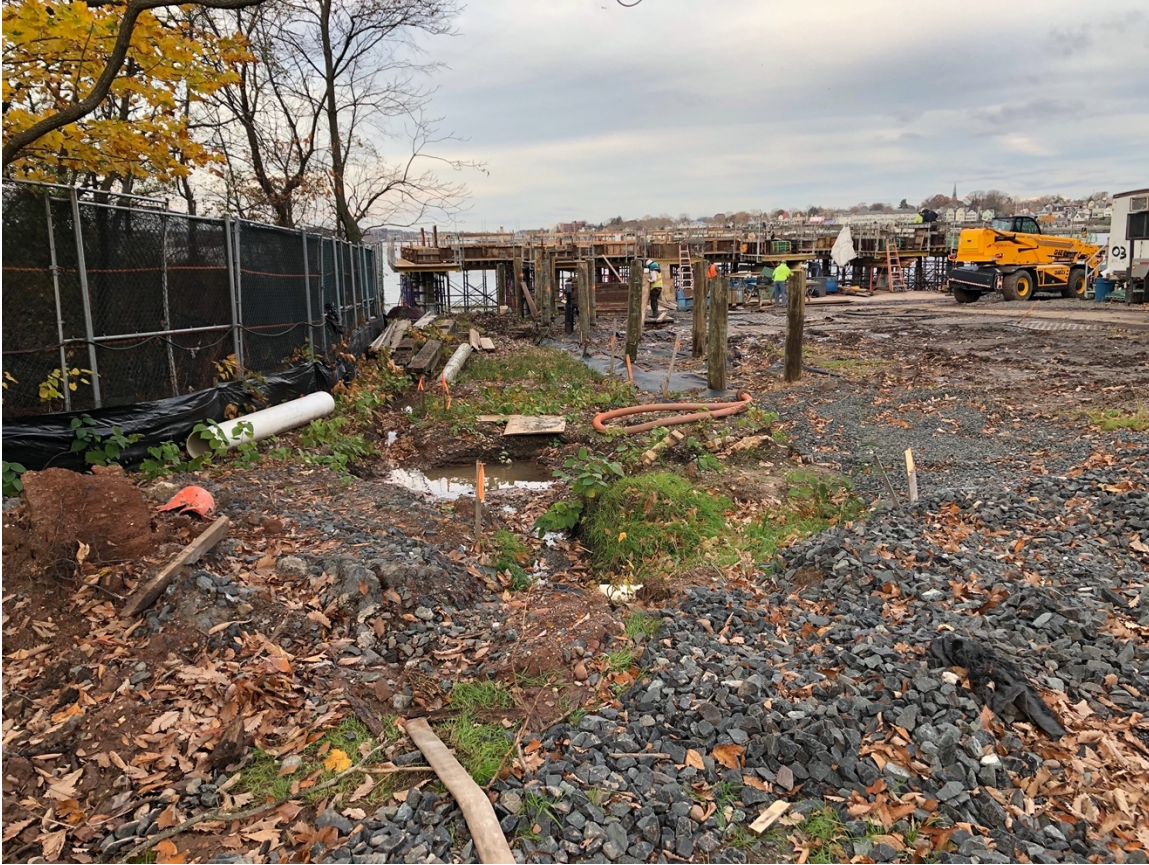
Image 34: Trench 07 pre-excavation, looking west.
