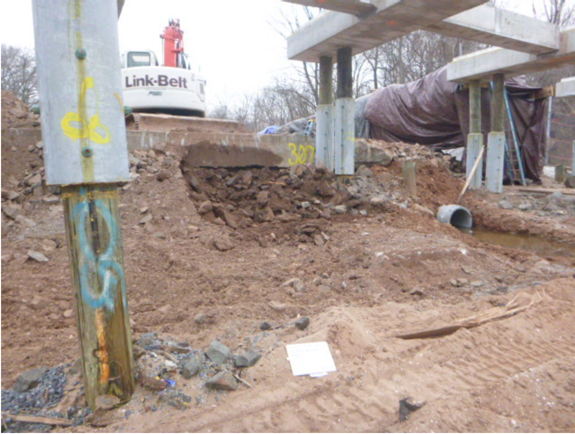
Image 56: Construction debris and fill removal, beach area.
