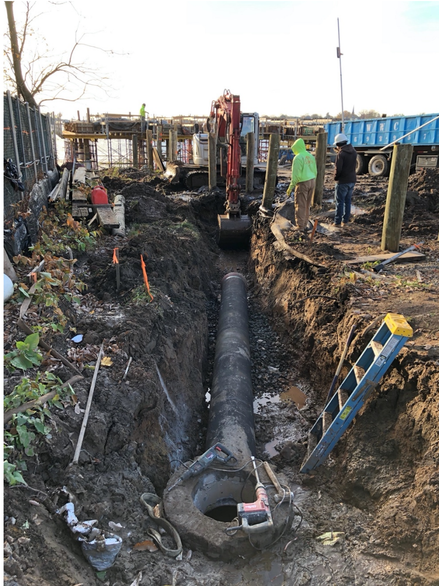
Image 35: Trench 07, excavation in progress, looking west.
