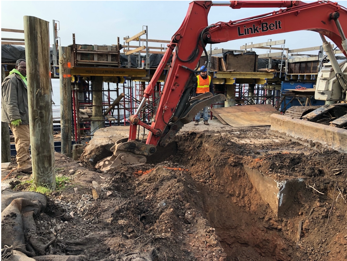
Image 37: TP 4, excavation in progress, looking west.
