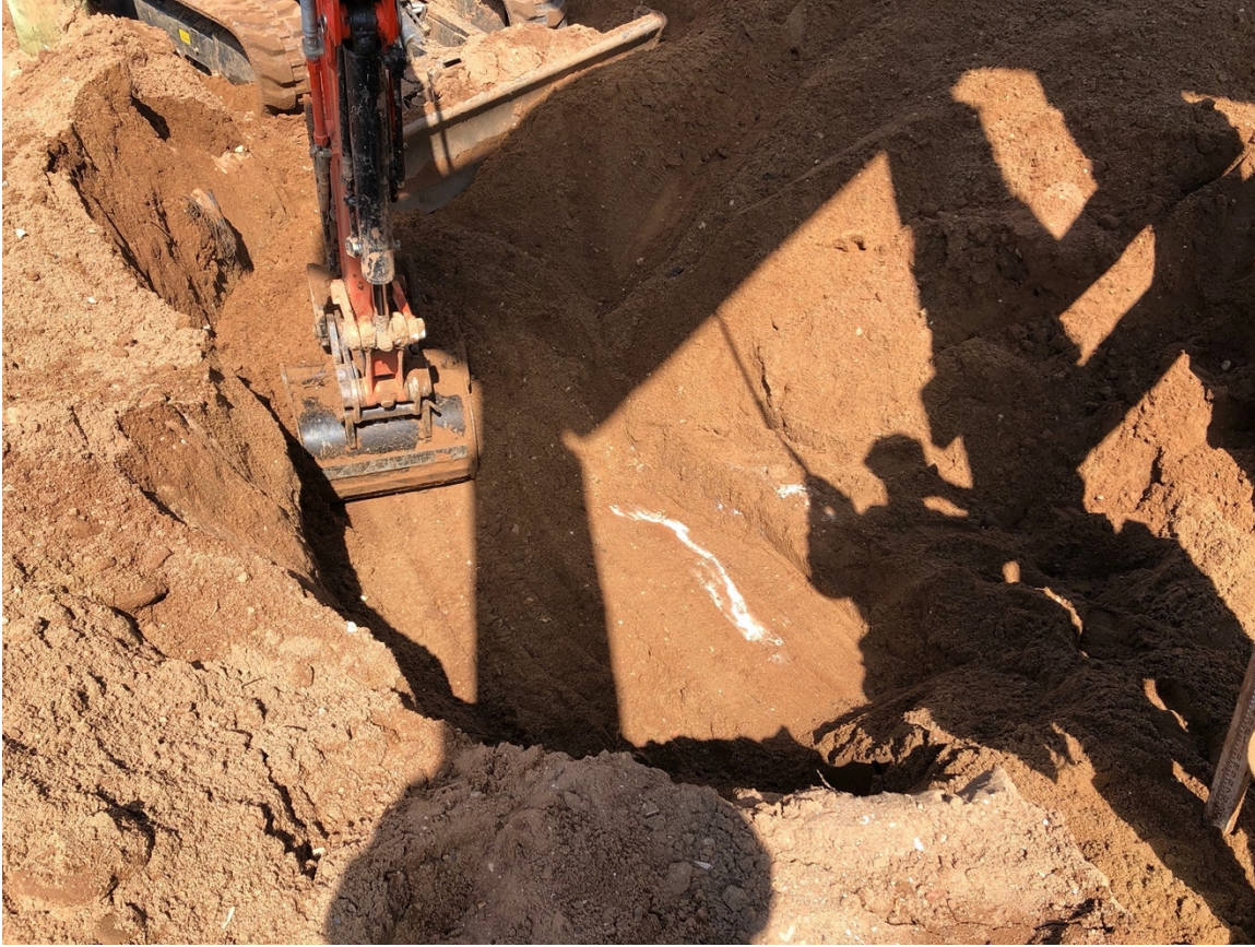
Image 79: Concrete flooring in Trench 31.
