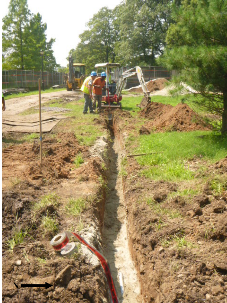
Image 09: Trench 02, Section 2, excavation in progress.
