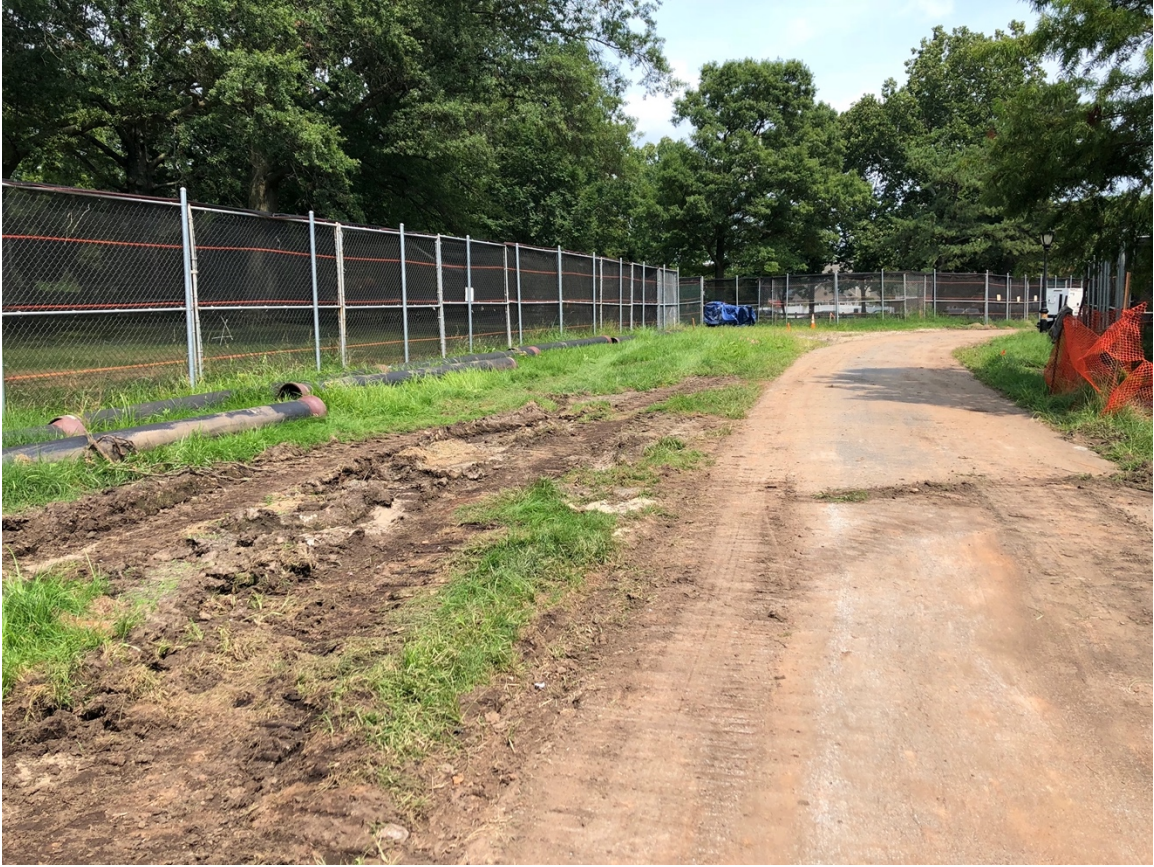
Image 31: Trench 06 pre-excavation, looking east.
