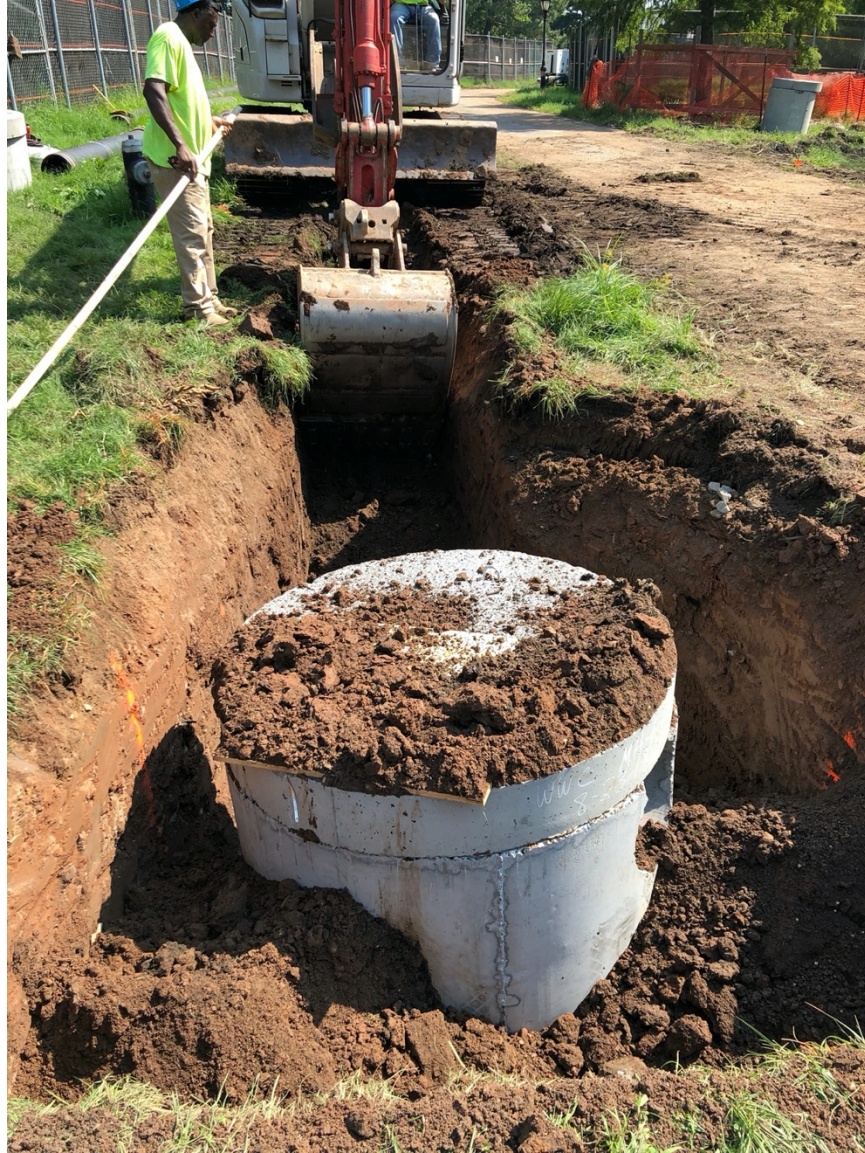
Image 32: Trench 06 excavation in progress, with Catch Basin 1 in foreground, looking east.
