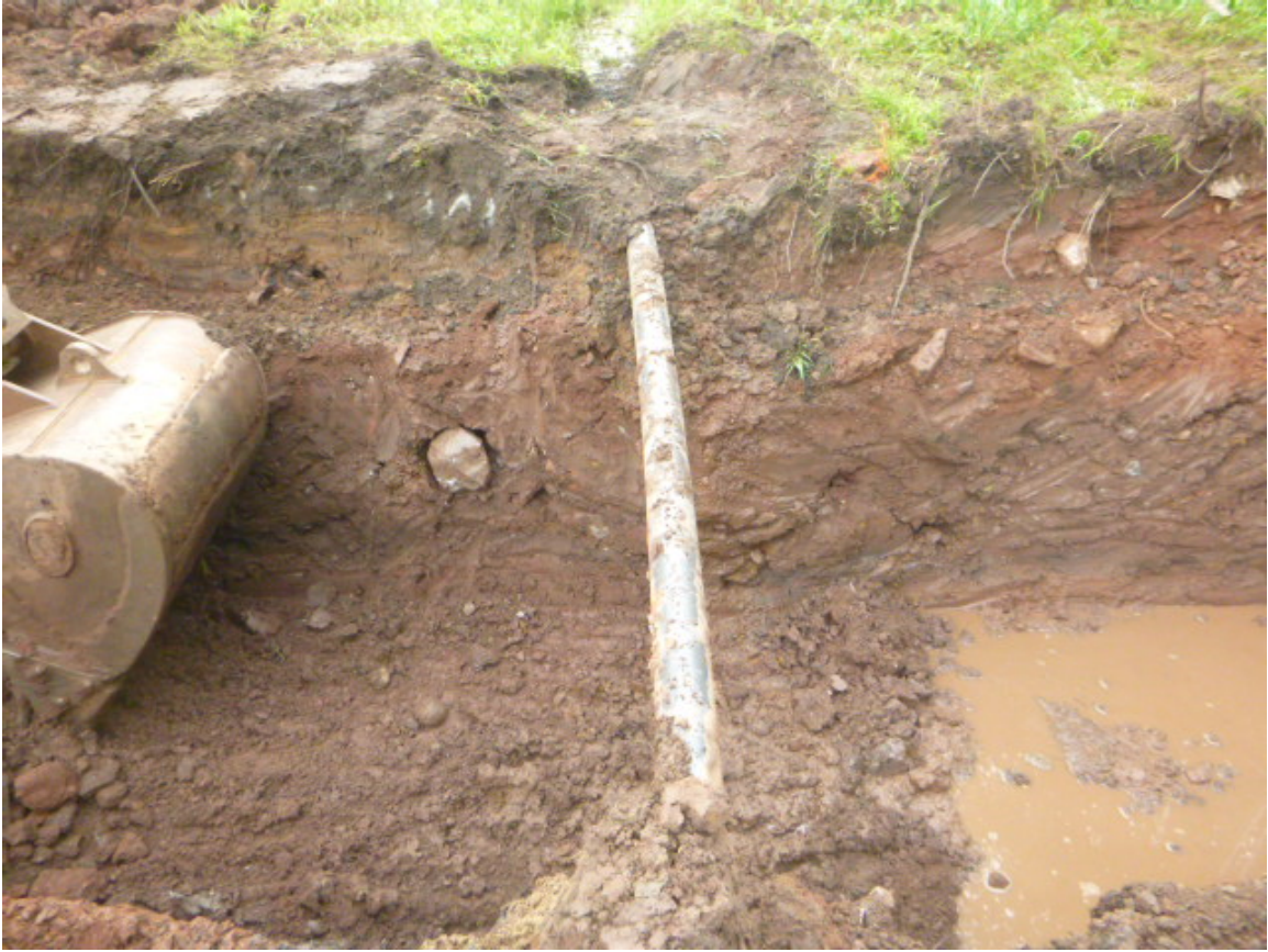
Image 17: Stratigraphic profile, west wall – Trench 03.
