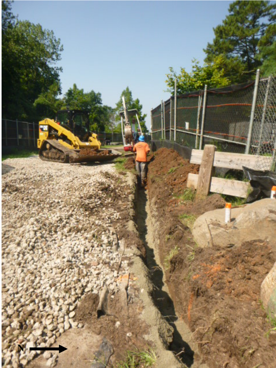
Image 07: Eastern section of Trench 02, excavation in progress.
