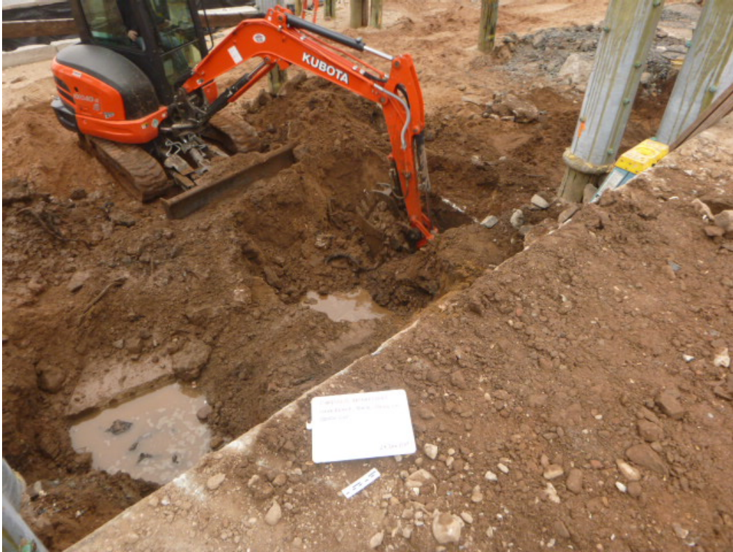
Image 65: Widening of Trench 20.
