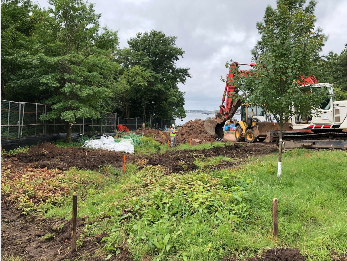
Image 15: Weir area pre-excavation, looking west.
