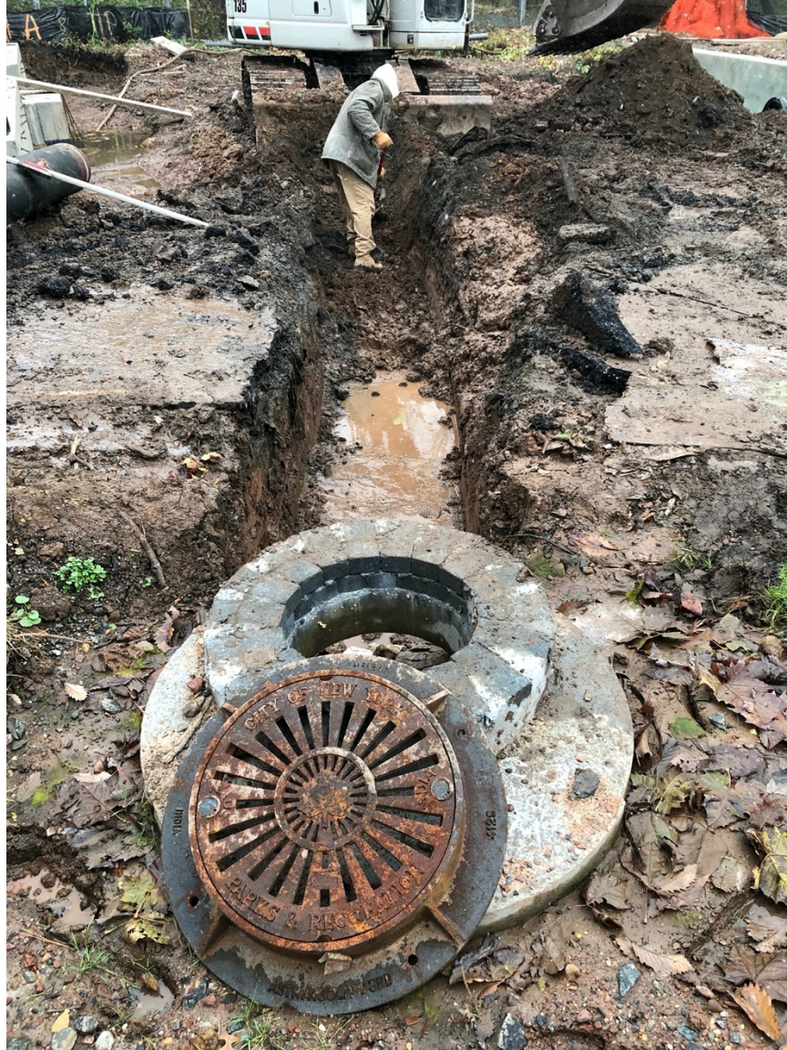
Image 39: Trench 08, excavation in progress, looking south.
