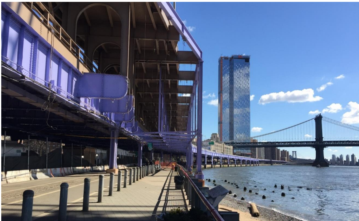
Photo 2: Looking north, on the East River Waterfront Esplanade that includes a bike path, seating areas and general open space, at the south end of the Project Area.
