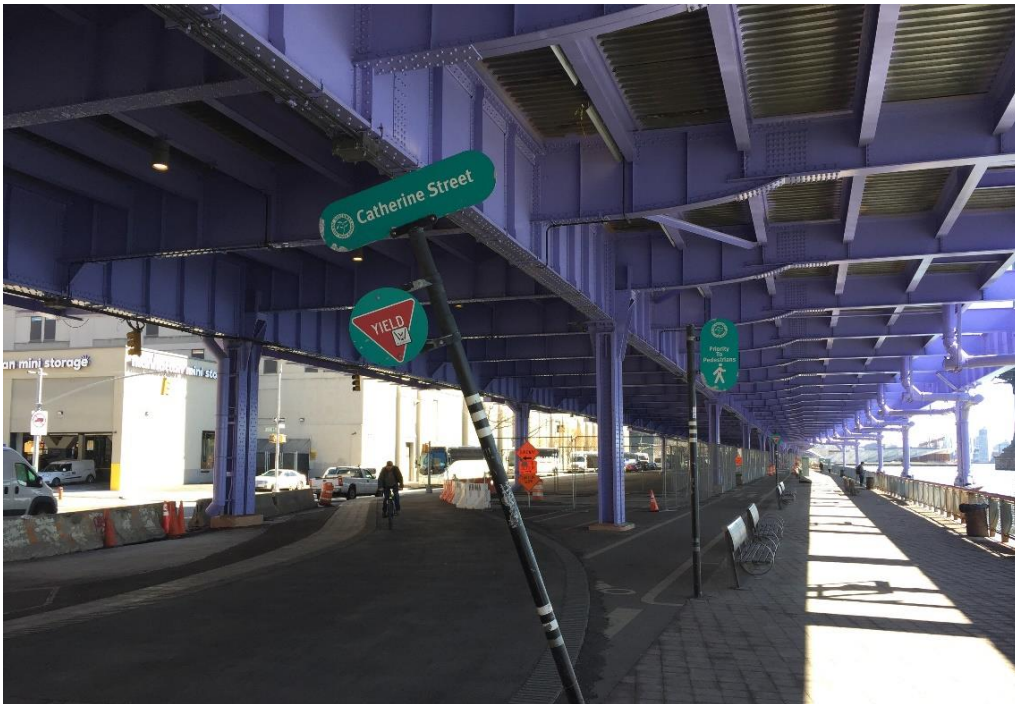
Photo 4: Under the FDR Drive and on the East River Waterfront Esplanade at Catherine Slip, looking north. The bike lane runs along the esplanade and was temporarily shifted due to construction.
