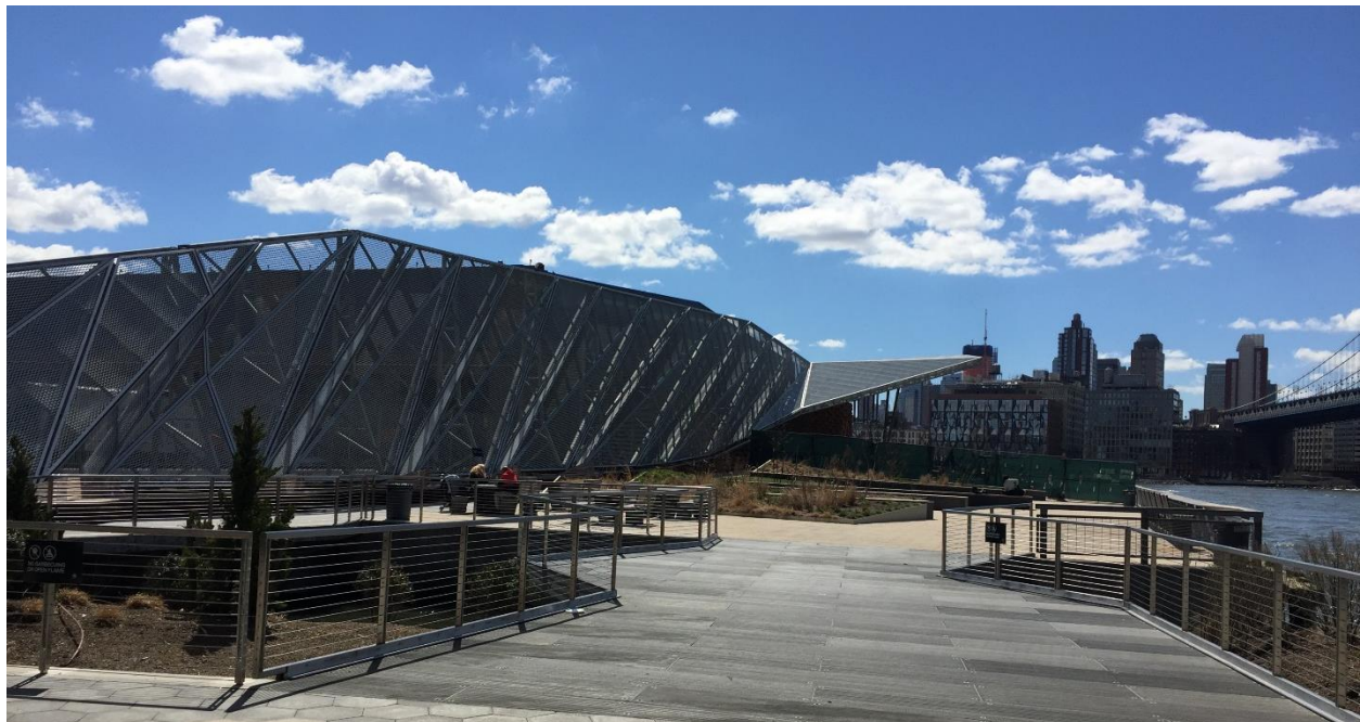
Photo 8: Looking east towards Brooklyn at the Pier 35 park, an outdoor public space.
