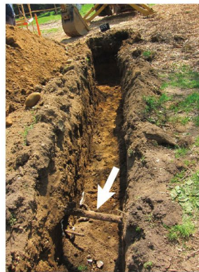
CB2 excavation looking southeast. Note electrical conduit (arrow). (5/4/15)
