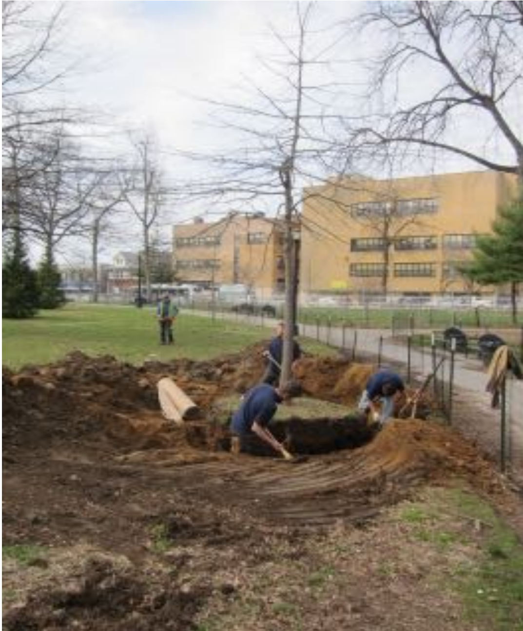
Photo 1. Excavating Tree No. 74 (later Tr -1) located north of the manor house. It was one of the larger trees slated for removal to allow relocation of the walk seen in the photo. The view is southwest with Jamaica Avenue in the far left background. (4-13-15)
