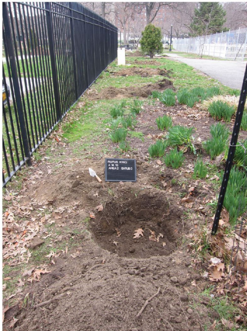
View along the line of shrub excavations adjacent to the home lot fence to the left. View is north from Shrub 3. (4/14/15)
