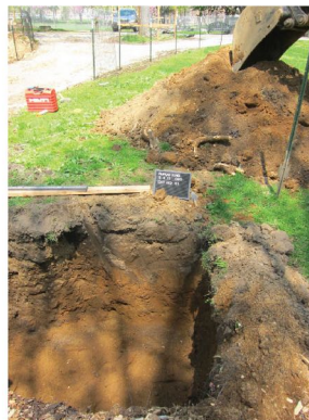
North wall of CB3 excavation with backdirt pile beyond. (5/4/15)
