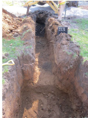
CB1 excavation looking east toward existing drain. (5/4/15)
