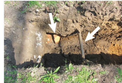
North end of CB2 excavation with electrical conduit (right arrow) and existing drain (left arrow) exposed. (5/4/15)
