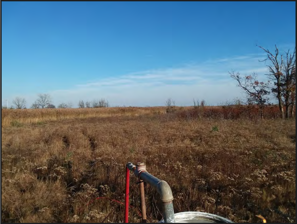
Photograph 1.6. General view of the southwestern end of the project alignment looking northeast across the Oakwood Beach marsh from near drill hole DH11 (Photographer: John Stiteler, November 2018).
