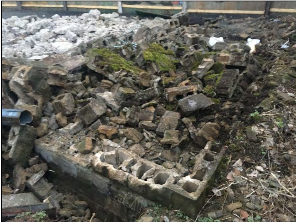
Photograph 4.11 Rubble pile from the aboveground demolition of the block shed, view to the west.
