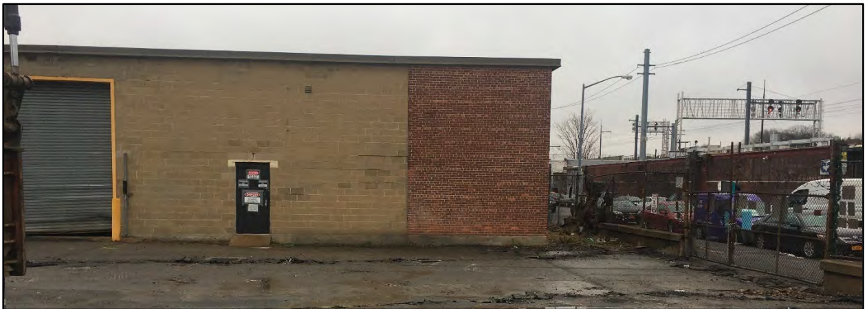
Photograph 1.4 The standing warehouse building adjacent to the eastern in-use entranceway, view to the east. Note the cut outs in the asphalt in preparation for the installation of the eastern entranceway gravel.
