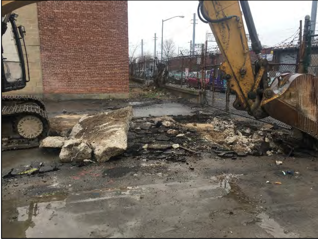
Photograph 4.2 Eastern construction with concrete slab underlying asphalt, view to the east.
