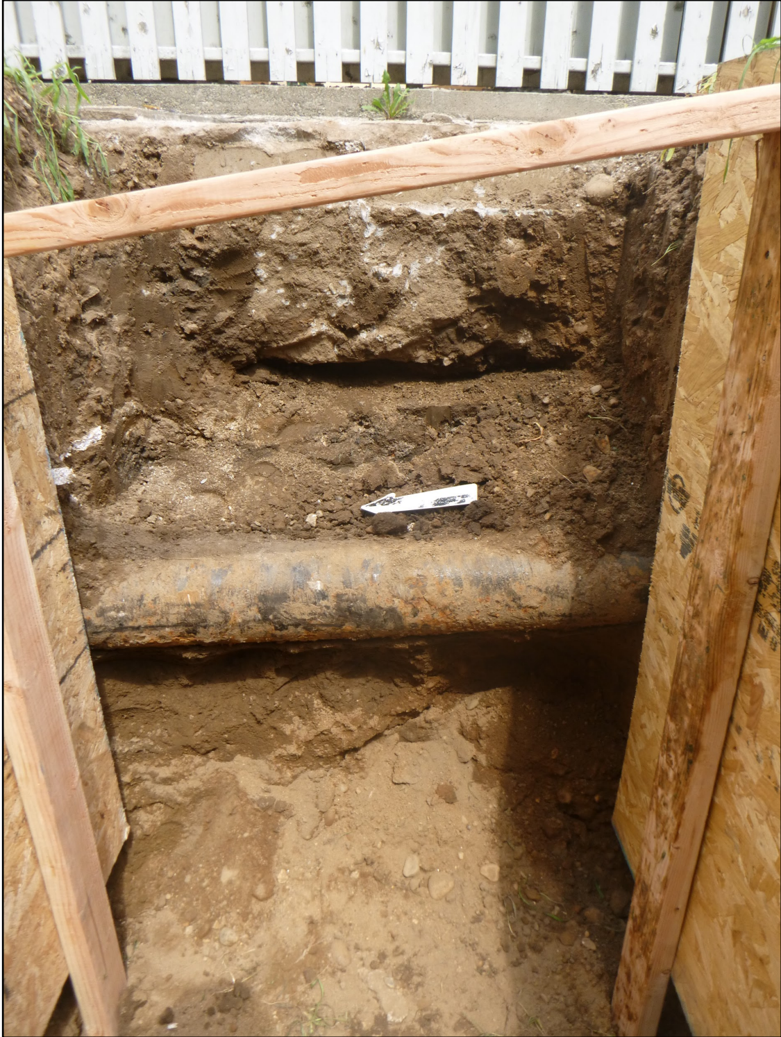
Image 9: Section 5 east wall profile showing electrical utility line at 2'5" bgs (.74m)
