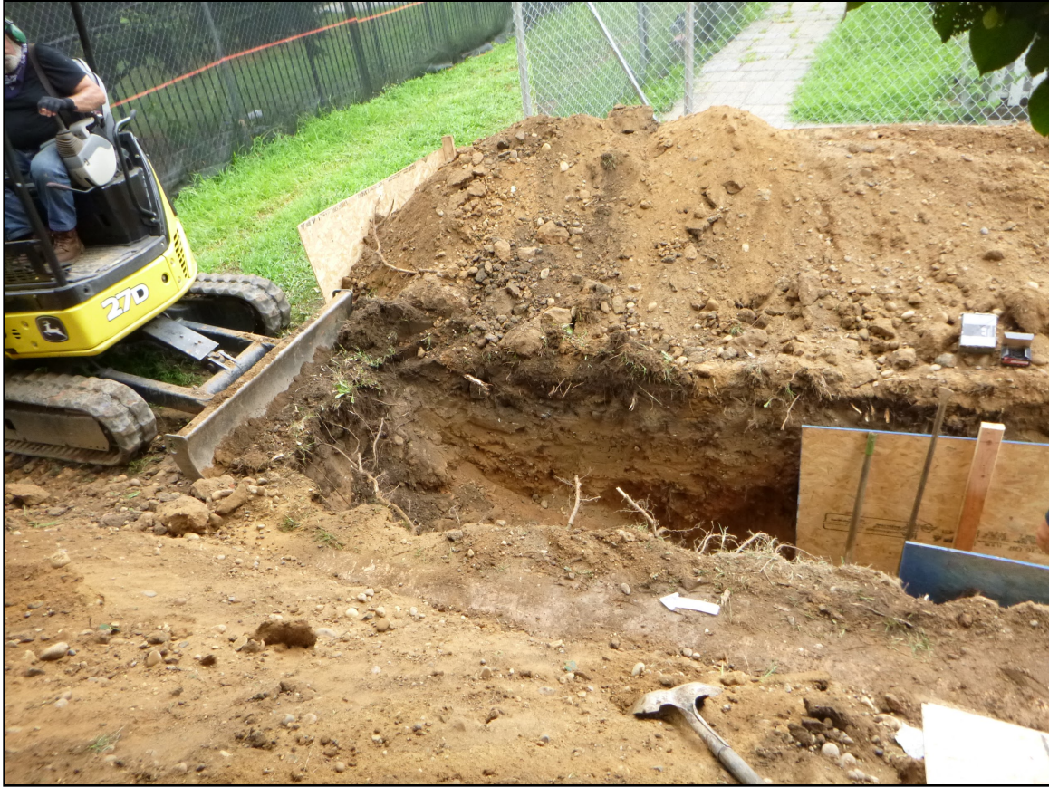
Image 11: Section 6 east wall profile at 5' bgs (1.52m).
