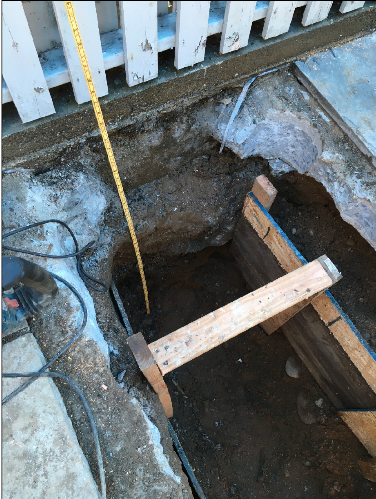
Image 13: Section 7 east wall showing concrete pad.
