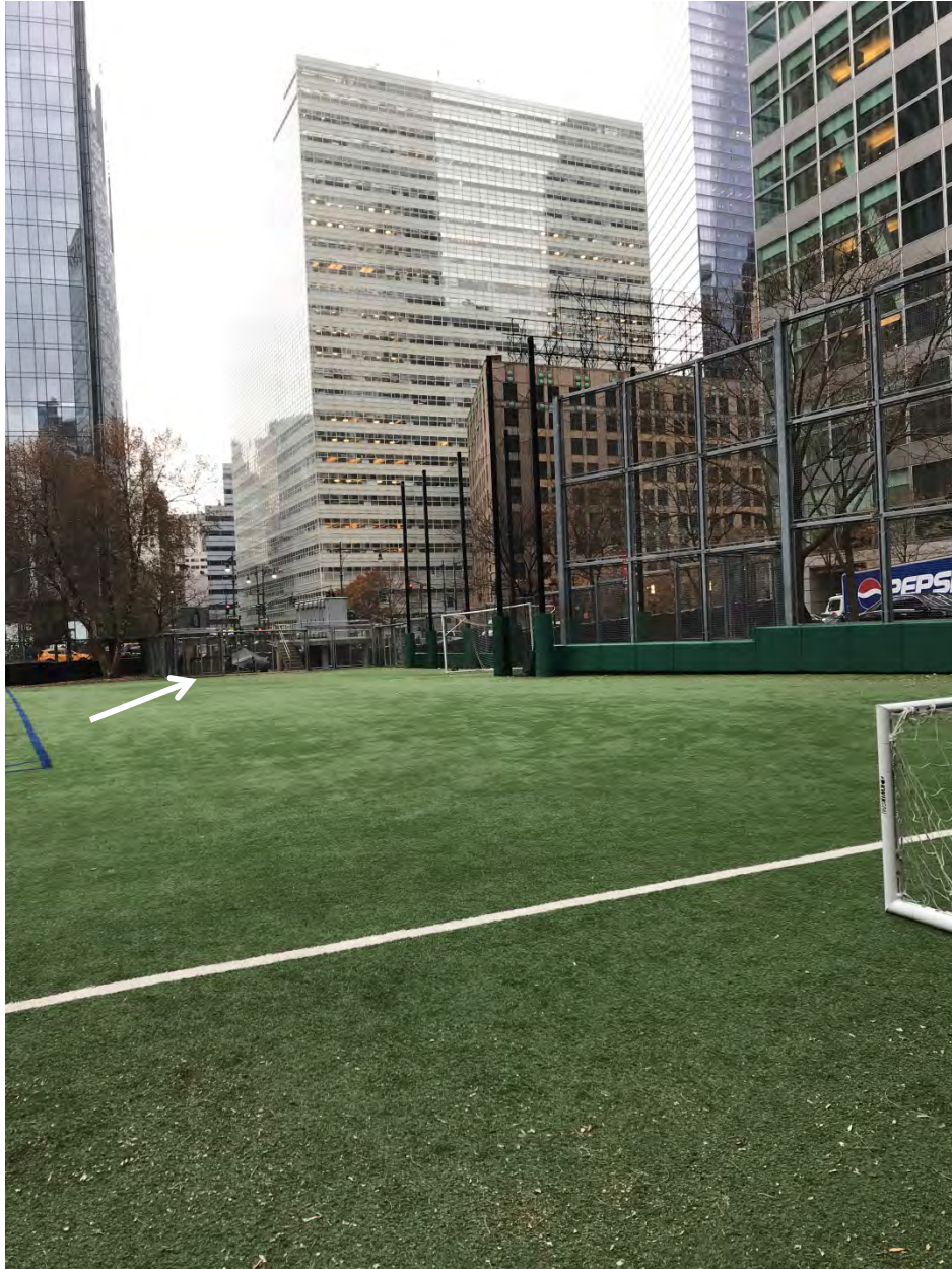
Photograph 5: Southeastern section of the Battery Park City Ballfields, facing southeast from the western edge of the fields. Arrow points to utility boxes at the extreme southeastern corner for the field.
