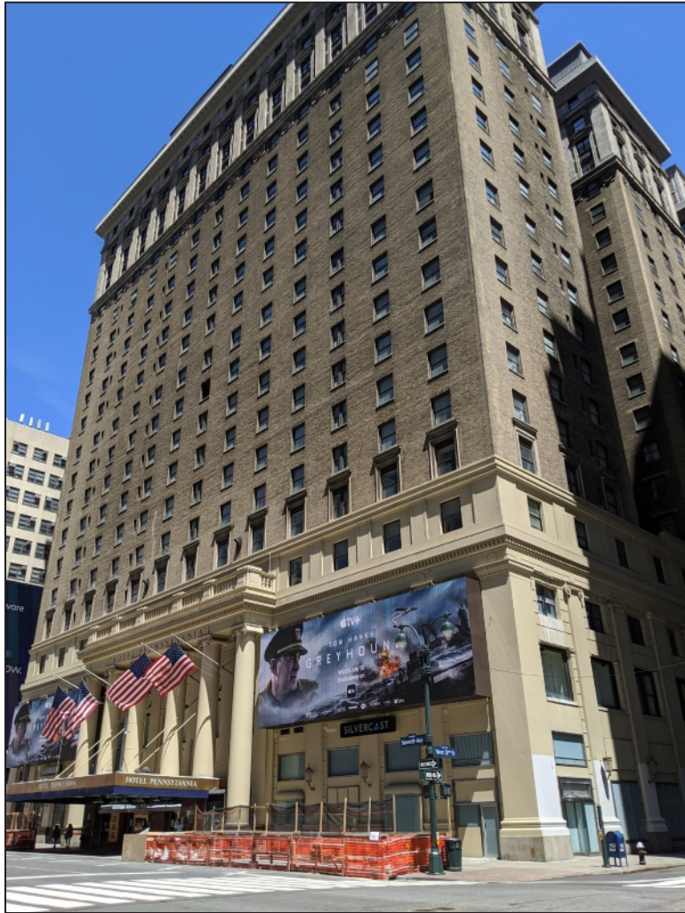
View of the Seventh Avenue façade of the Hotel Pennsylvania 1 looking north from West 32nd Street
