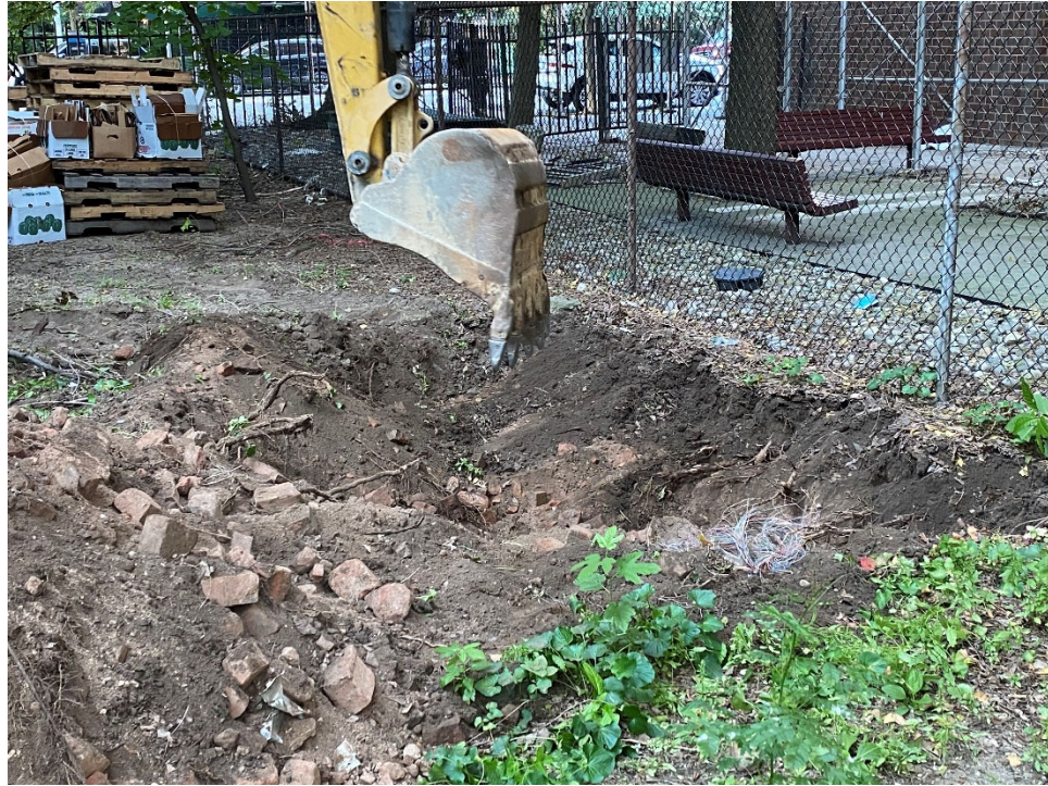
Photo 4-7 Surface Conditions at the Beginning of Mechanical Excavation of Trench 2
