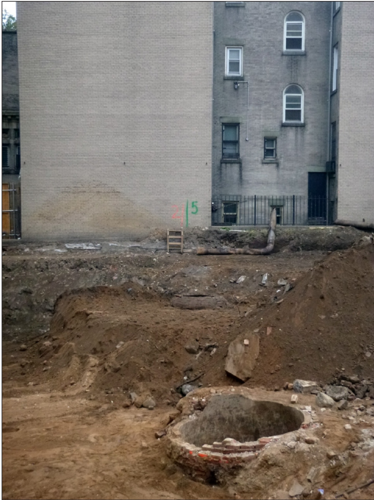
Looking north at the relationship between Feature 11 (foreground) and Feature 2 (visible in center), both of which were situated on the property formerly known as 267 Myrtle Avenue (CAC Field Image 839) 13
