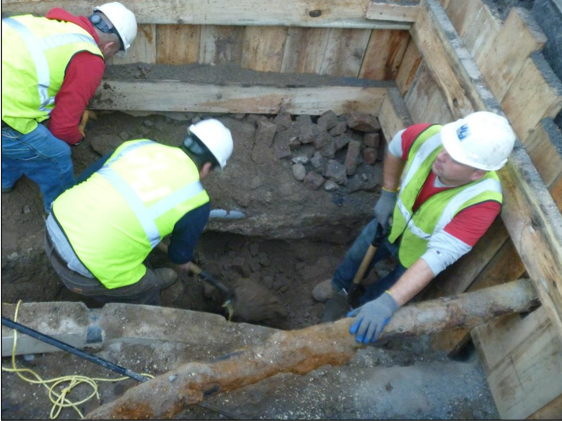
Image 06: Stratum V excavation in TP 20, facing east.
