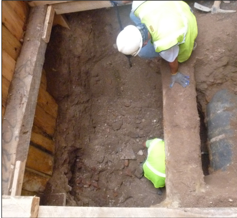
Image 01: Feature 1 in TP17 west profile, below shoring timbers.
