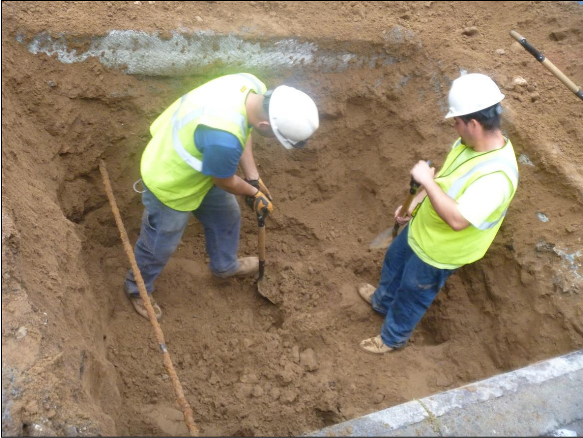
Image 07: TP 23 plan view in progress, facing north.
