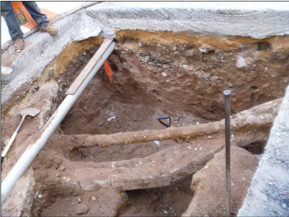
Image 02: TP 9 west profile before installing wood shoring.
