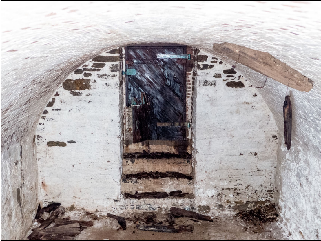
Image 11: Feature 2/Burial Vault 1 facing west, with patch on the roof of the vault.
