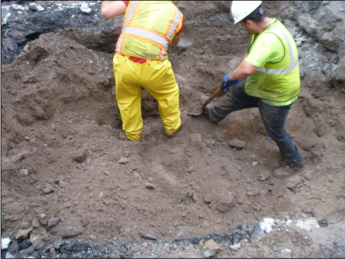
Image 03: TP 14 excavation in progress, facing north.
