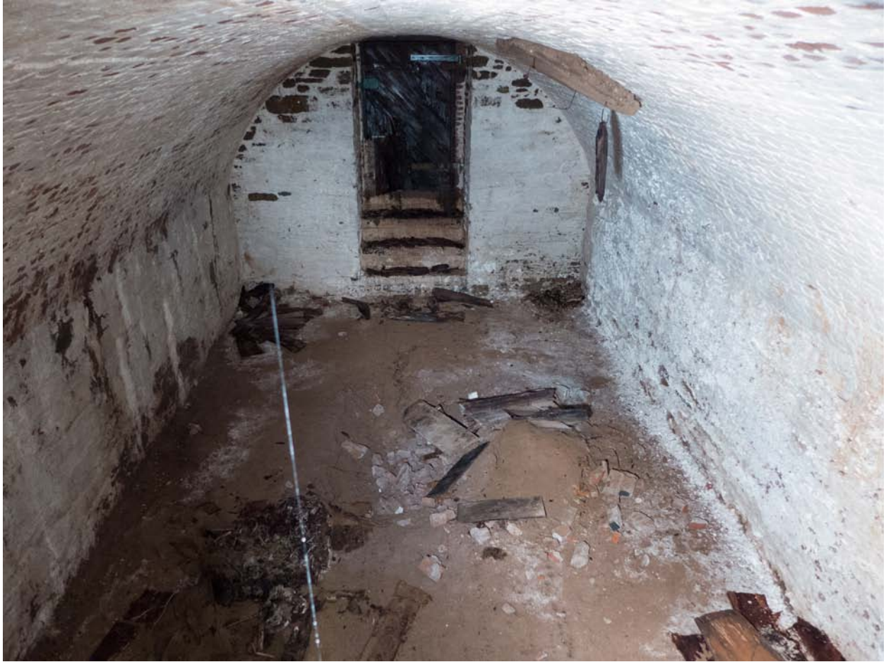
Image 01: Burial vault interior looking east.
