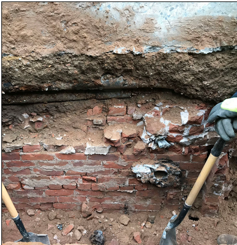
Image 09: Feature 14's eastern end in TR84 S6 north profile, with two previously cut utility pipes in its south face.
