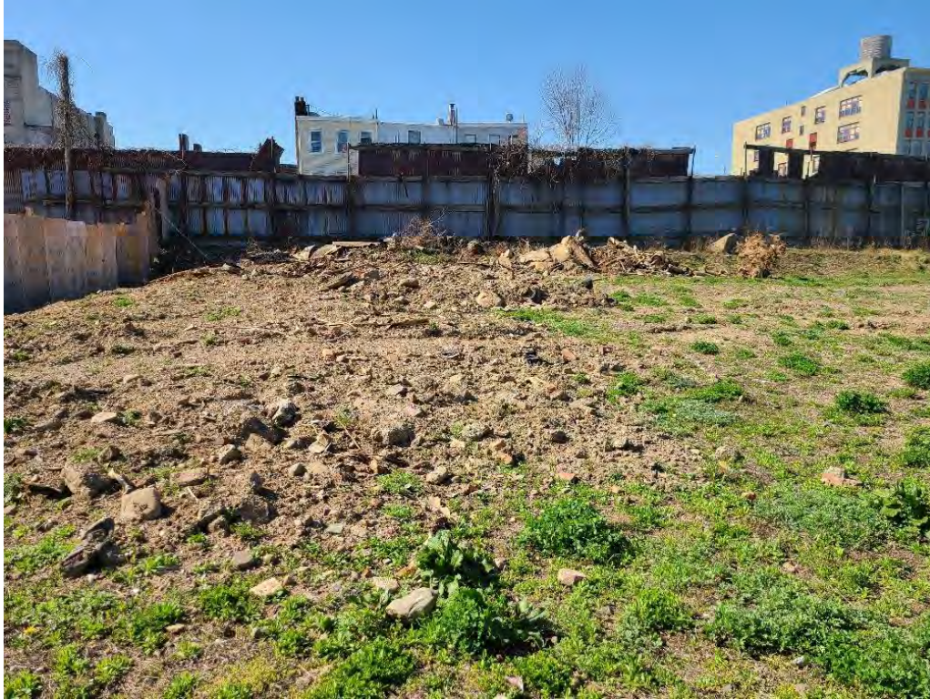
Photograph 3. Detail of the recent earthmoving at the southeastern side of the project site, with the new wooden fence on the left marking the lot boundary. View looking south.
