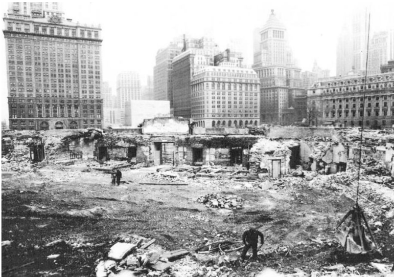
Photo 5. The photo shows the fort in 1941 after demolition of the exterior brick wall introduced earlier to support the the building's use as an aquarium. The view is northeast with the Customs House in the far right background. (Anonymous 1941)
