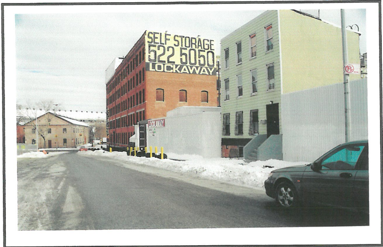
Photo 5: View to west of 19 th century industrial building fronting Flushing Avenue.
