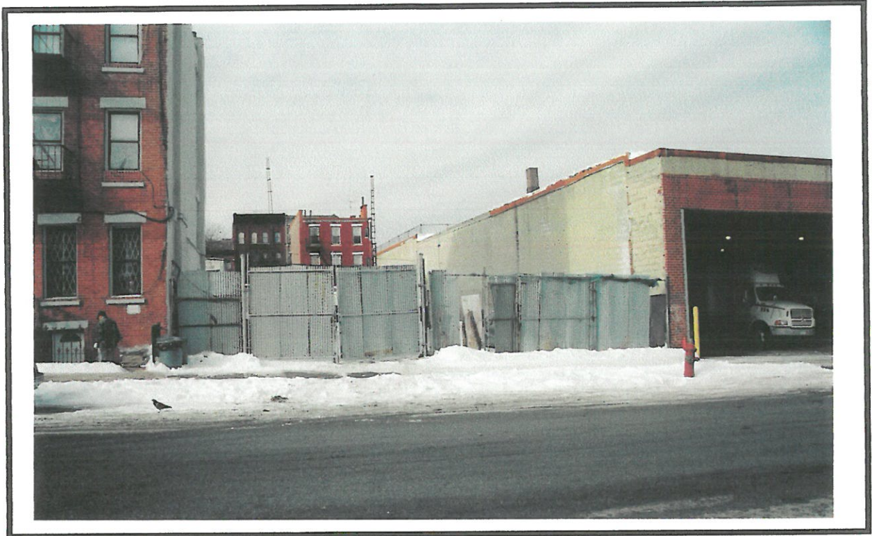
Photo 1: Looking south to 30 & 32 Carlton Avenue. Lots are currently vacant, undeveloped land.
