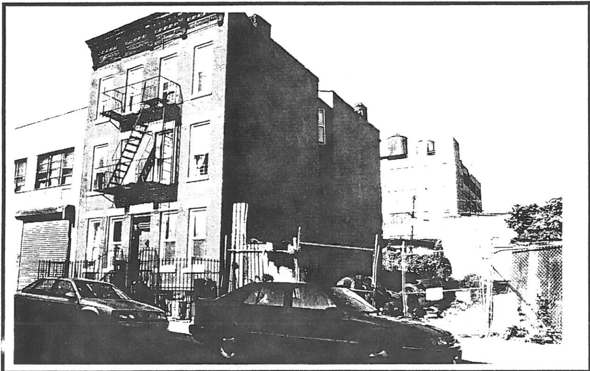
Photo 8: This brick 3-story building at 122 Walworth Street is an example of a “new law” tenement. New law tenements had light wells with windows in the center of the building to provide light and ventilation to the interior rooms. This building dates to the late 19 th century.
