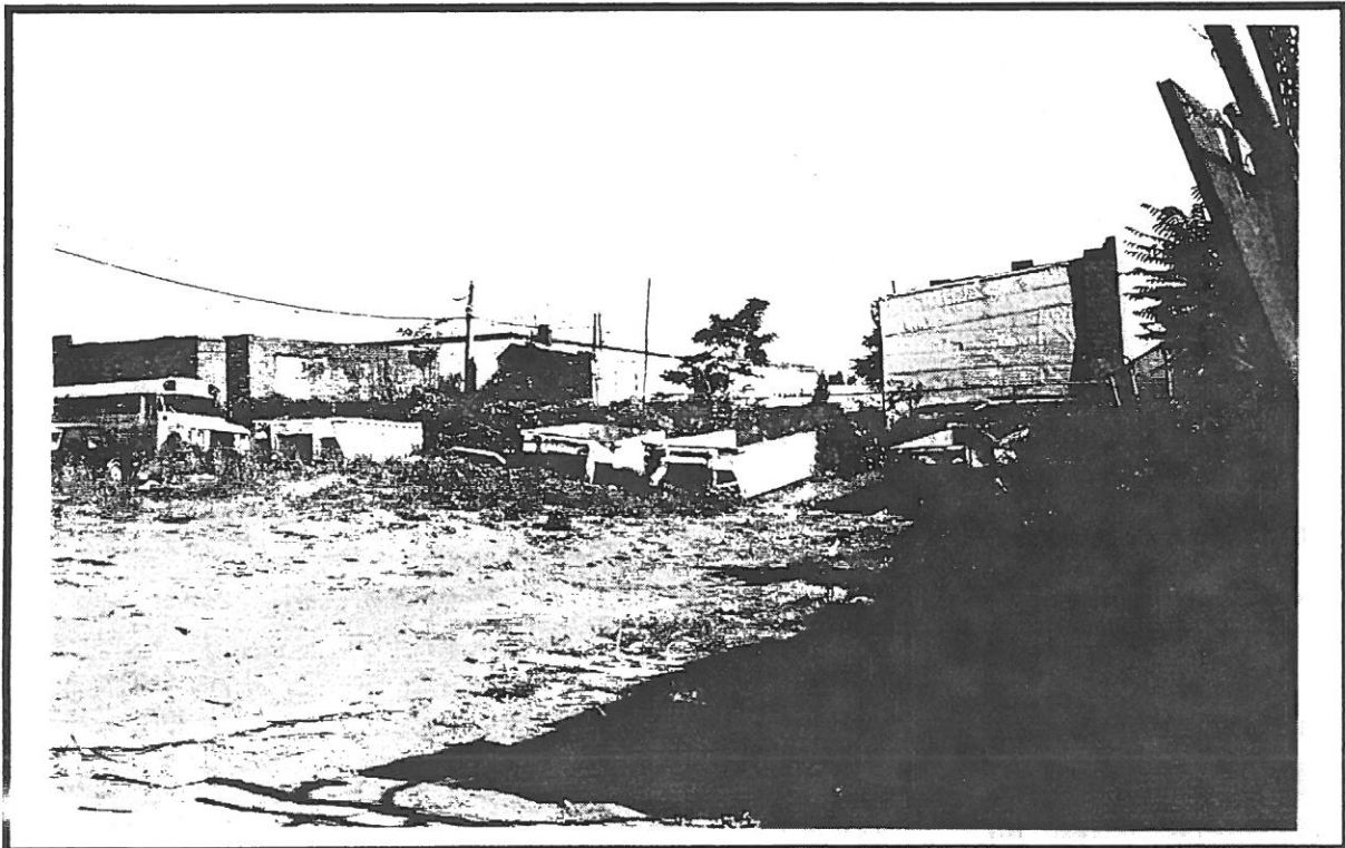
Photo 2: Debris and junked vehicles occupy the project area. View is to northwest looking to 108-110 Walworth Street.
