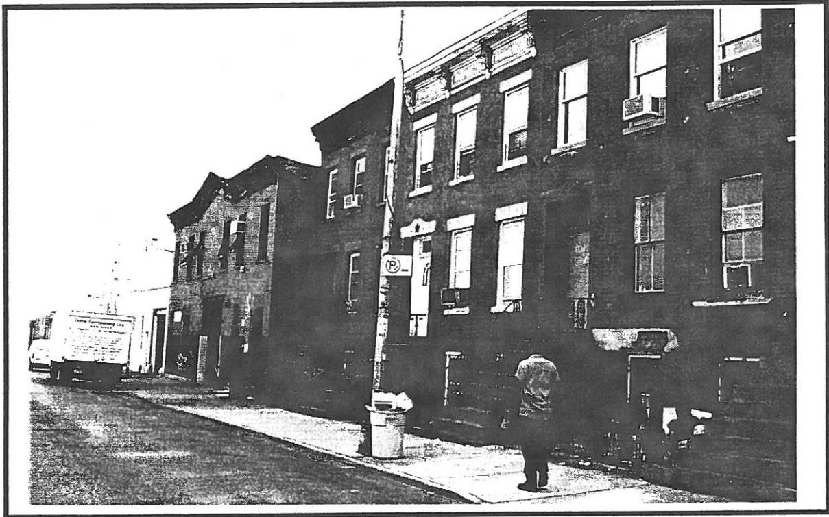
Photo 9: Brick buildings in the Italianate-style dominate the east side of Walworth Street, as opposed to the frame dwellings that were located on the west side. View to northeast.
