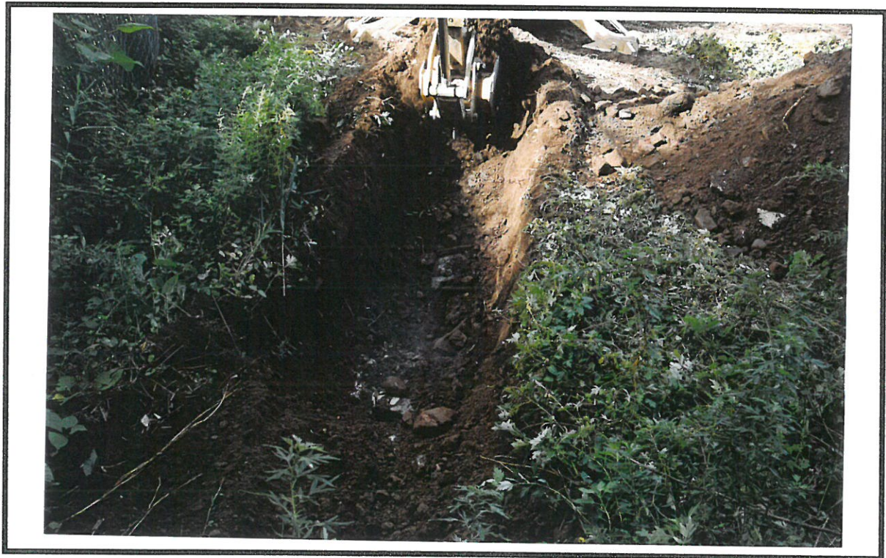
Photo 10: Trench 8 was excavated along the line of Red Hook Lane, which represented the historic rear lot lines of Lot 12-15 & 22-24. It was thought possible that privies might be located along this line.
