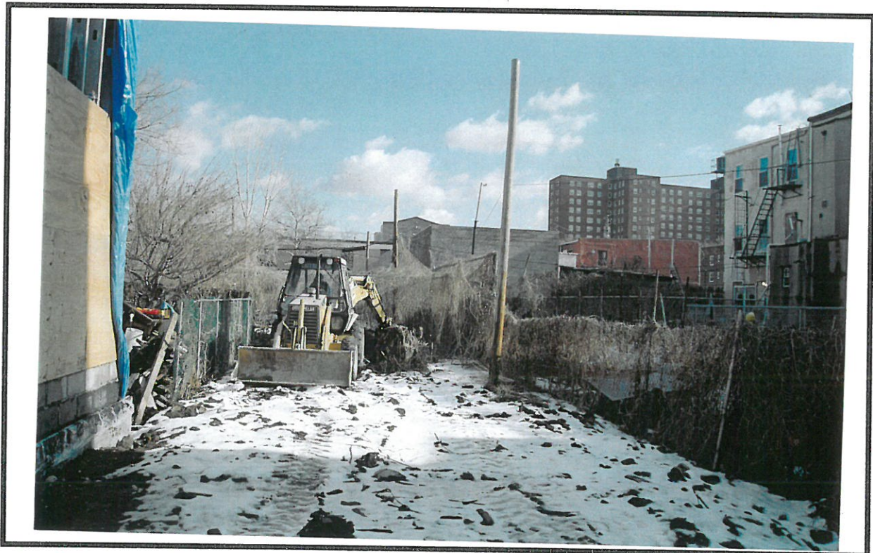
Photo 18: Backhoe preparing to excavate Trench 13 on rear of Lot 43 (Dikeman Street) in February 2005. Reported to be location of shed or shack, a light scattering of artifacts were recovered, but no evidence of structure or shaft feature was identified. View to northwest
