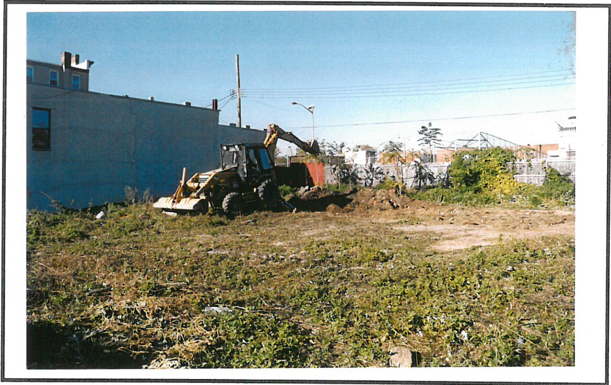
Photo 3: Backhoe excavating Trench 5 on Lot 12. View to northwest.
