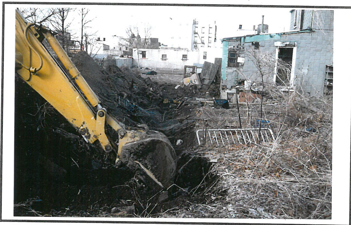
Photo 5: Excavating Trench 10 on Lot 26 in January 2005. Trench 4 (Lot 24) is essentially an extension of Trench 10. View to west.
