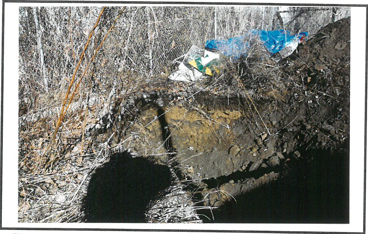
Photo 17: Excavating west side of Trench 12 in effort to located privy on Lot 28. Beneath frozen top soil, soils were sandy and soft. View to west.
