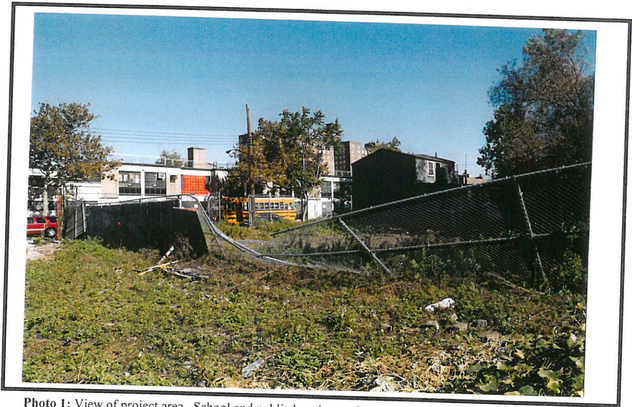
Photo 1: View of project area. School and public housing project are to the north and northeast. Chain link fence divides several of the lots within the project area. This fence divides Lot 15 from Lot 14. House on Lot 24 is only structure remaining on the project area.
