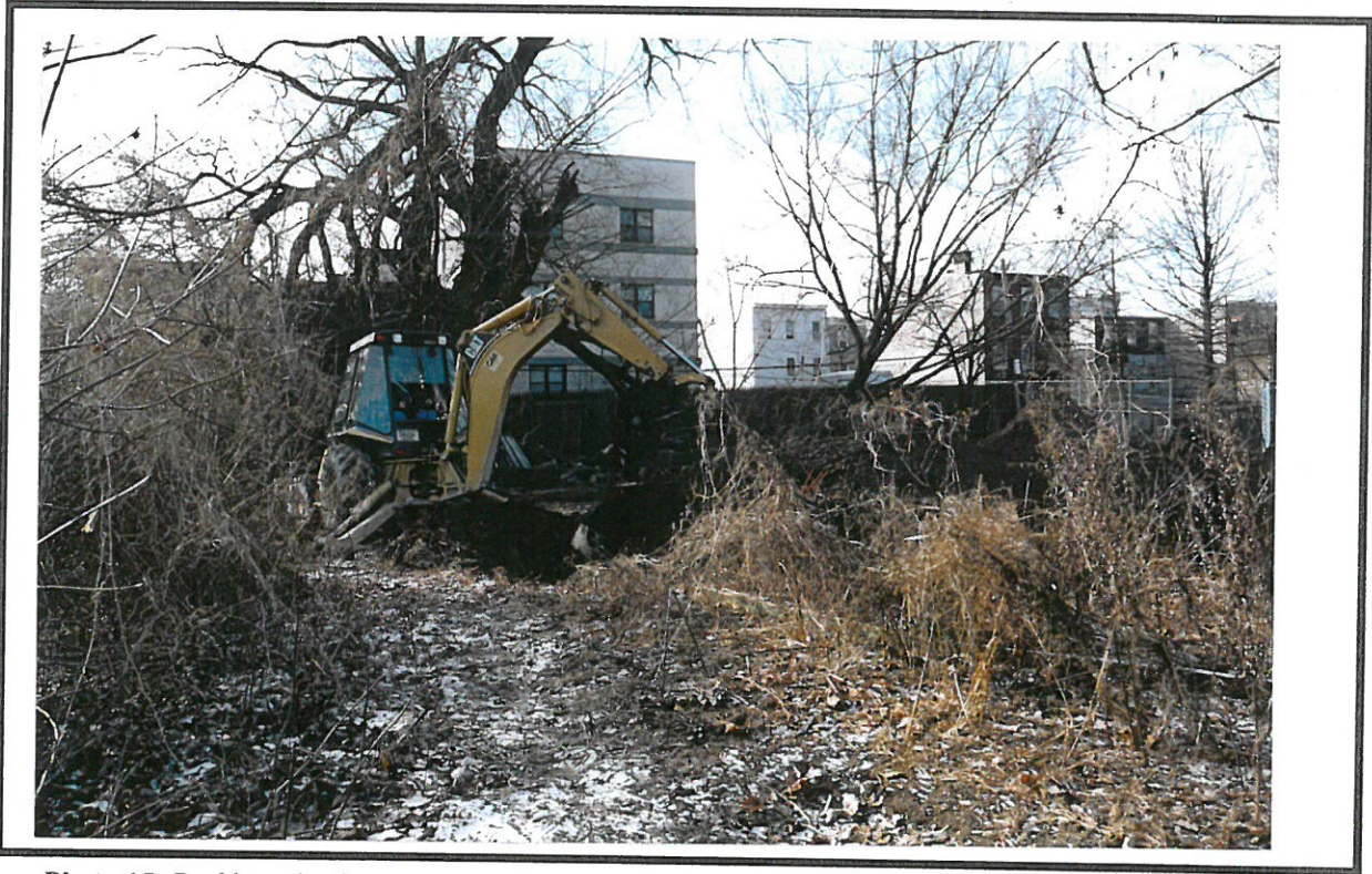
Photo 15: Backhoe clearing area on Lot 27 near large willow tree that prevented excavation along rear lot line. View to southwest.
