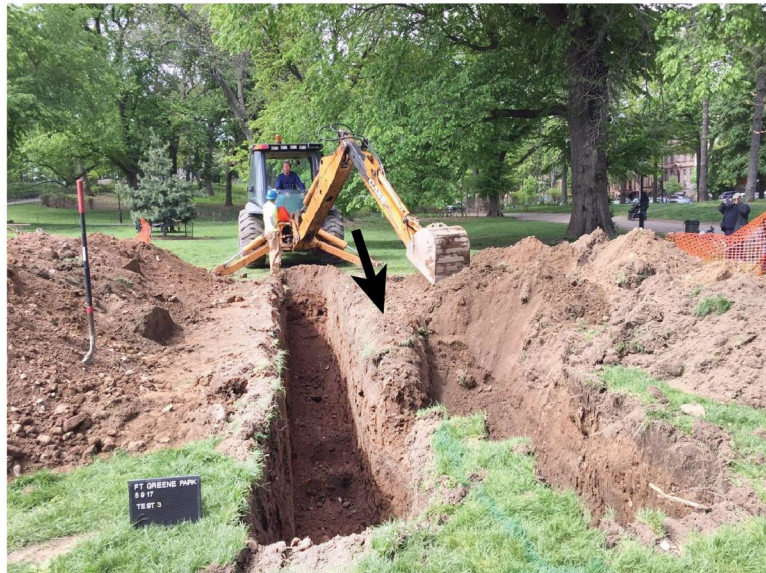
9c Test No. 3 looking north. The trench, on the west side of the property line addressed in Test No. 2, now partially backfilled, was also the possible location of a privy pit for a tenanted dwelling in the 1840s. The baulk (arrow) between the two trenches soon partially collapsed. (Geismar 5/9/17)
