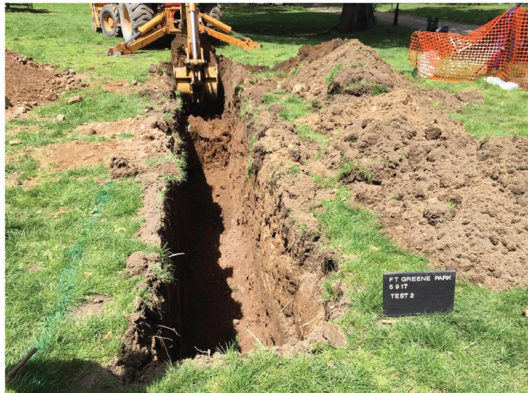
8c Test No. 2 looking north. The trench is near the rear property line of a former tenanted dwelling, the possible location of a privy pit in the 1840s. Note the color variation in the excavated soils. (Geismar 5/9/17)
