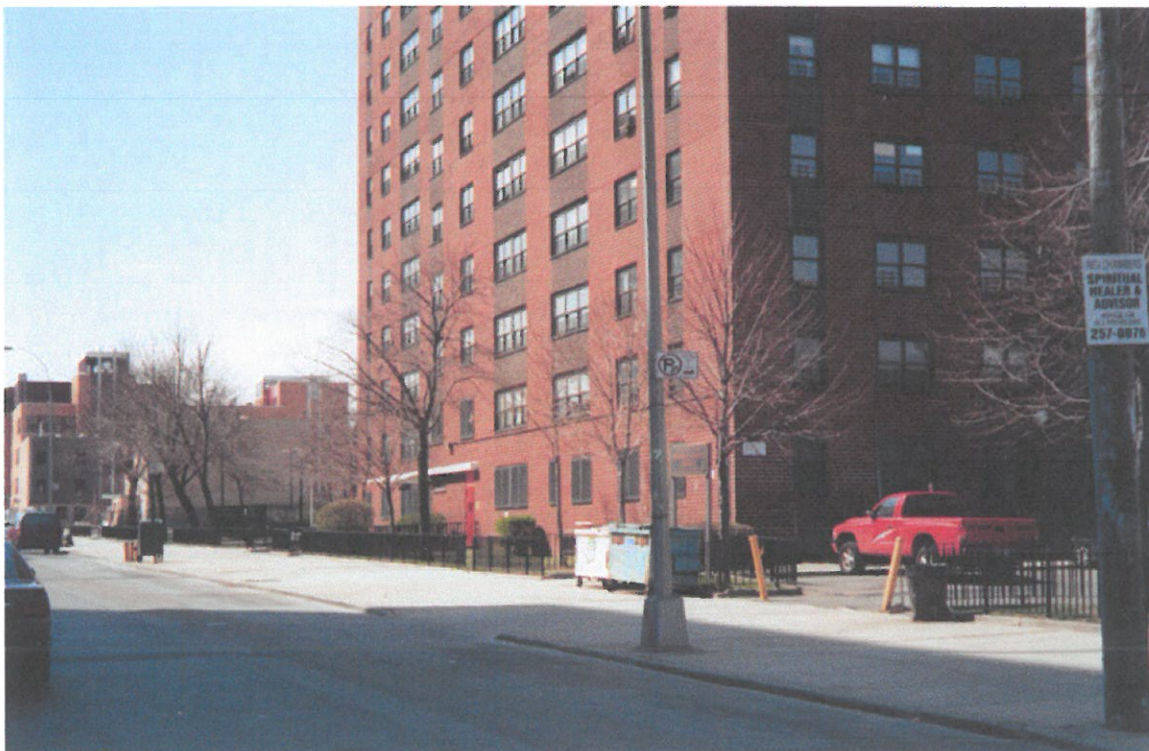
Photograph Number 6: View of Prospect Plaza Hope VI Revitalization Area – Site A, facing northwest from Prospect Place.
