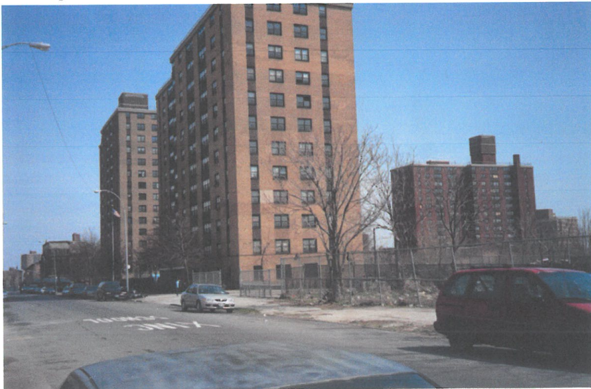
Photograph Number 8: View of Prospect Plaza Hope VI Revitalization Area – Sites B and C, facing southeast from Prospect Place.
