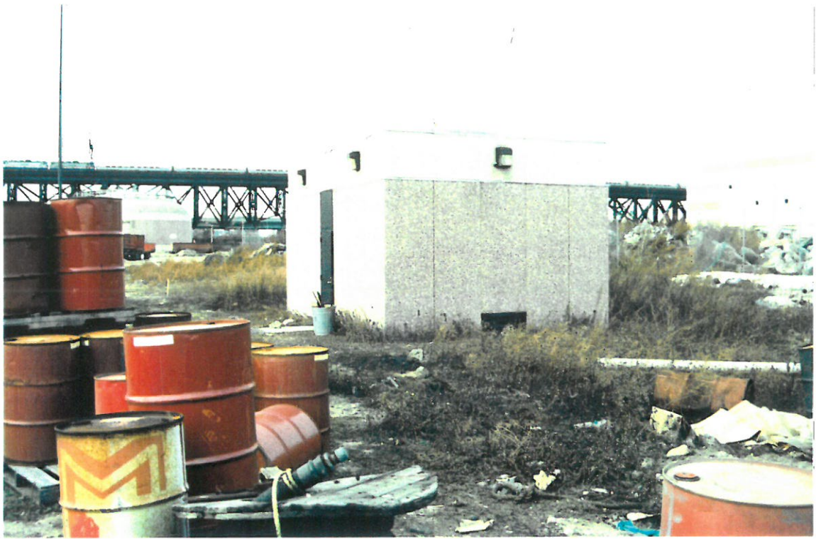
Photo 6 - Paint Storage Building View Is To The West
