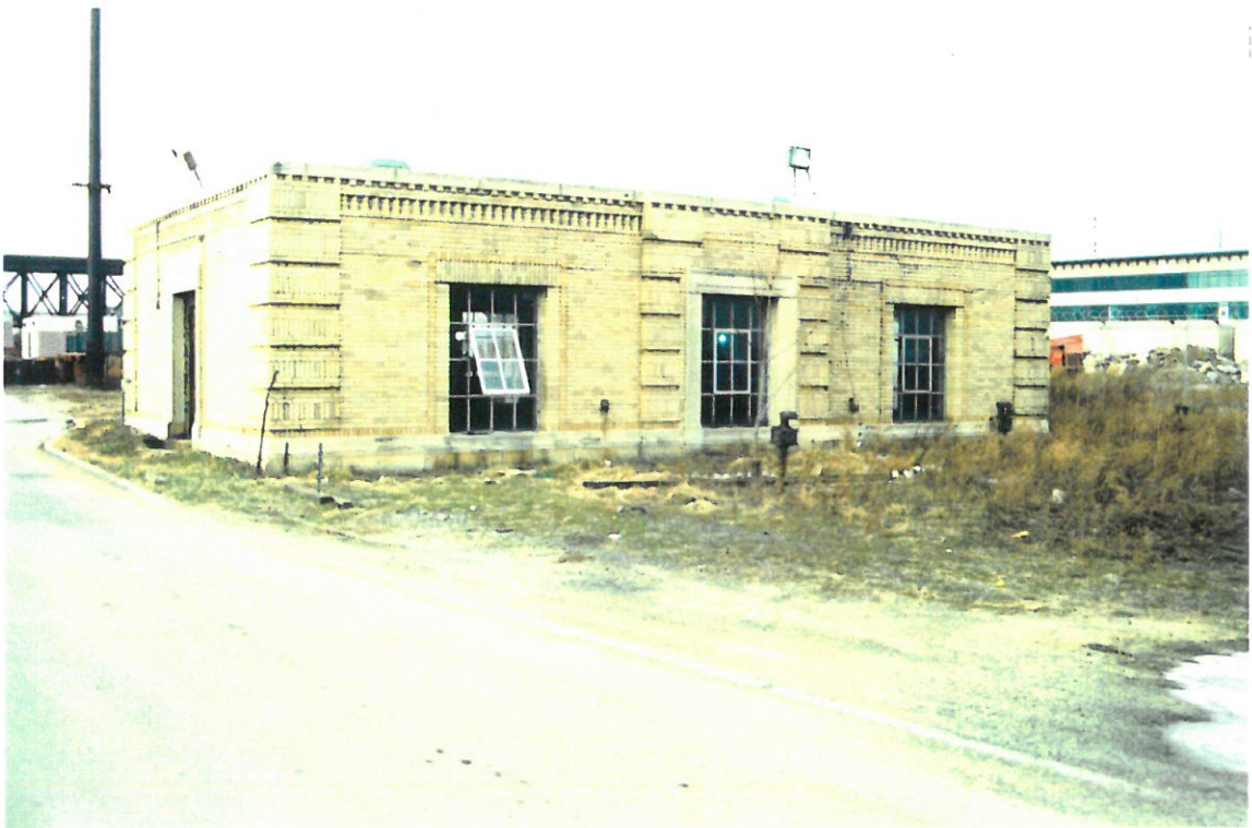
Photo 7 - Fuel Oil Storage Building View Is To The West
