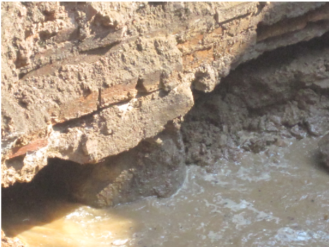
Photograph 5. Trench 26-1, Feature 3 footing.
