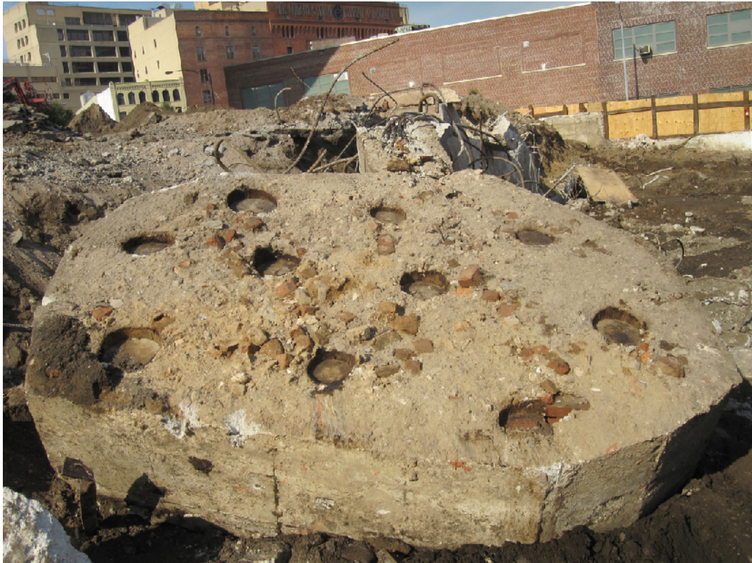
Photograph 42. Pile cap.
