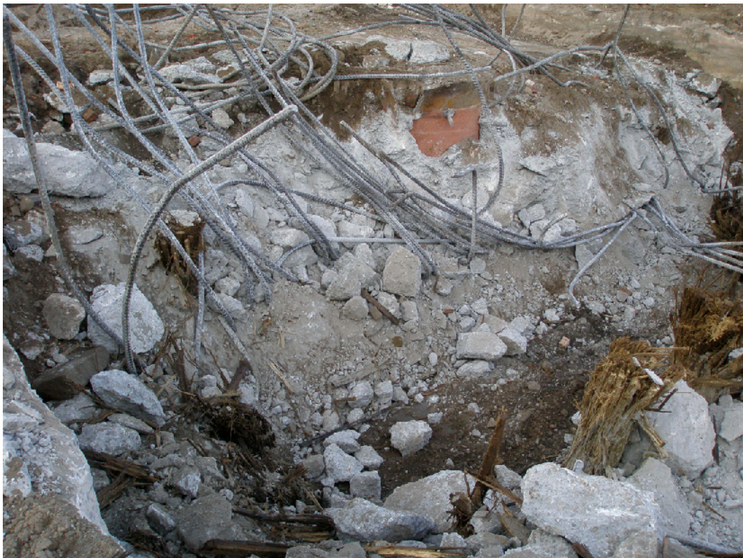
Photograph 41. Trench 22-2, billboard base and pile cap.
