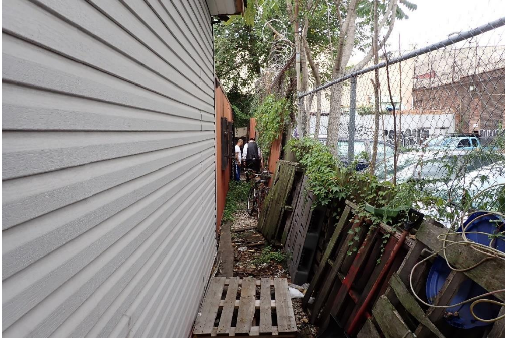
Photograph 2. South side of the project area, note temporary structure and metal shipping containers, facing east.
