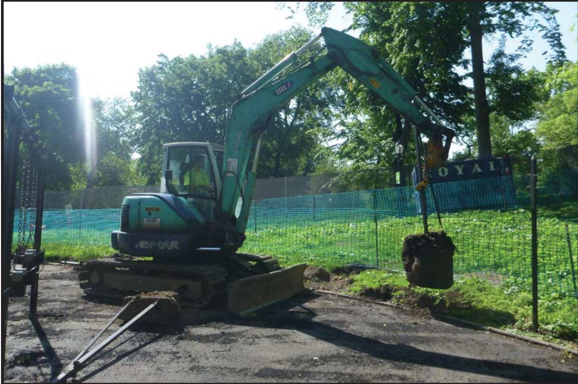
Photograph 3.5. Mariners' Playground, view facing southeast showing the removal of fence posts in progress at the southern edge of the playground (Photographer: James Lee, May 2016) [HRI Neg.#16020/D1:002].
