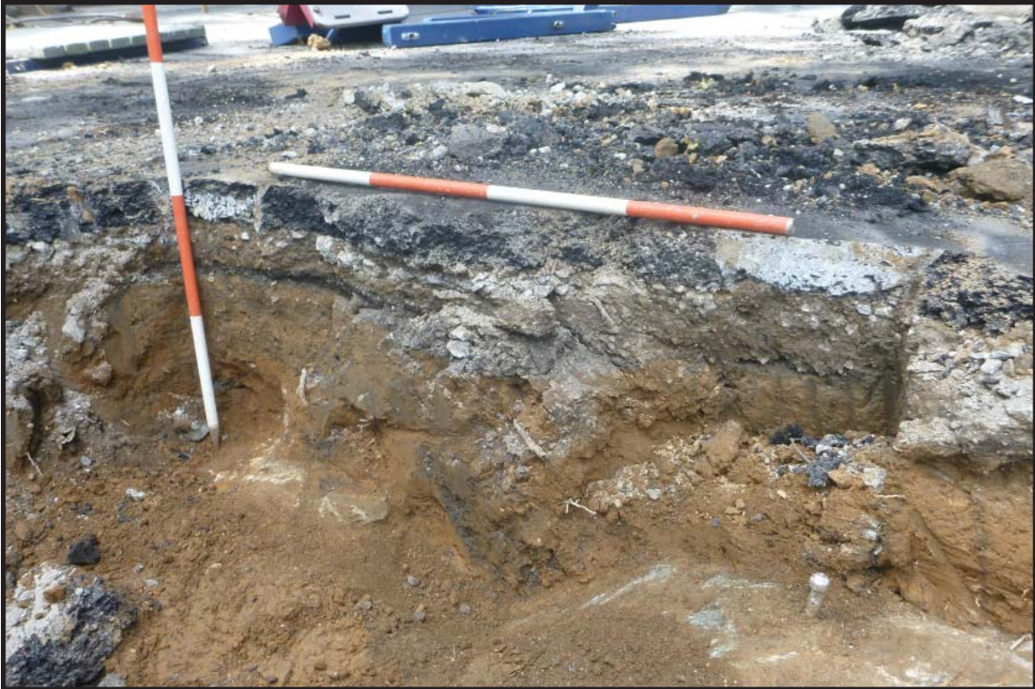
Photograph 3.13. Mariners' Playground, view facing north showing the northeast profile of Contractor Excavation 5. Scale rods are in feet. Note the bedrock with protruding steel bolts at the base of the excavation (Photographer: James Lee, May 2016) [HRI Neg.#16020/D1:025].
