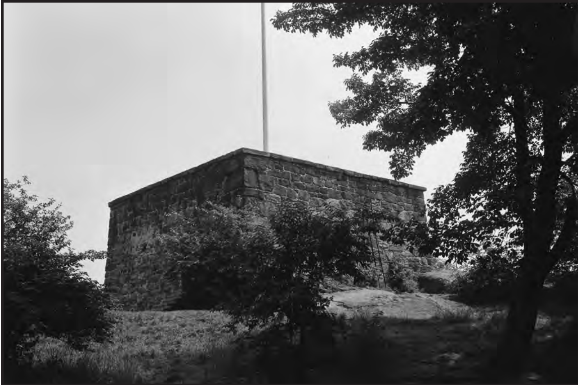
Photograph 2.11. Historic view looking northeast, May 1962. Note flagpole in northeast corner of the building, restored masonry, embrasures and parapet, iron ladder, and brick and stone exterior stair. Source: New York City Parks Department (Central Park Conservancy 31593).
