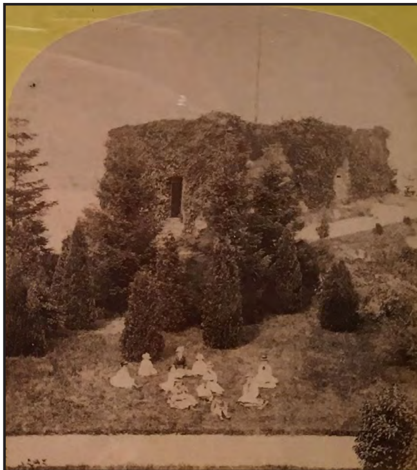
Photograph 2.4. Historic view looking northeast, circa 1875. Note flagpole in northeast corner of the building, stair leading up to doorway and apparent removal of pedimented roof. The blockhouse is clearly no longer in use as a magazine for storing gunpowder by this date. Source: Unknown Photographer, Stereographic View (Metropolitan Museum of Art, Herbert Mitchell Collection 2007.457.69).
