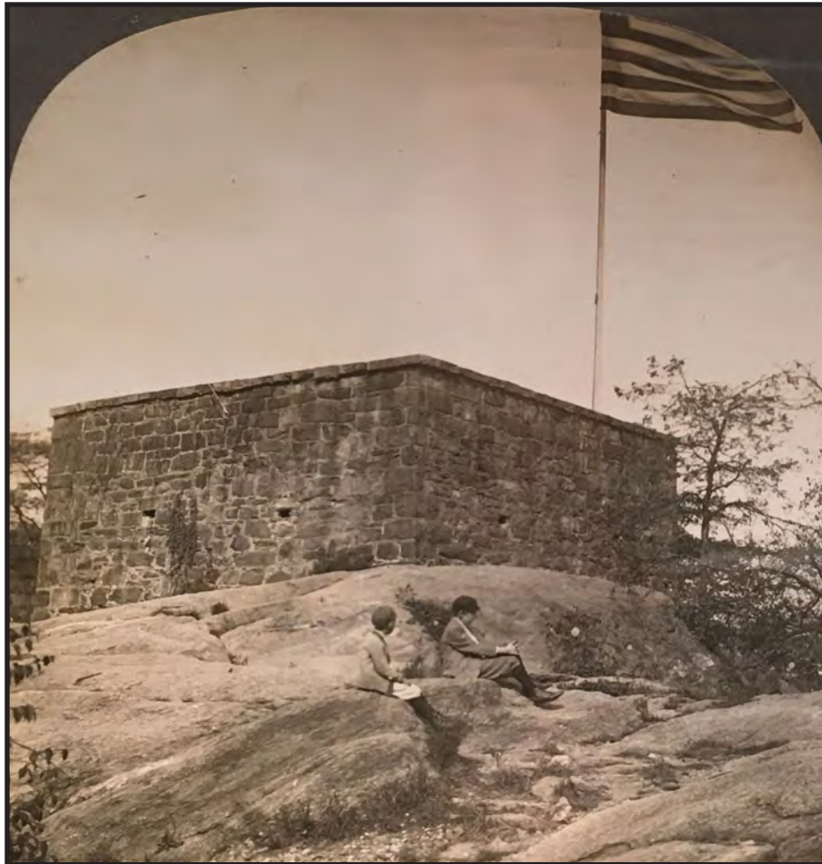
Photograph 2.7. Historic view looking northwest, 1909. Note flagpole in north-east corner of the building, restored masonry, embrasures and parapet. Source: Unknown Photographer, Stereographic View (Metropolitan Museum of Art, Herbert Mitchell Collection 2007.457.70).
