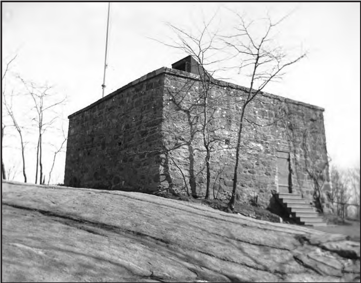
Photograph 2.5. Historic view looking southeast, 1899. Note flagpole in northeast corner of the building, interior stairway hood along west wall, restored masonry, embrasures and parapet, and wooden exterior stair leading up to iron door. Source: George E. Stonebridge (New-York Historical Society, George E. Stonebridge Collection 63861-4868).
