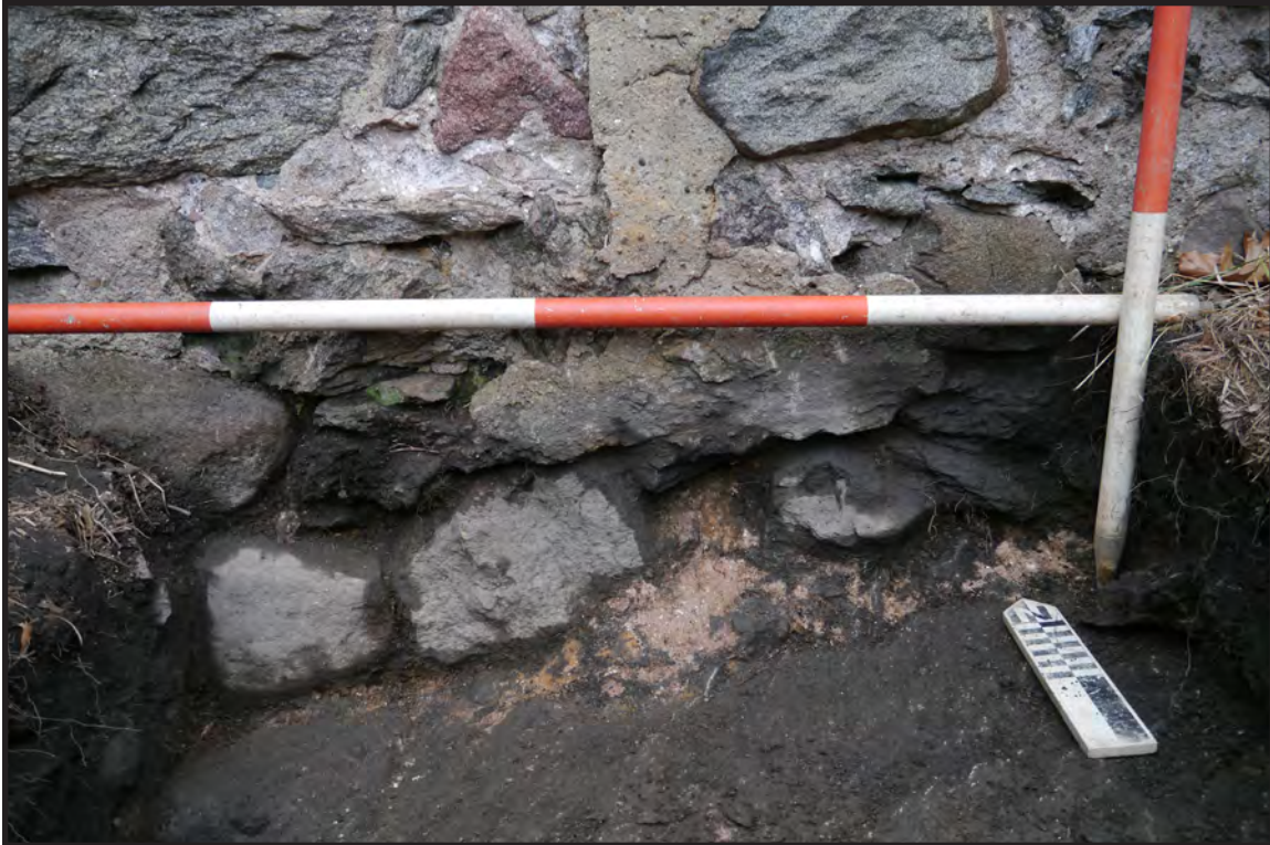
Photograph 4.14. View facing north showing Excavation Unit 3 and the bedding mortar observed between the bedrock and the bottom of the blockhouse foundation; scales in feet and tenths of feet (Photographer: James Lee, December 2017 [HRI Neg.#17070/D1:183]).
