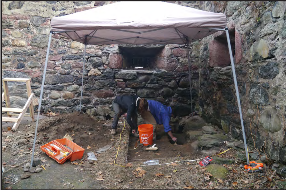
Photograph 4.2. View facing east showing Excavation Unit 2 in progress in the southeast corner of the blockhouse (Photographer: James Lee, December 2017 [HRI Neg.#17070/D1:048]).
