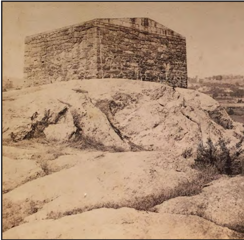
Photograph 2.3. Historic view looking southwest, circa 1865. Note shallow pedimented roof and blocked embrasures. The blockhouse at this time may still have been in use as a magazine for storing gunpowder. Source: Unknown Photographer, Stereographic View (Metropolitan Museum of Art, Herbert Mitchell Collection 2007.457.67).
