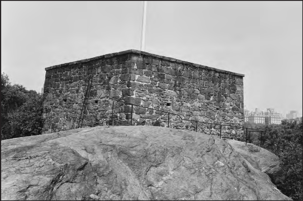
Photograph 2.10. Historic view looking southwest, May 1962. Note flagpole in northeast corner of the building, restored masonry, embrasures and parapet, iron railing and ladder. Source: New York City Parks Department (Central Park Conservancy 31592).
