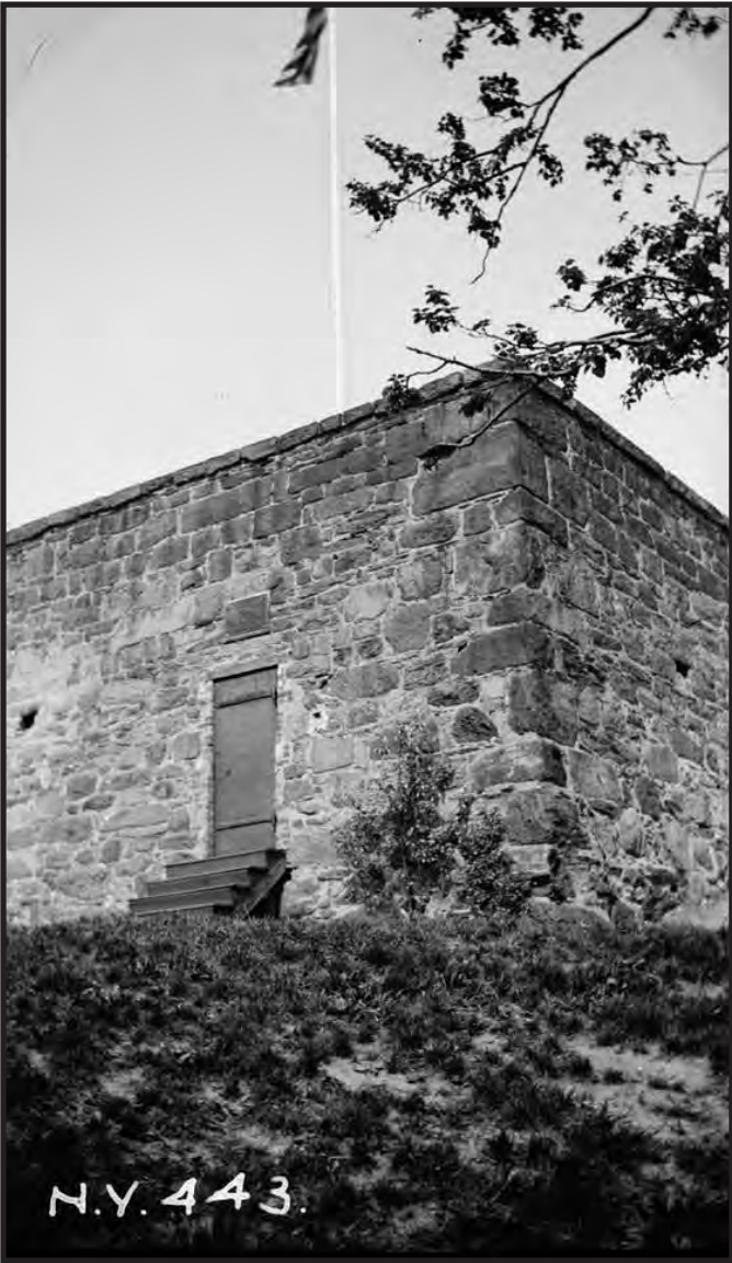
Photograph 2.8. Historic view looking northeast, February 16, 1936. Note flagpole in northeast corner of the building, absence of interior stairway hood along west wall, restored masonry, embrasures and parapet, and wooden exterior stair leading up to iron door. Source: Wakefield Worcester (Historic American Buildings Survey NY 443).
