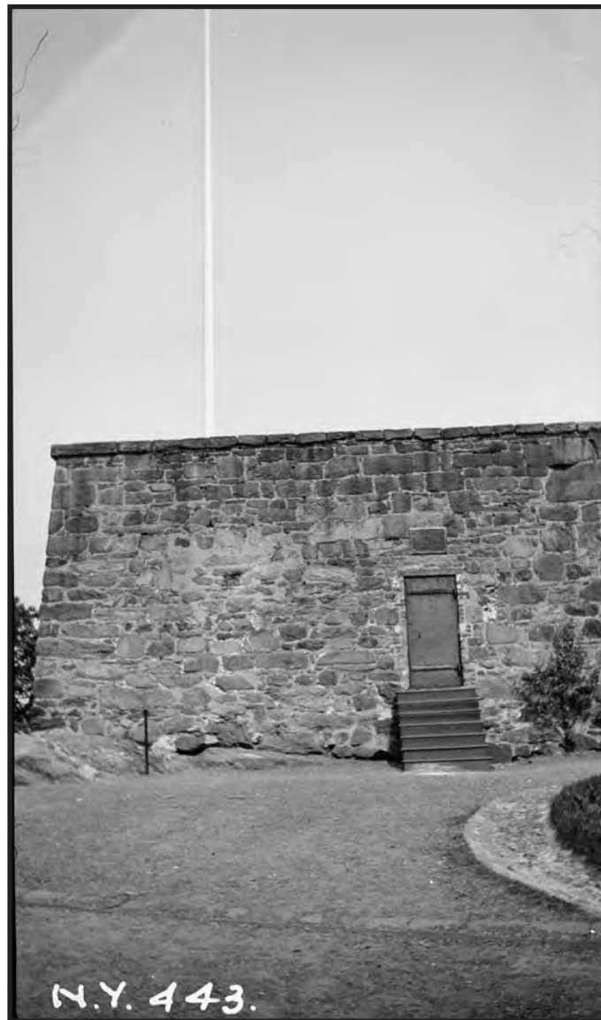
Photograph 2.9. Historic view looking east, May 12, 1936. Note flagpole in northeast corner of the building, restored masonry, embrasures and parapet, and wooden exterior stair leading up to iron door. Source: Arnold Moses (Historic American Buildings Survey NY 443).
