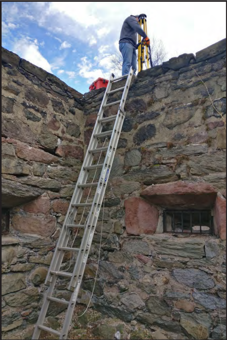
Photograph 3.3. View facing southeast showing digital laser scanning equipment being set up on top of the southern wall of the block-house to scan the top and interior (Photographer: James Lee, March 2017 [HRI Neg.#17013/D1:017]).
