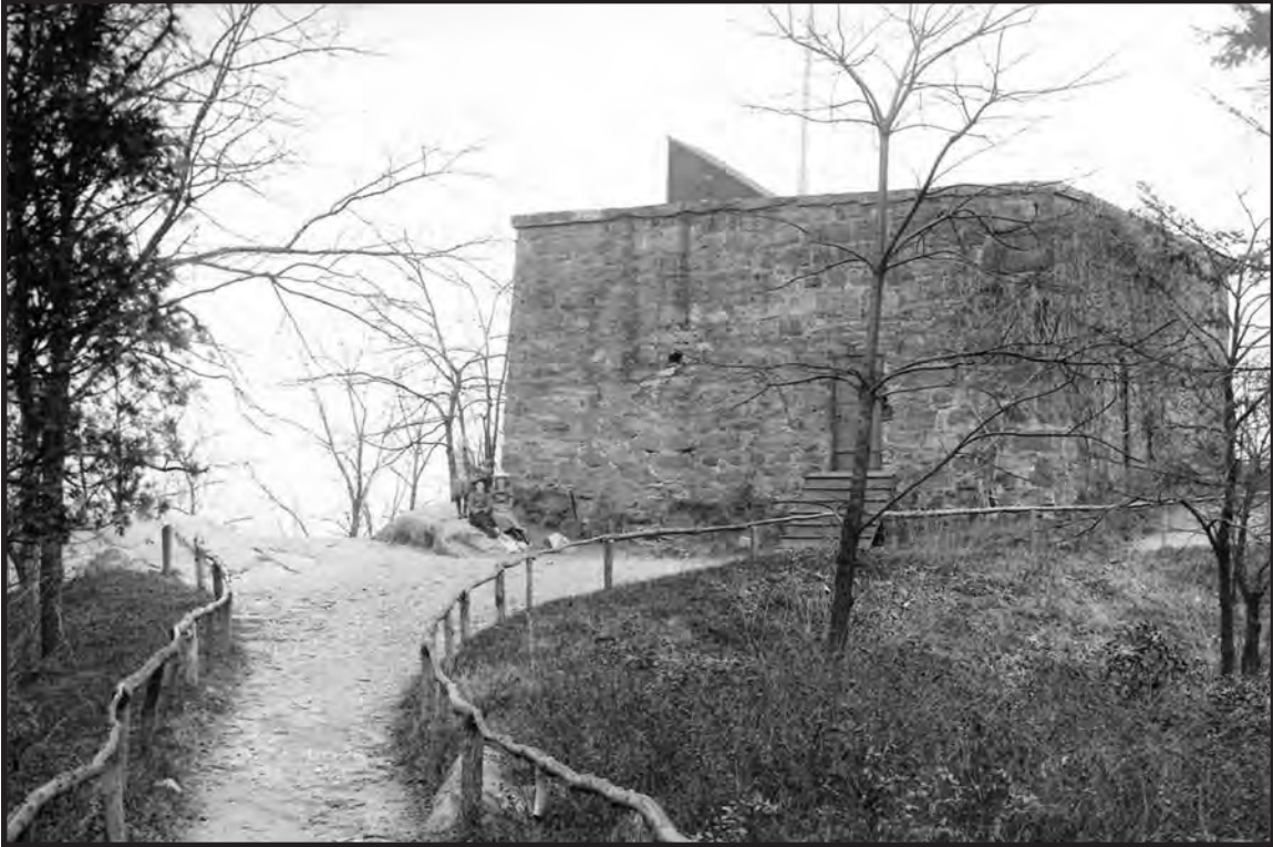
Photograph 2.6. Historic view looking east northeast, 1904. Note flagpole in northeast corner of the building, interior stairway hood along west wall, restored masonry, embrasures and parapet, and wooden exterior stair leading up to iron door. Source: Unknown Photographer (New-York Historical Society, R.S. Guernsey Lecture 20592).
