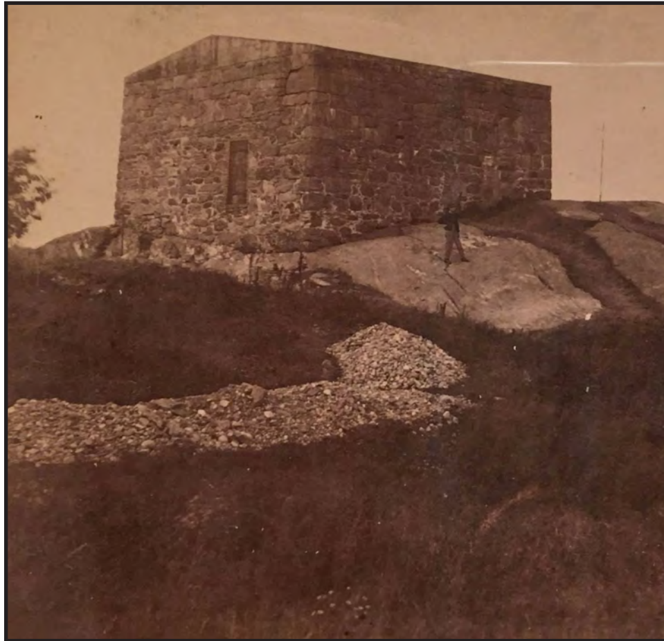
Photograph 2.2. Historic view looking northeast, circa 1865. Note shallow pedimented roof, blocked embrasures, iron door and absence of stair. The blockhouse at this time may still have been in use as a magazine for storing gunpowder. Source: E. and H.T. Anthony and Company, Stereographic View No. 1898 (Metropolitan Museum of Art, Herbert Mitchell Collection 2007.457.71).
