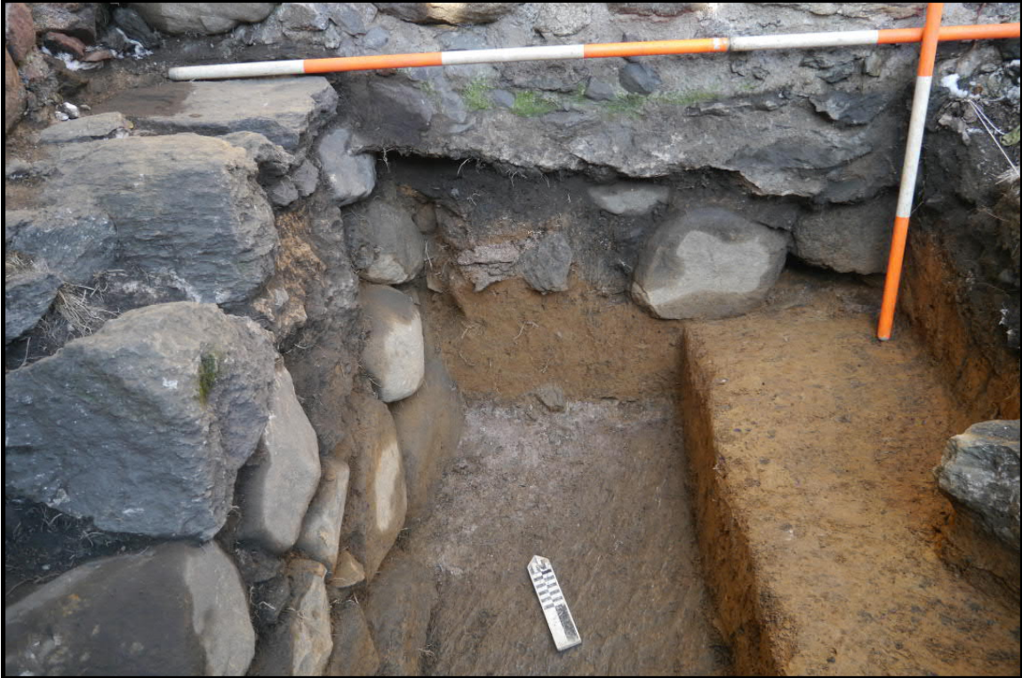
Photograph 4.17. View facing north showing the north profile of Excavation Unit 4. Note the mortar between the bedrock and clay fill; scales in feet and tenths of feet (Photographer: James Lee, December 2017 [HRI Neg.#17070/D1:210]).
