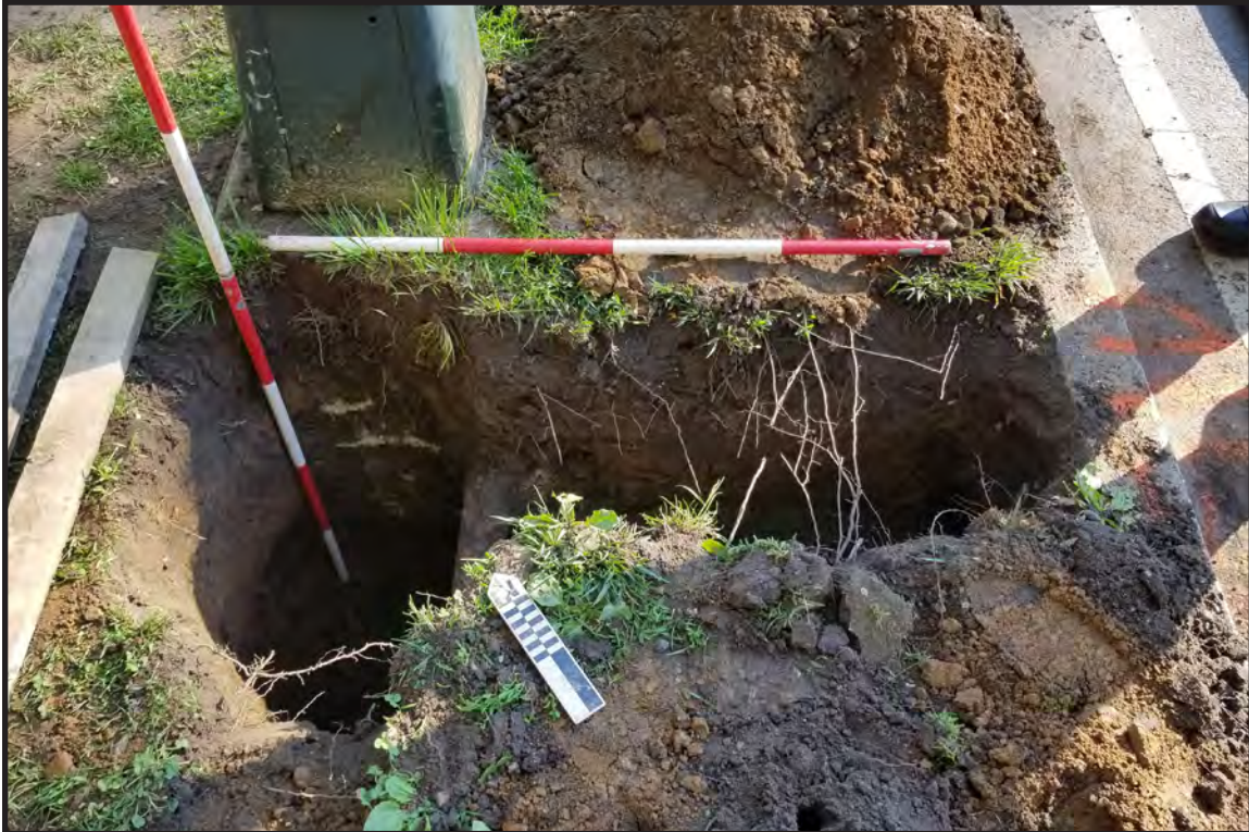
Photograph B.3. View facing northeast showing completed excavation of SLF #1 (Photographer: Joshua Butchko, May 2021 [HRI Neg.#21036/D1:001]).
