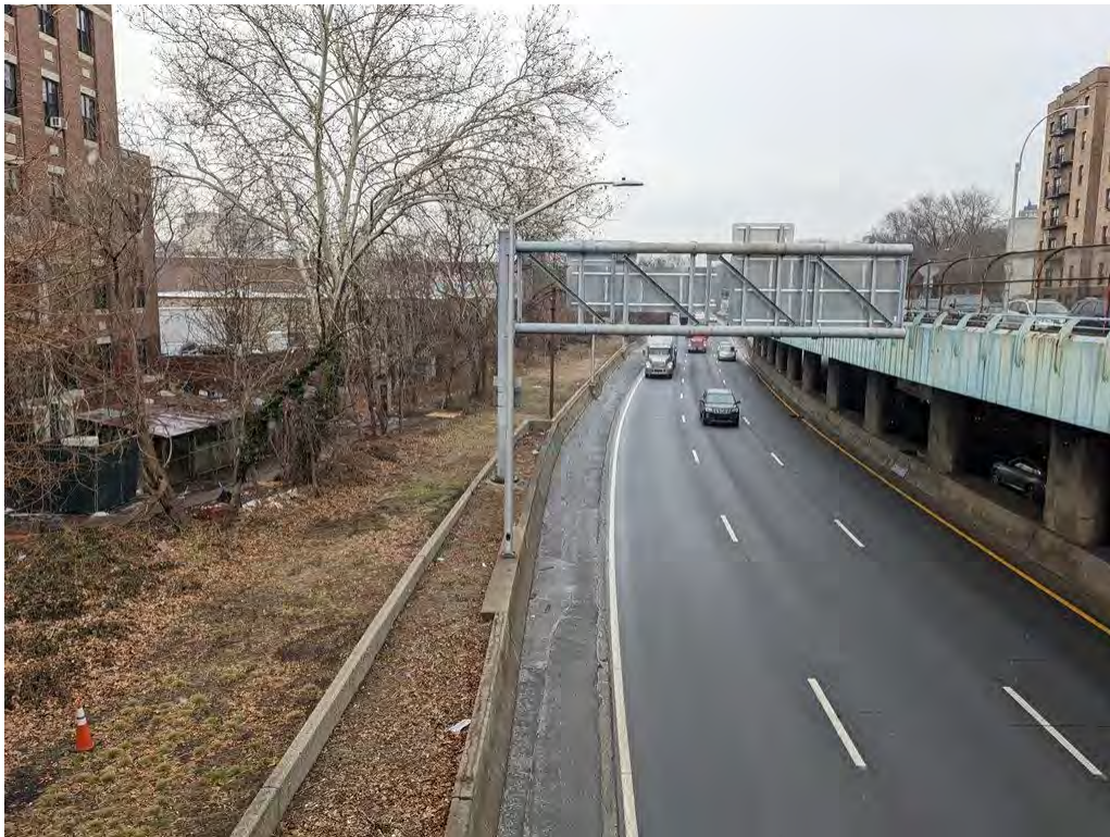
Photograph 22. The CSX-owned portion of the APE, looking northeast from West 231 st Street.
