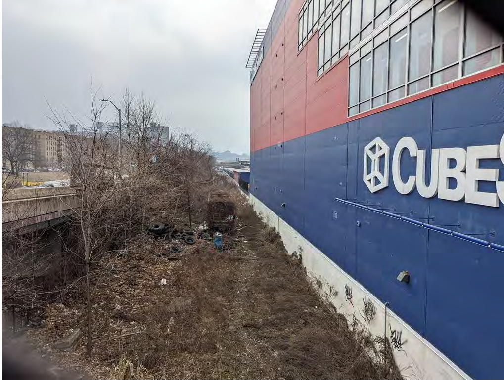
Photograph 25. The MTA Metro-North-owned portion of the APE, looking southwest from West 230 th Street. The proposed underground conduit would be located nearest the Interstate 87 overpass on the left.
