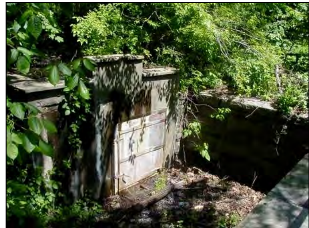
Putnam Trail, pump house foundation, looking northwest
