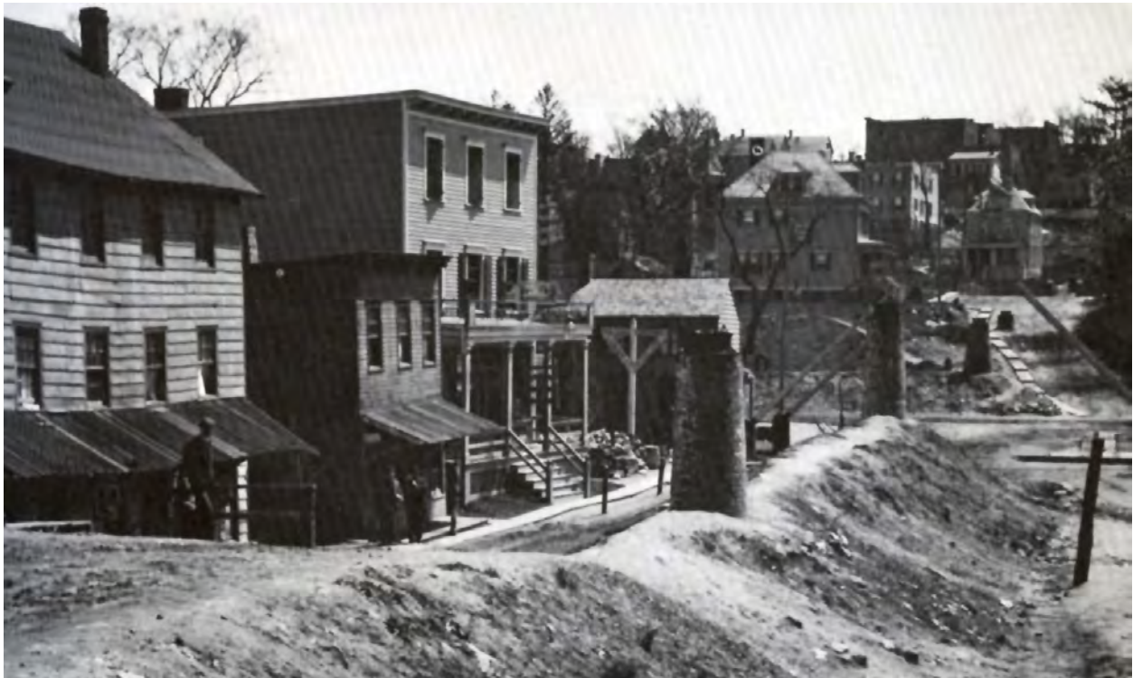
1909 view of the project site in the right background at West 231 st Street as the road was being prepared to be raised. The manhole columns indicate the roadway's present height. Courtesy Kingsbridge Historical Society Archives.
