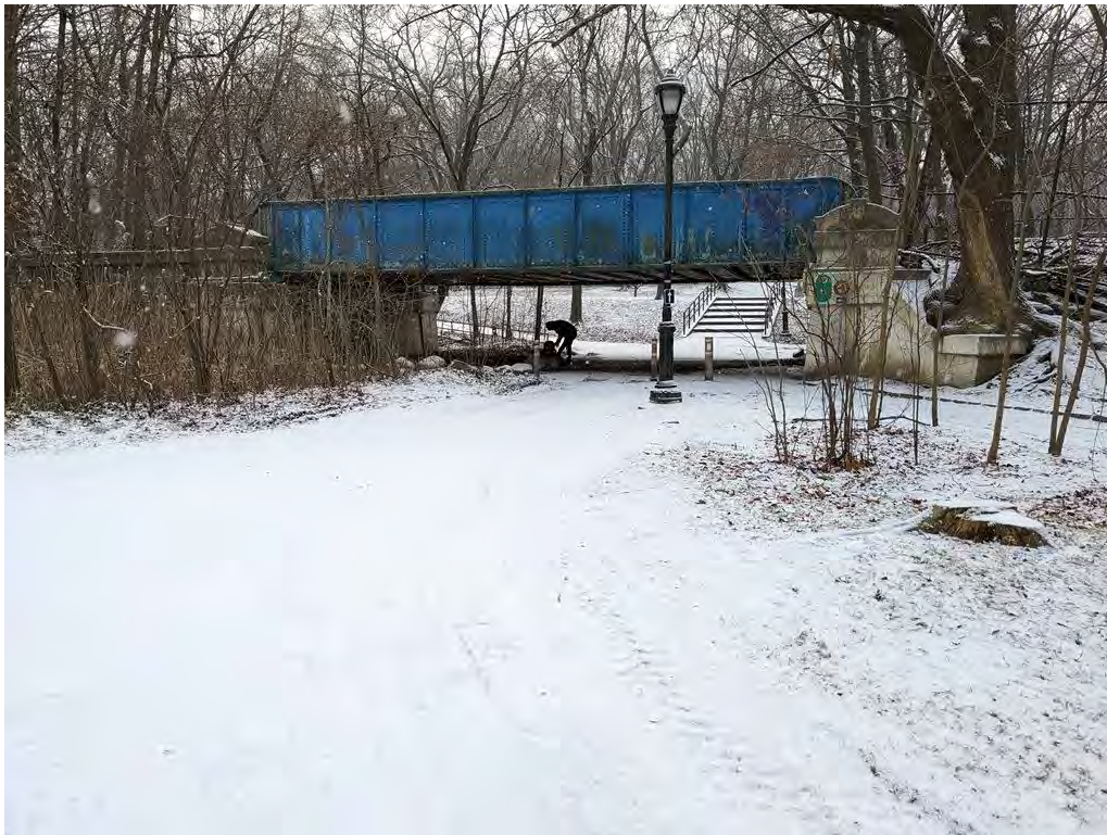
Photograph 8. The APE showing the 1904 railroad bridge carrying the Old Putnam Trail. View looking southeast.
