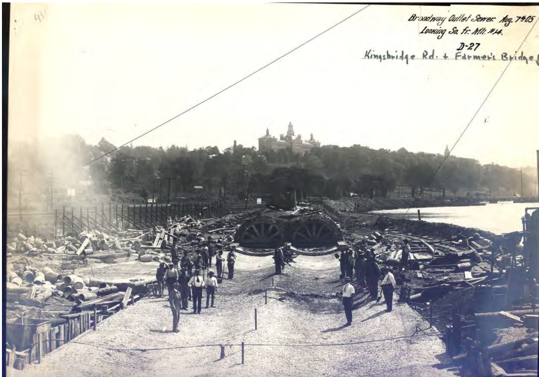
1905 view of the Broadway sewer outlet. The project site is in the far background. Courtesy City of New York Department of Sewers.
