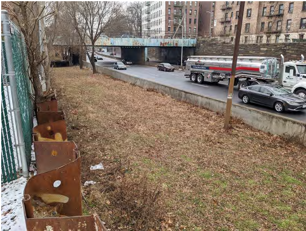
Photograph 16. The CSX-owned portion of the APE, looking northeast toward the West 238 th Street overpass.
