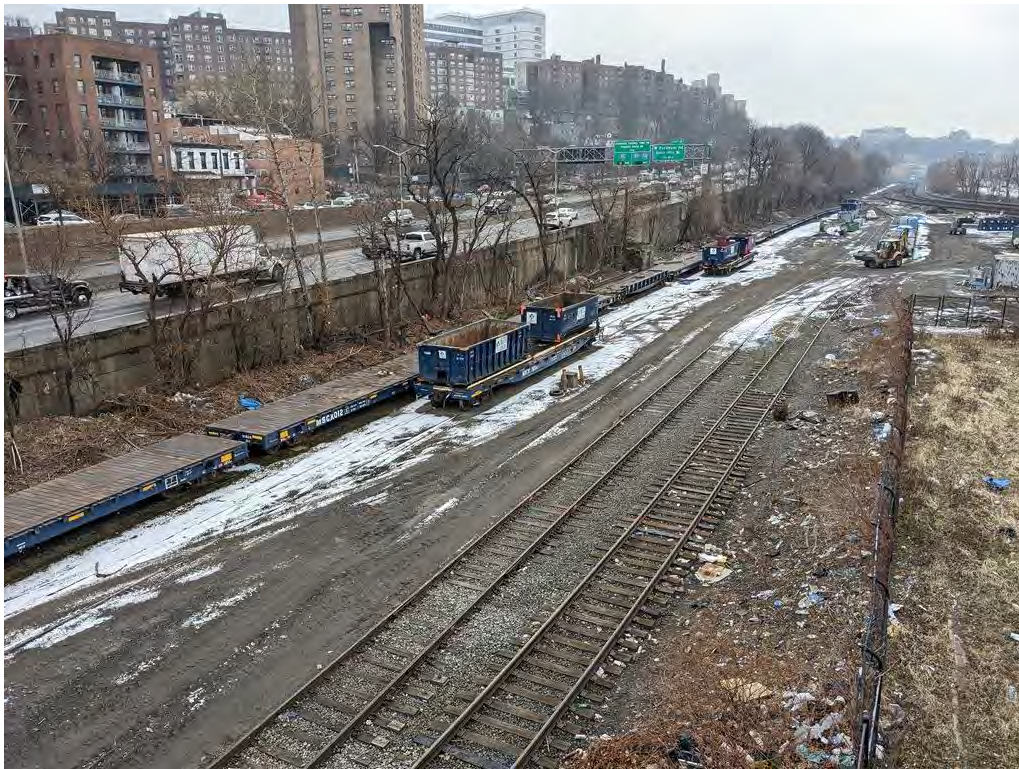
Photograph 28. The MTA Metro-North-owned portion of the APE, looking south from south of West 225 th Street. The proposed underground conduit would be located between the railroad tracks and Interstate 87.
