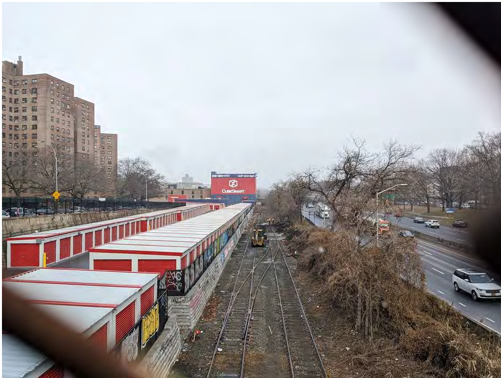
Photograph 26. The MTA Metro-North-owned portion of the APE, looking northeast from West 225 th Street. The proposed underground conduit would be located to the right of the railroad tracks.
