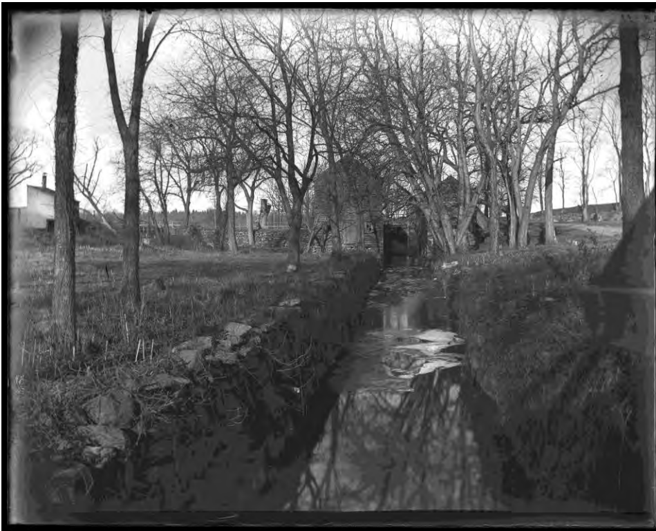
Circa. 1900. Former mills and mill race on the southern side of the Van Cortlandt Lake dam. The railroad tracks are on the far right. Courtesy New-York Historical Society.
