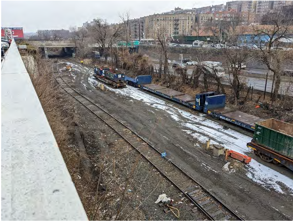
Photograph 27. The MTA Metro-North-owned portion of the APE, looking northeast towards West 225 th Street overpass. The proposed underground conduit would be located between the railroad tracks and Interstate 87.
