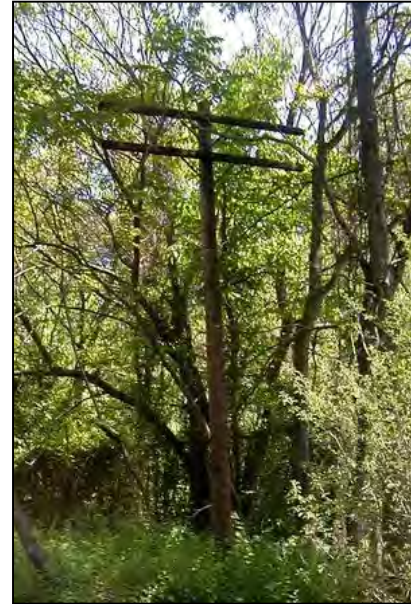
Putnam Trail, wood electric pole, looking northwest
