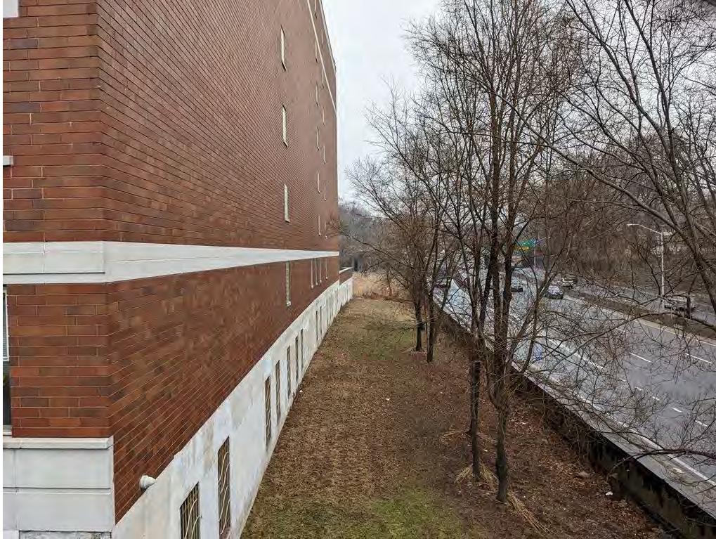
Photograph 15. The CSX-owned portion of the APE, looking northeast from West 238 th Street.
