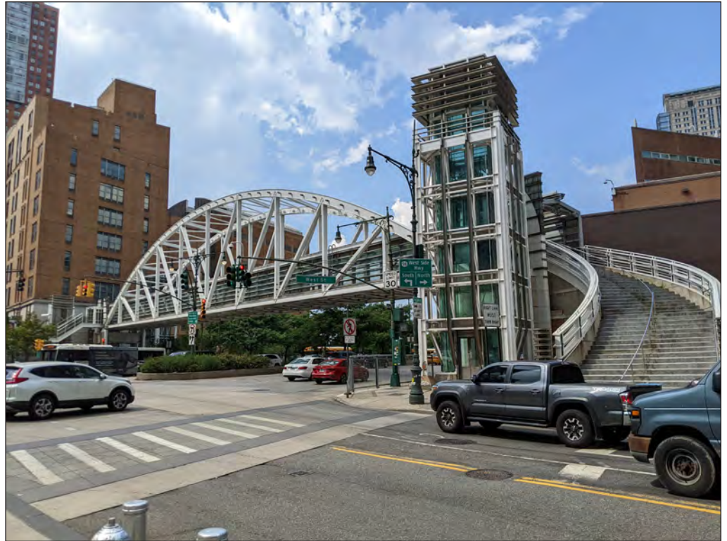
Chambers Street pedestrian bridge, view northwest on Chambers Street 3
