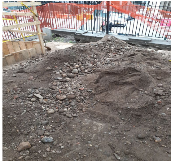
Photo 27. TP is in the upper left corner with screened soil from c. 9.5 ft. (3.0 m) bgs in the foreground. The rocks and stones were discards during screening. (S. Spritzer 10/7/2020)
