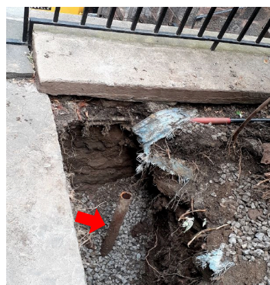
Photo 34 (left). The SW Light Pole Pit looking east after excavation. An electrical pipe (arrow) was exposed just under the surface. (S. Spritzer 4/19/2021)
