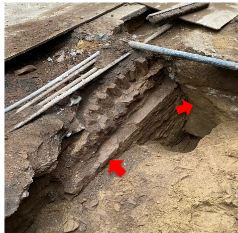
Photo 20. East end of an unidentified vault exposed in the west wall of the Broadway Trench (left arrow). Part of a flagpole base (right arrow) is also exposed (R. Fiore 12/2/2020)
