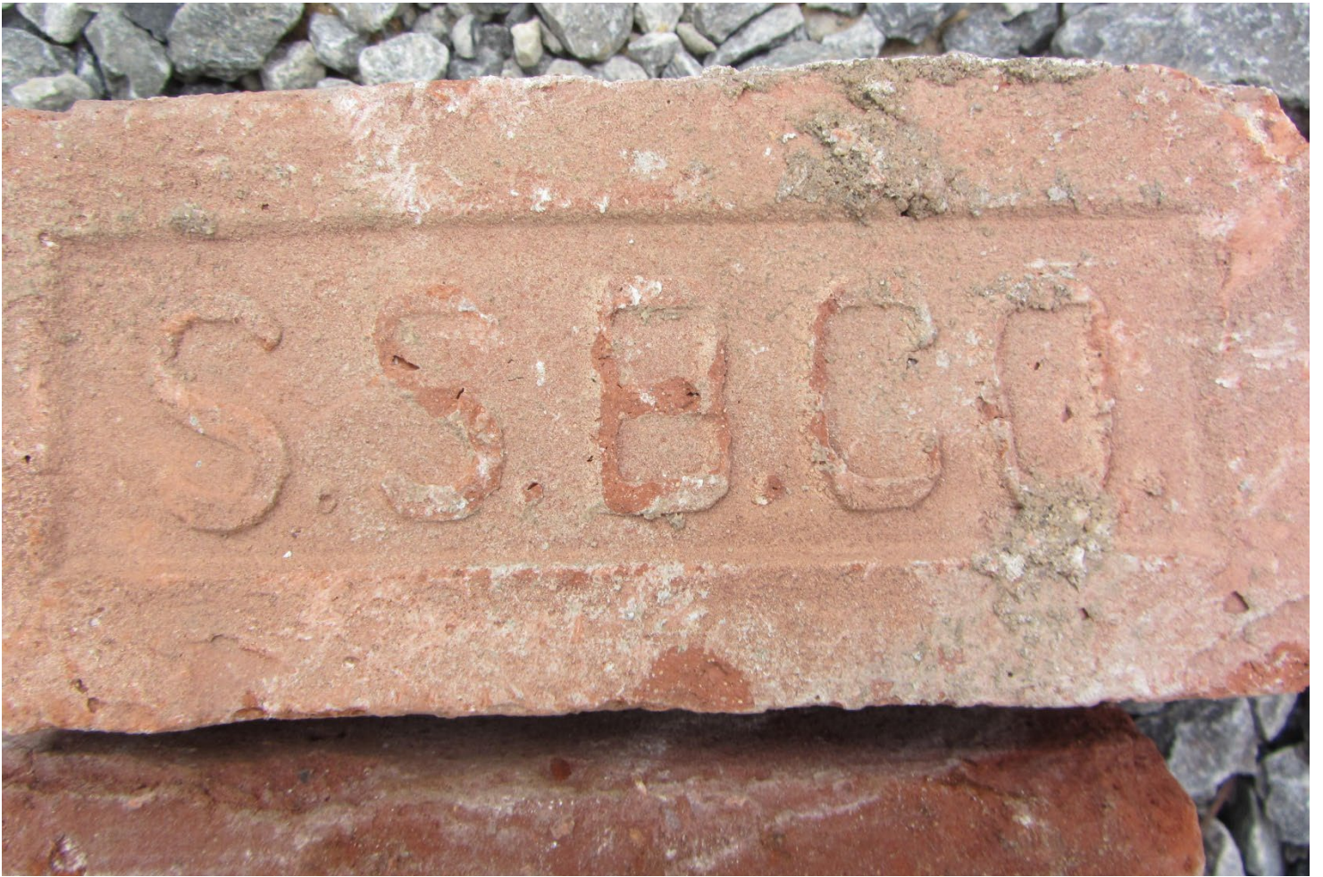
Photograph 19: Representative brick removed from interior wall of Vault C.
