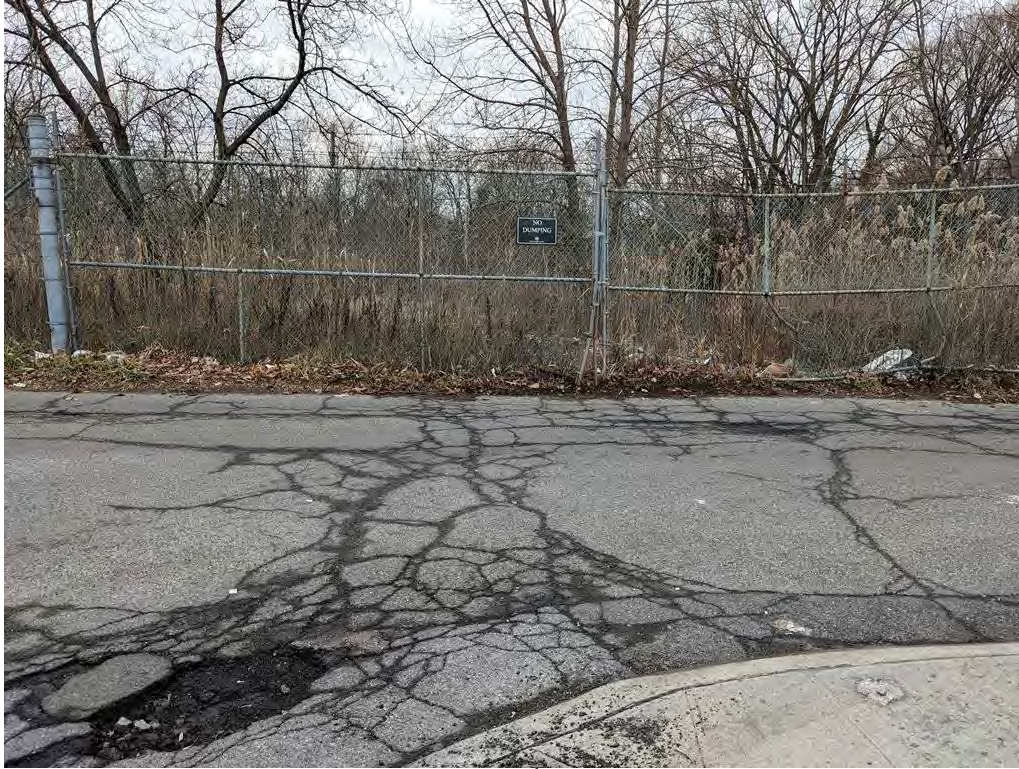
Photograph 37. BMP #1gated entrance from 235 th Street. View looking northwest.
