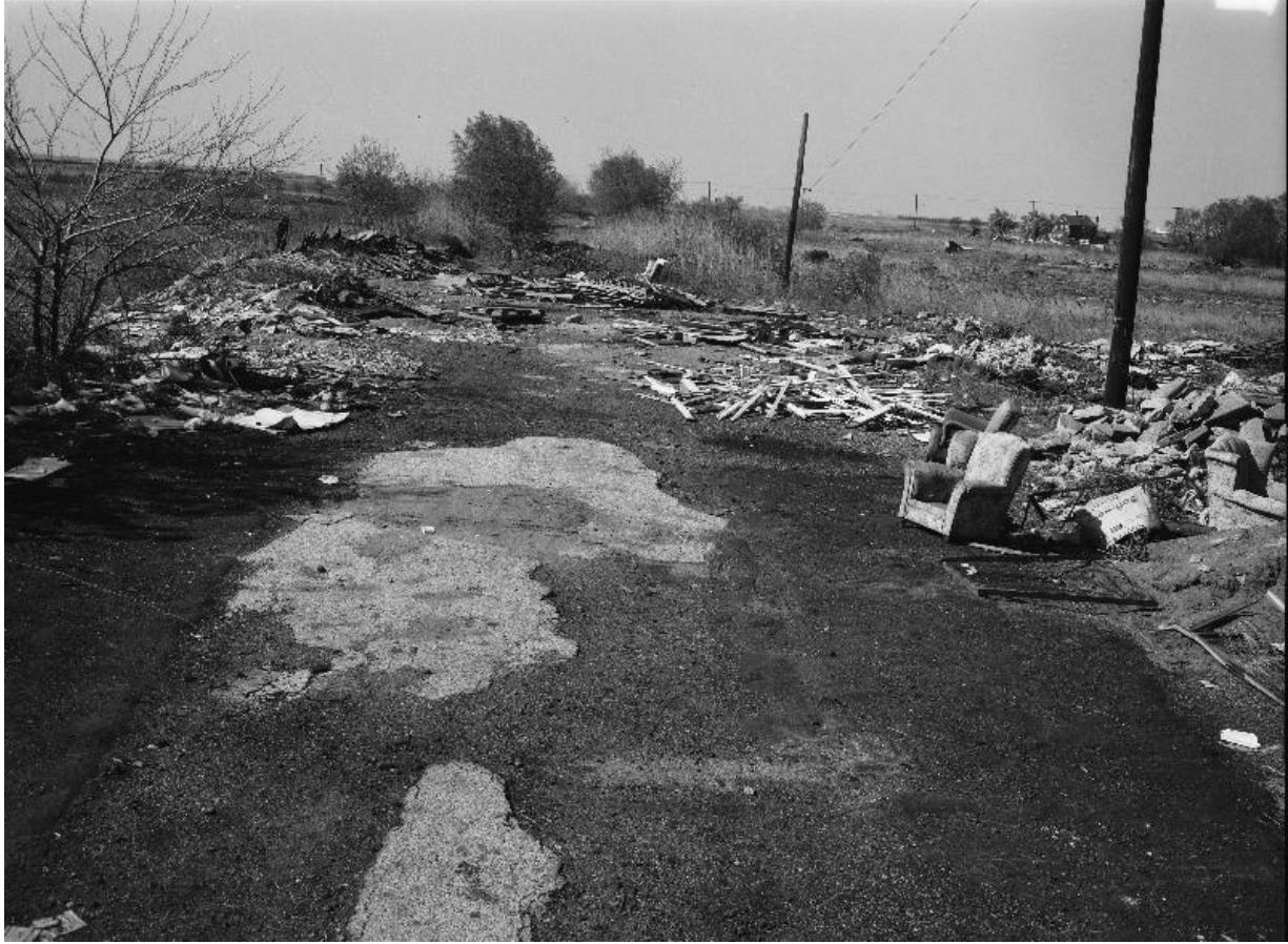
32472_9_Q008_05-11-1966_Brookville Park, Dumping
