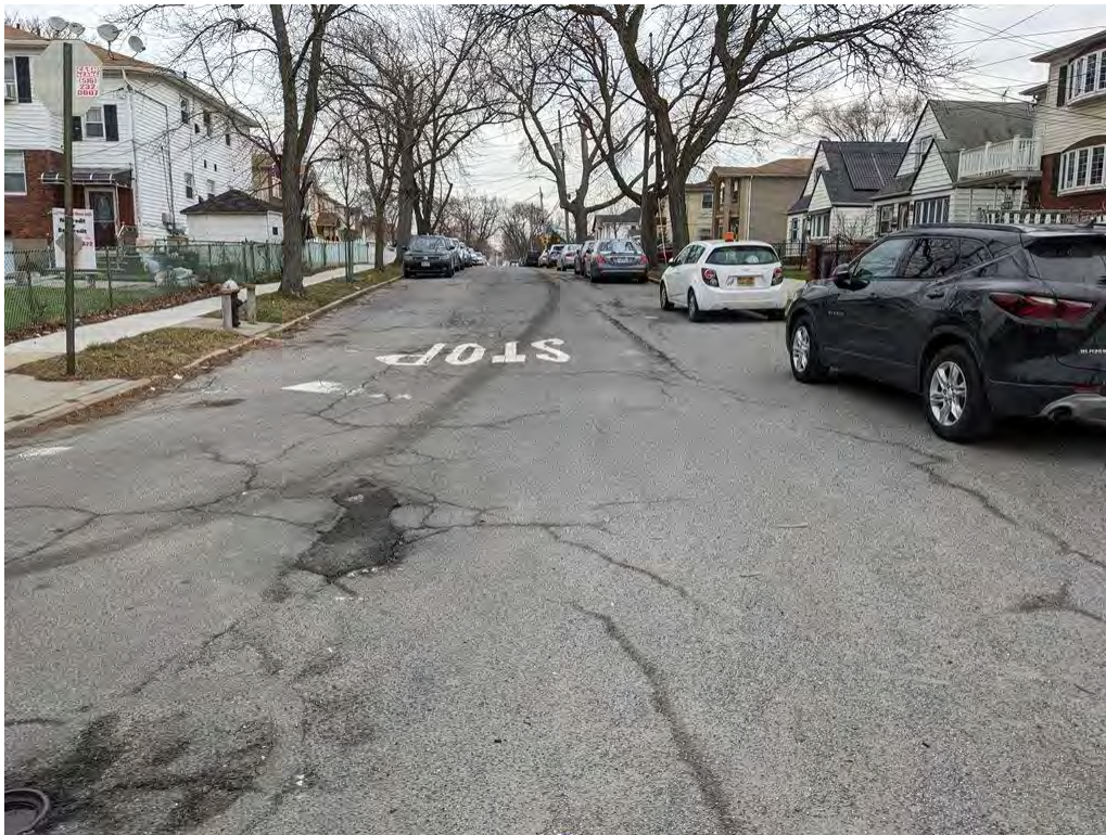
Photograph 10. 148 th Avenue looking east from Brookville Boulevard.
