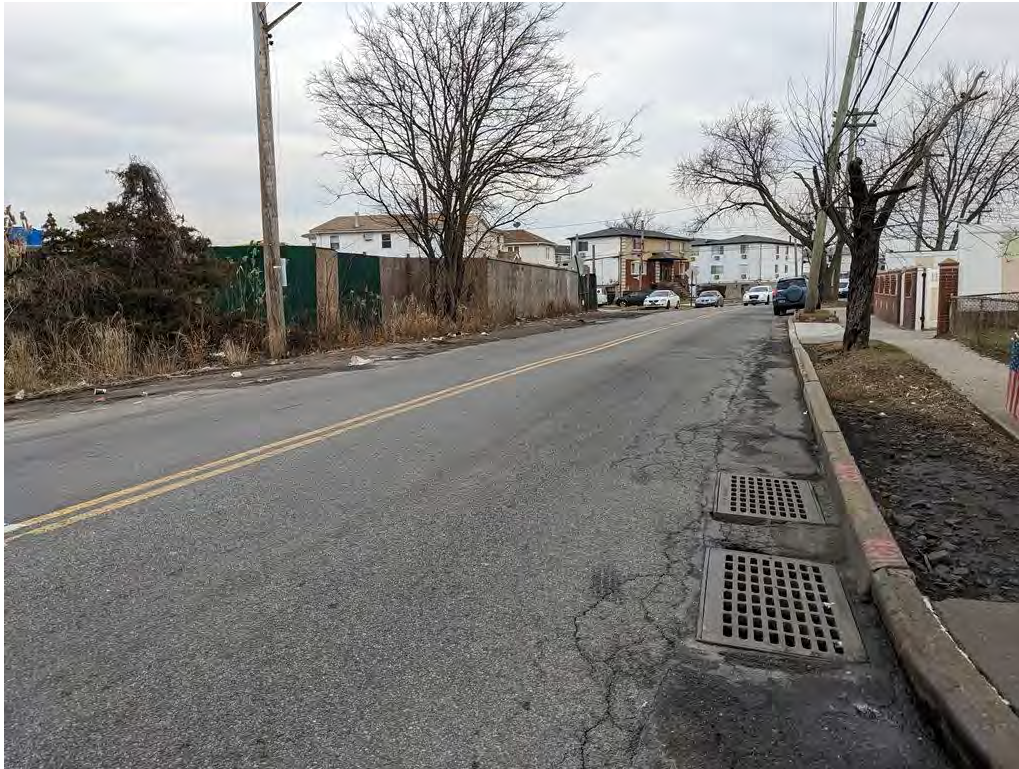
Photograph 1. Brookville Boulevard looking north from the intersection of 149 th Avenue.
