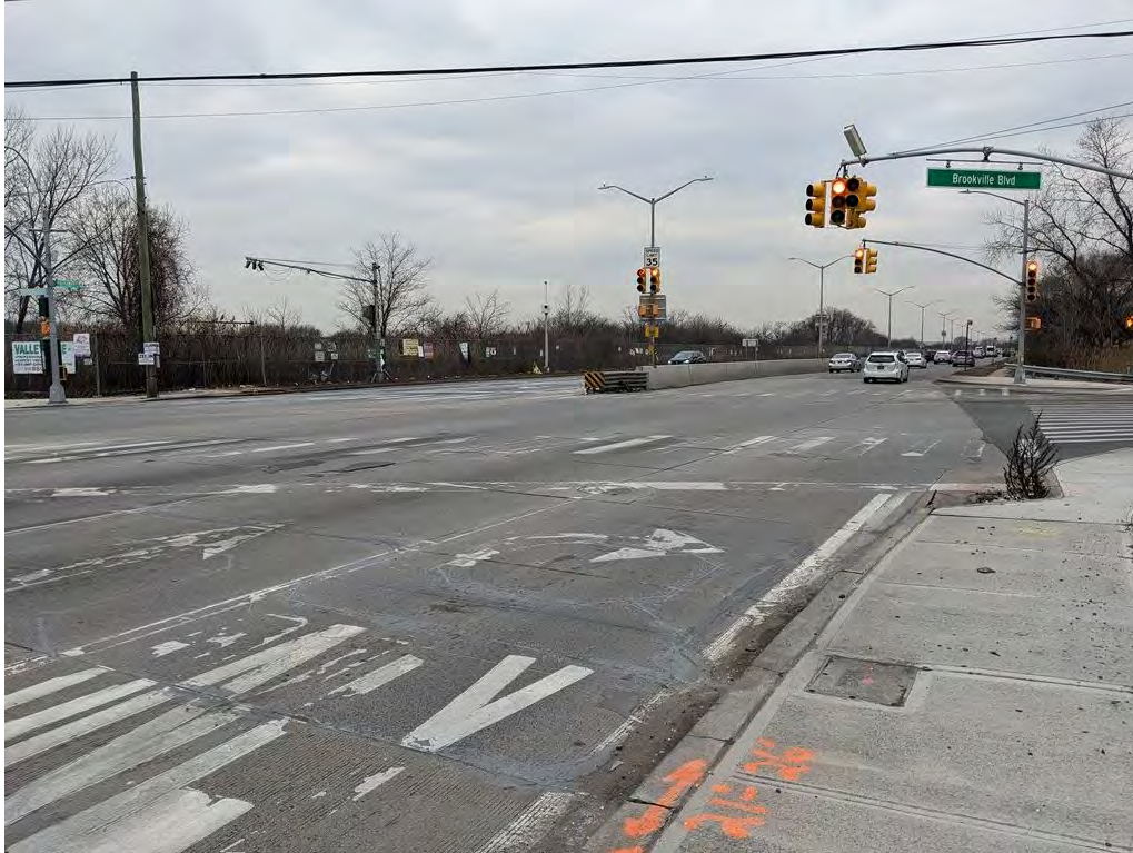
Photograph 35. Brookville Boulevard and Rockaway Boulevard intersection. View looking northwest.
