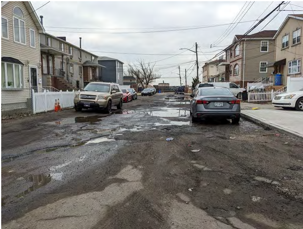
Photograph 18. 236 th Street looking southwest from Bentley Road.
