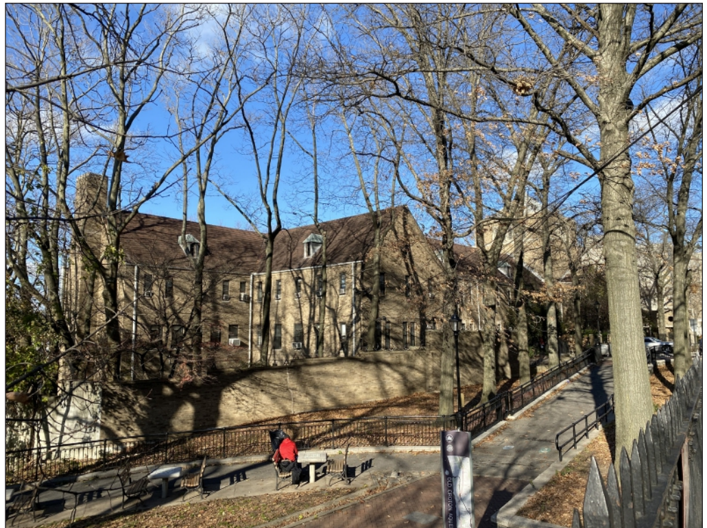
Looking north at the former convent from Highbridge Park, showing the steep grade change to the west (left) and the retaining wall lining the south of the Project Site 2
