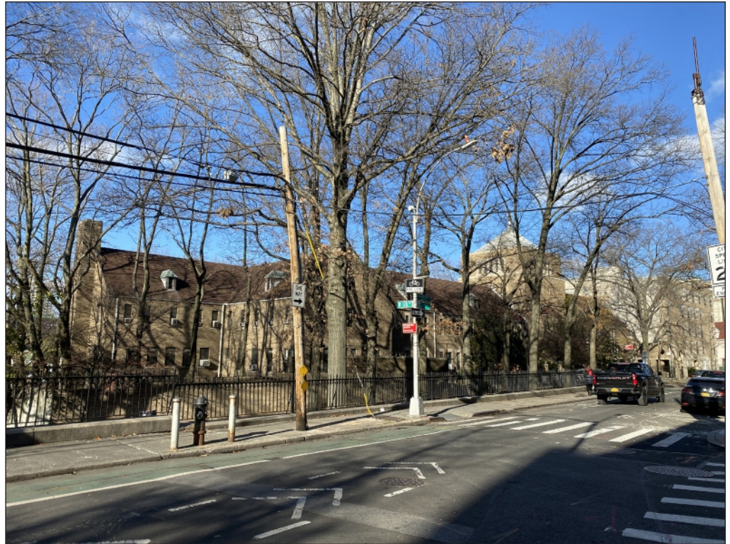
View of the former convent looking northwest from University Avenue 1
