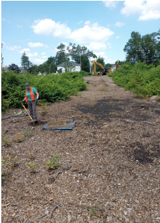
7. ST8 during excavation, facing north.
