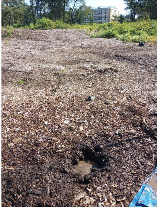
3. Water-filled ST1, facing east.
