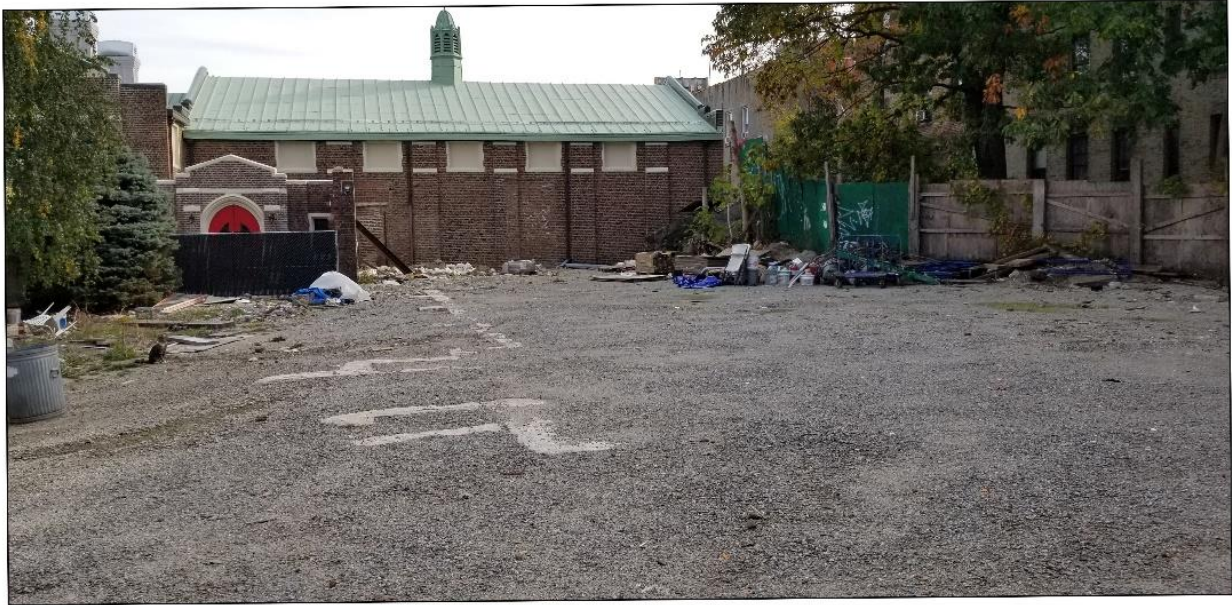
Fig. 6. View of Lot 16 of the project site looking southeast towards the parish hall
