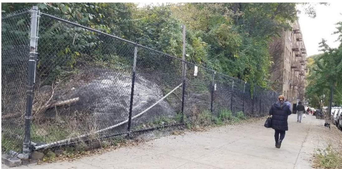
Fig. 5. View of the Seaman Avenue side of the project site to Dyckman Street from the corner of Cumming Street
