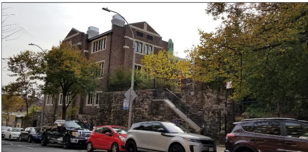
Fig. 4. View of the Parish Hall from Cumming Street
