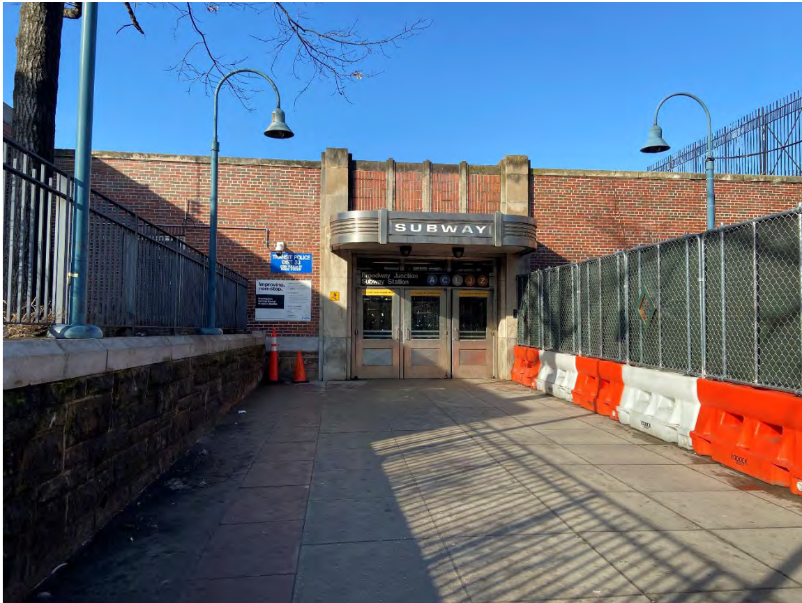
Photograph 1: Facing west from Van Sinderen Avenue to the station entrance at the Control House for the A, C, E, J, and Z Subway lines.
