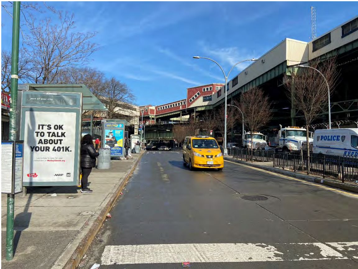
Photograph 4: Facing north from the west side of Van Sinderen Avenue to the location of the proposed new elevated A/C to L transfer bridge. Elevated A/C Line at right.
