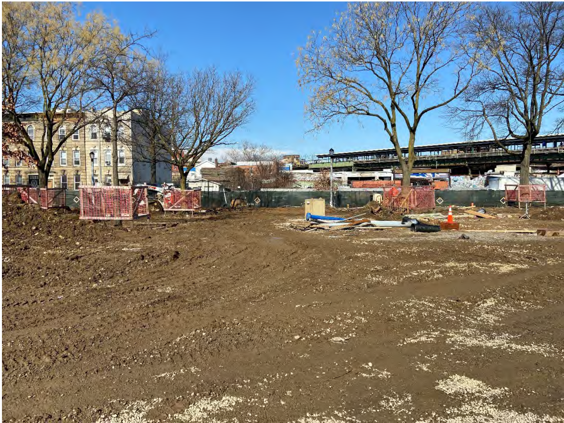
Photograph 9: Facing north to Truxton Street from Callahan-Kelly Playground while under construction.
