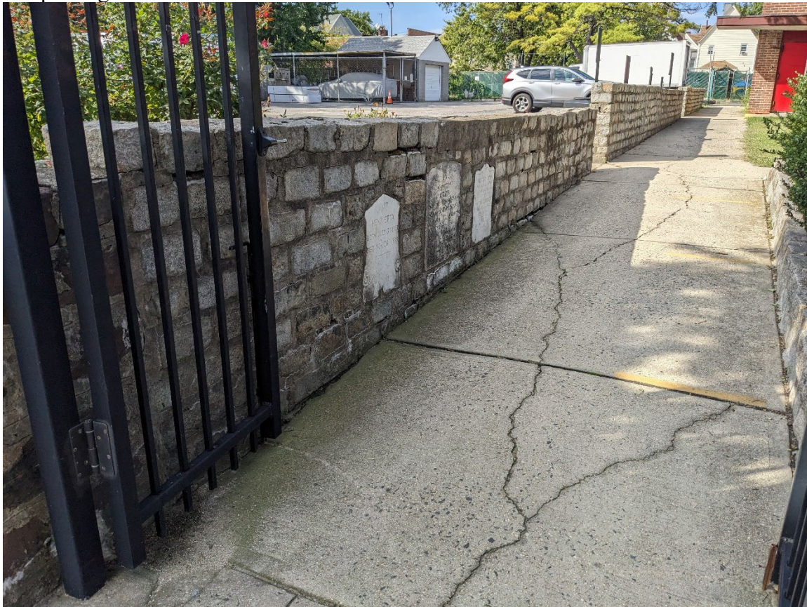
Photograph 7: Facing northwest from East Tremont Avenue to sidewalk and wall between the church yard and the parking lot to the west (left), with three headstones from the former cemetery embedded.
