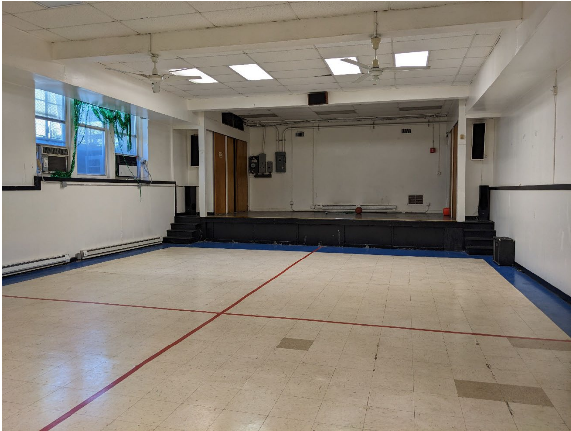
Photograph 24: Inside the Westchester United Methodist Church basement auditorium with deep window wells visible at left. This level was constructed in 1913 and served as the meeting space until the upper levels were built ca. 1948.
