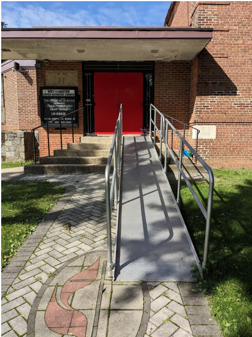
Photograph 3: Facing north to main church entrance from yard to south of church.
