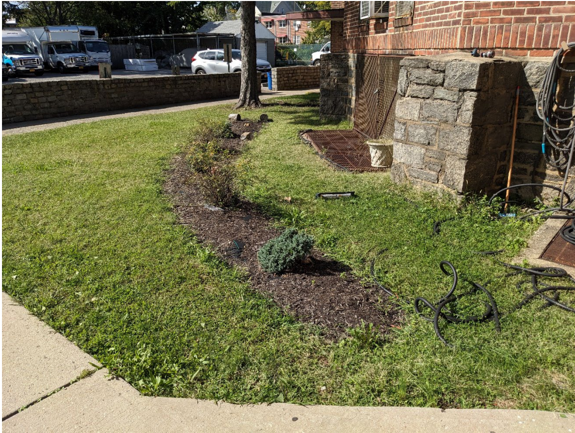
Photograph 4: Facing northwest from sidewalk to south of church to garden plantings and deep window wells.
