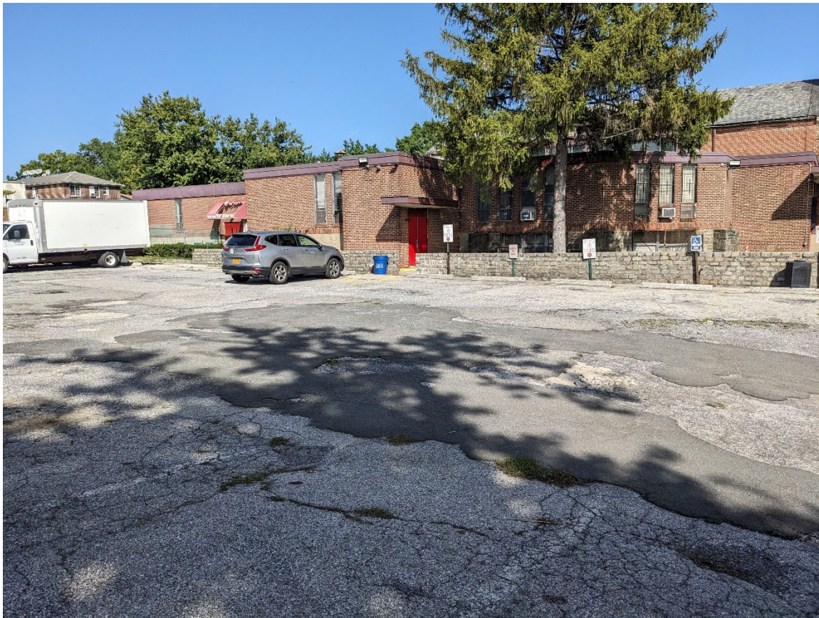
Photograph 11: Facing northeast from southwest end of parking lot to church with additions to the left (north).
