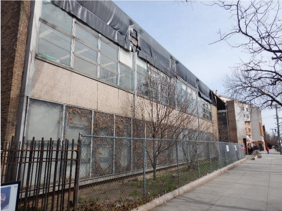
Photo 4. View facing south side of New Lots Library.
