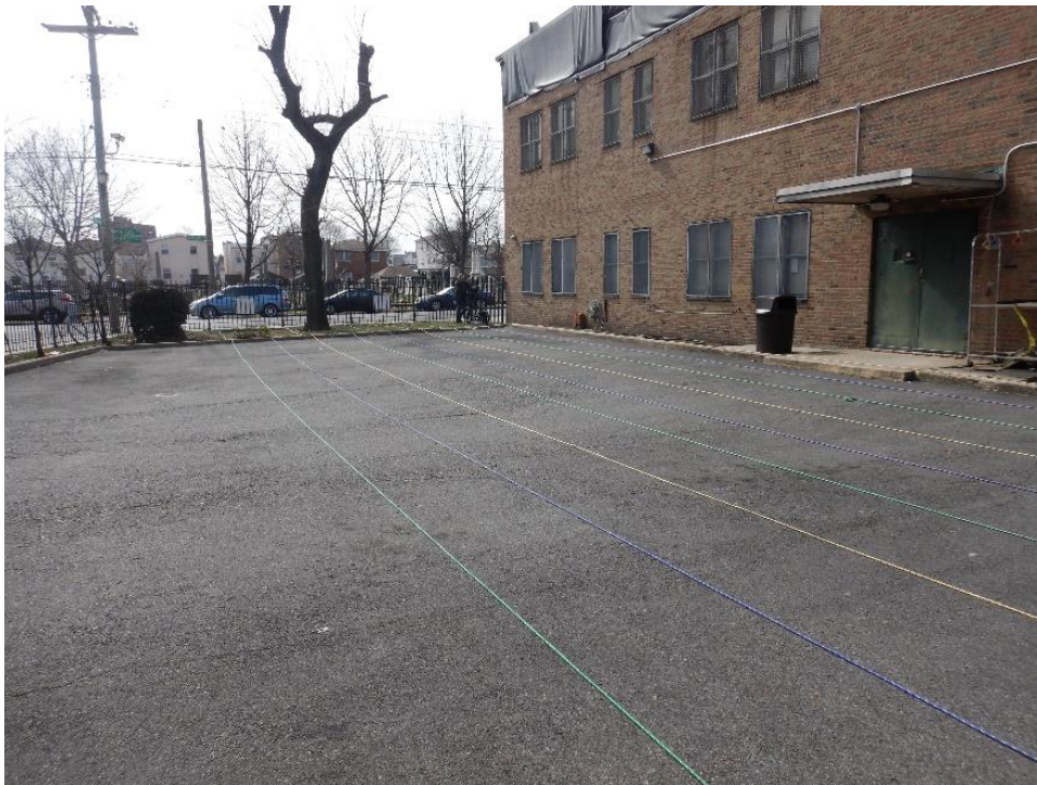
Photo 10. GPR transects on the east parking lot.
