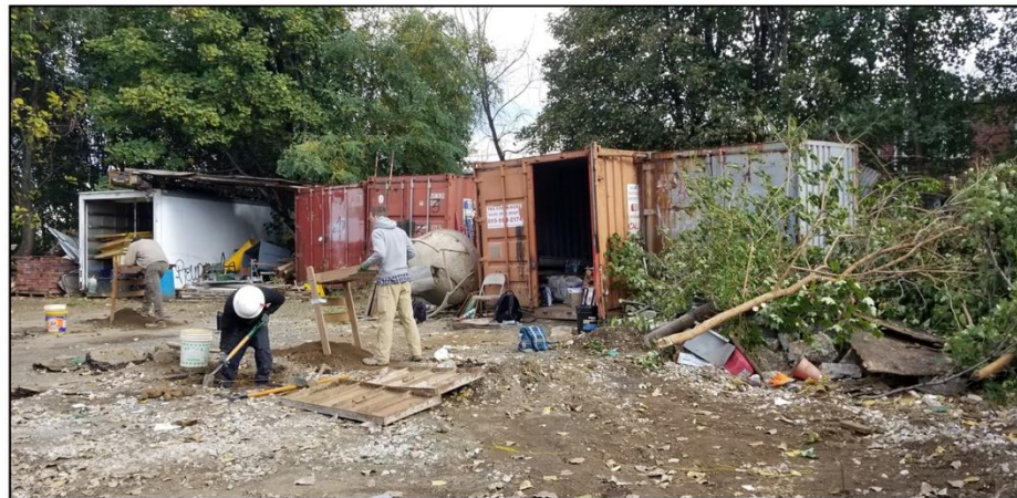
Fig. 9. (top) AREA H – View from the southeast side of the site looking west, with the 8 th Street easement in the center. The area on the opposite side of the easement seen in this view is not part of the project site. TR 38 and TR 37 are in the foreground and TR 34 and TR 33 behind them. TR 32 has been backfilled.
