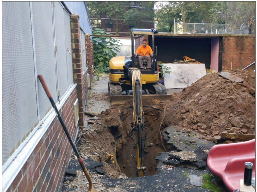
Facing southeast from back of 1-story building showing excavation of Trench 1. 6 Note loose brown urban fill with demolition debris
