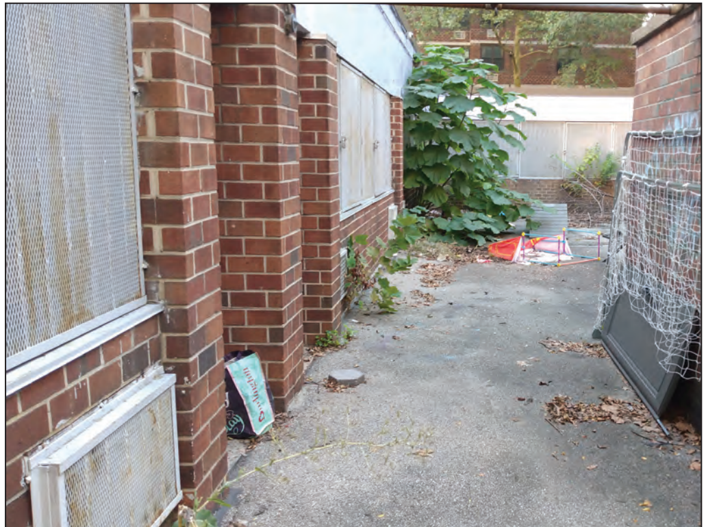
Facing east along back of 1-story building showing location of Trench 3. 4 Note brick storage/utility structure on the right
