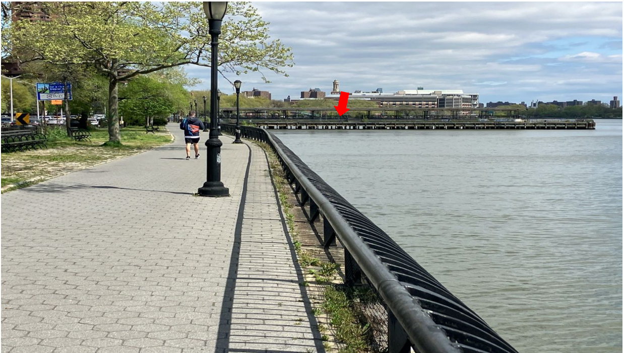
Photo 3. View north on the APE with the 107 th Street Recreational Bridge that defines the north limit of this section of the APE in the background (arrow). The walkway in this area is quite wide. Northbound traffic on the FDR is visible in the center left background. (Photo: J. Geismar 4/19/2023)
