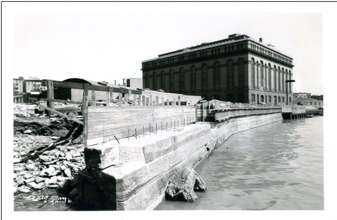
Photo 10. View N from point on a barge between E 94 and 95 Sts. Showing detailed view of original granite bulkhead, top course removed and top facing forms in place. (No. 2728 6-22-1936)
