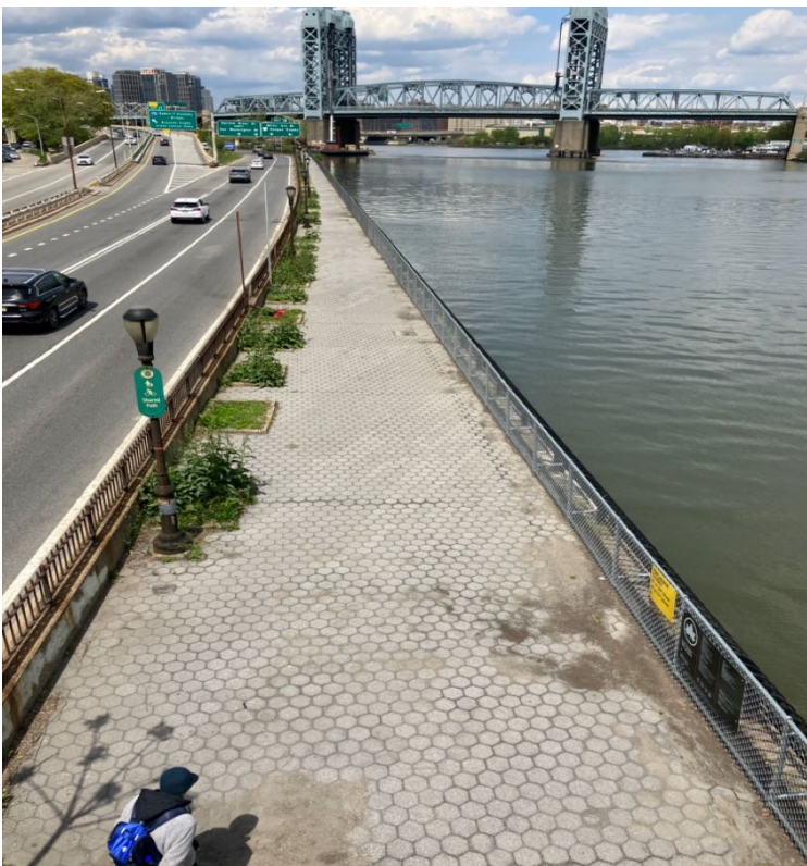
Photo 5. View north from the 120th Street pedestrian bridge access to the walkway (APE). The northbound FDR lanes (those on the right) lead to the Harlem River Drive; the one that branches off to the left is the access to the RFK-Triborough Bridge. The walkway is somewhat wider here than it is south of the pedestrian bridge but with little vegetation. (Photo: J. Geismar 4/25/2023)
