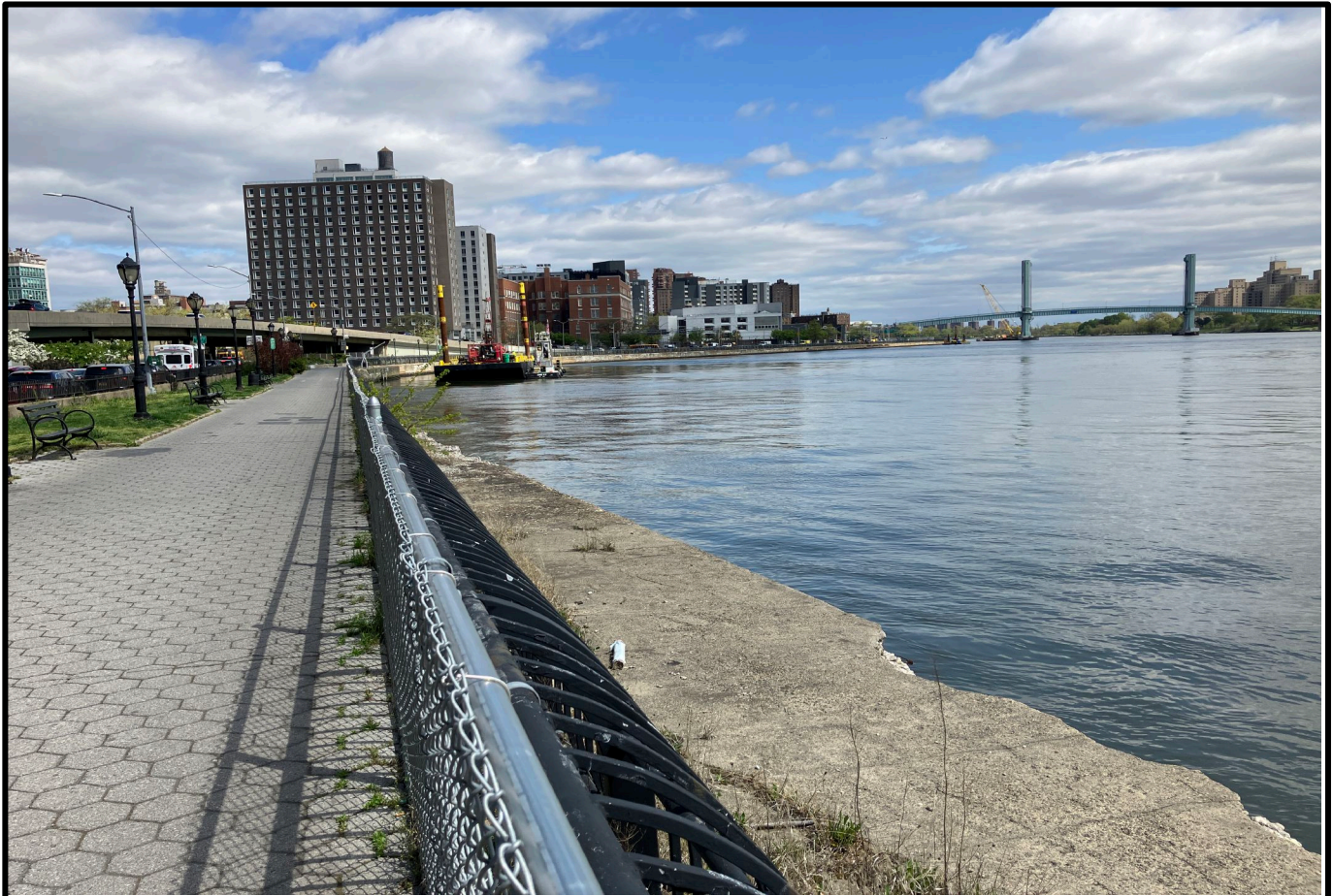
Bobby Wagner Walk (archaeological APE) looking N near 95 th Street and the East River with concrete topped seawall (bottom right) and the 103 rd Street Pedestrian Bridge to Wards Island (right background). (photo: J. Geismar 4-19-2023)
