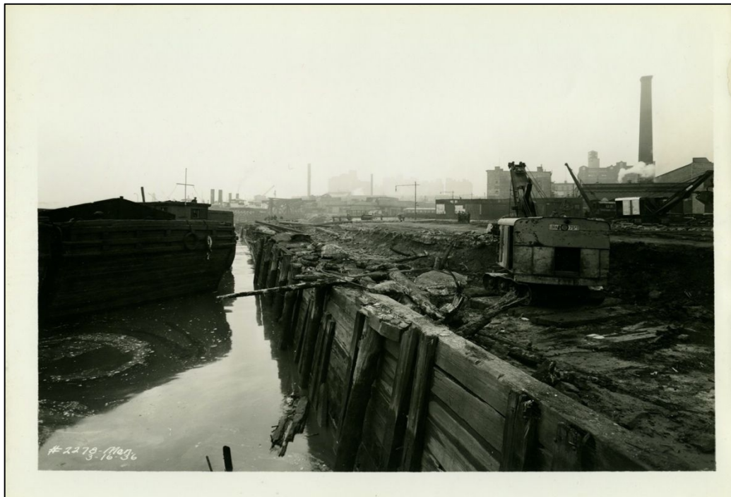
Photo 7. East River Drive. View south from pier off E 94 th Street showing excavation in back of [timber] bulkhead S of E 94 th Street. (No. 2278 3-16-1936).
