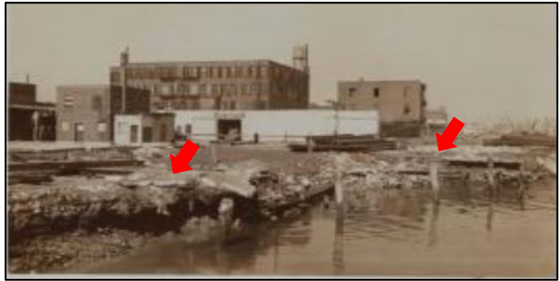
Photo 6. View north from 100 th Street in 1936 showing crib bulkhead then in the APE. (Sperr 1936: NYPL Digital Collections)
