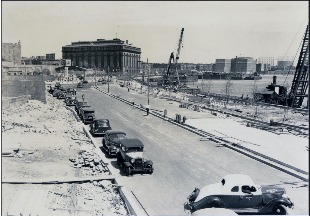
Photo 15. East River Drive and the adjacent park still under construction in May 1940 in the vicinity of the archaeological APE. The view is north from about 93 rd or 94 th Street. In the background is the Metropolitan Power House building on the block between 95 th and 96 th Streets. (Photo courtesy of the Municipal Archives: ID No. MAC_2407)
