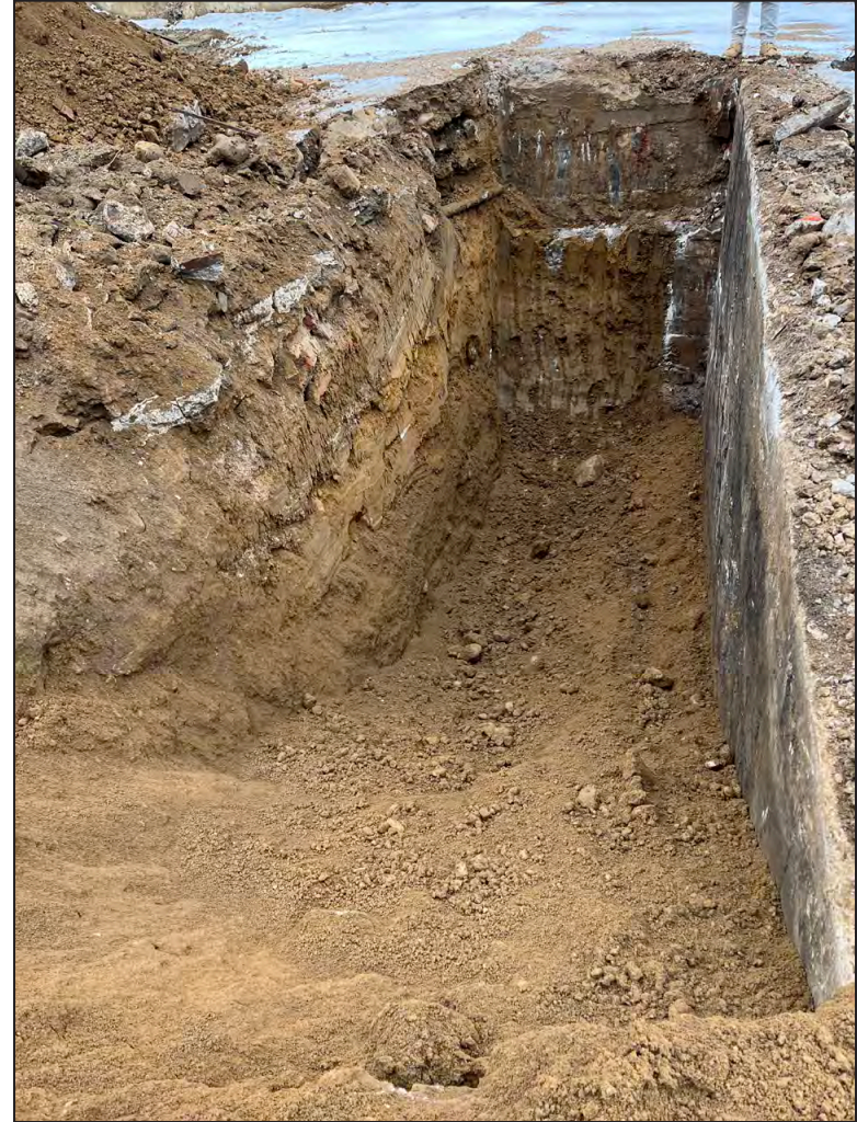
Looking in the opposite direction, showing more natural soils in the base of the excavation and along the western side 8
