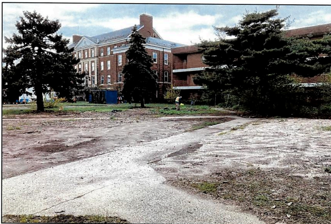
PHOTOGRAPH 13: Area Three, Showing Disturbed Sections of Building 513, View Southwest
