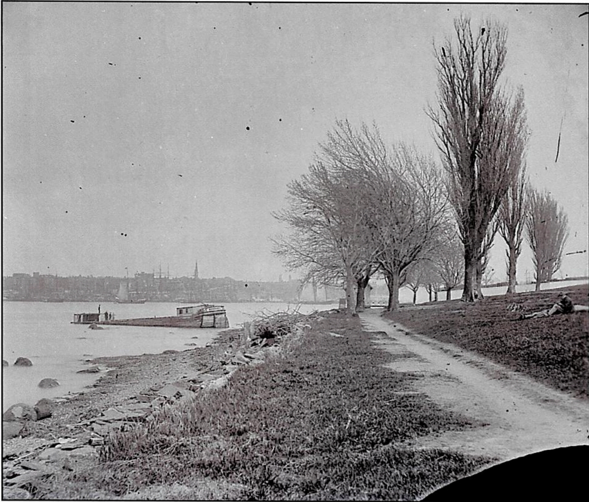
FIGURE 23: Photograph from ca. 1862, Showing Original Bluff of Governors Island's Northern Shoreline Reduced to Gentle Slope, and that a Track Road from the Wharf to Castle Williams Had Been Built. Sea wall ca. early 1800s visible as low stack of rocks against slope base, more of a rip-rap than a wall. (Brady 1861-1865, NAID 527660)
