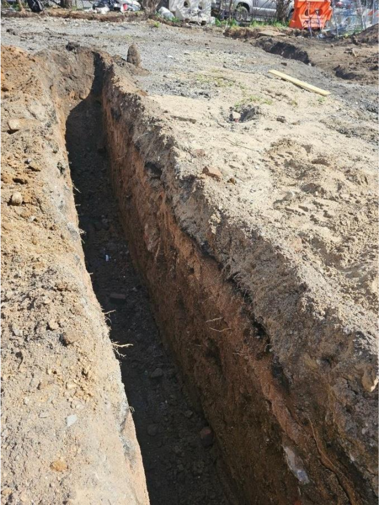
Image 6: Trench 2 – Looking east.
