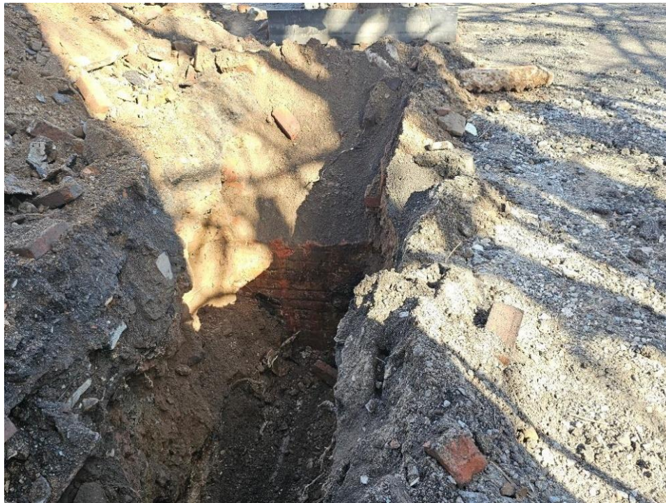
Image 9: Trench 3 – Remains of brick wall
