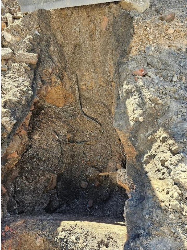
Image 10: Trench 3 – Metal “frames” within the trench.
