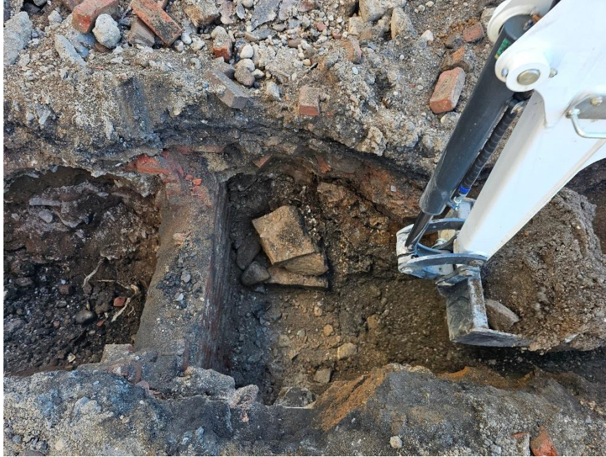
Image 8: Trench 3 – Remains of brick wall
