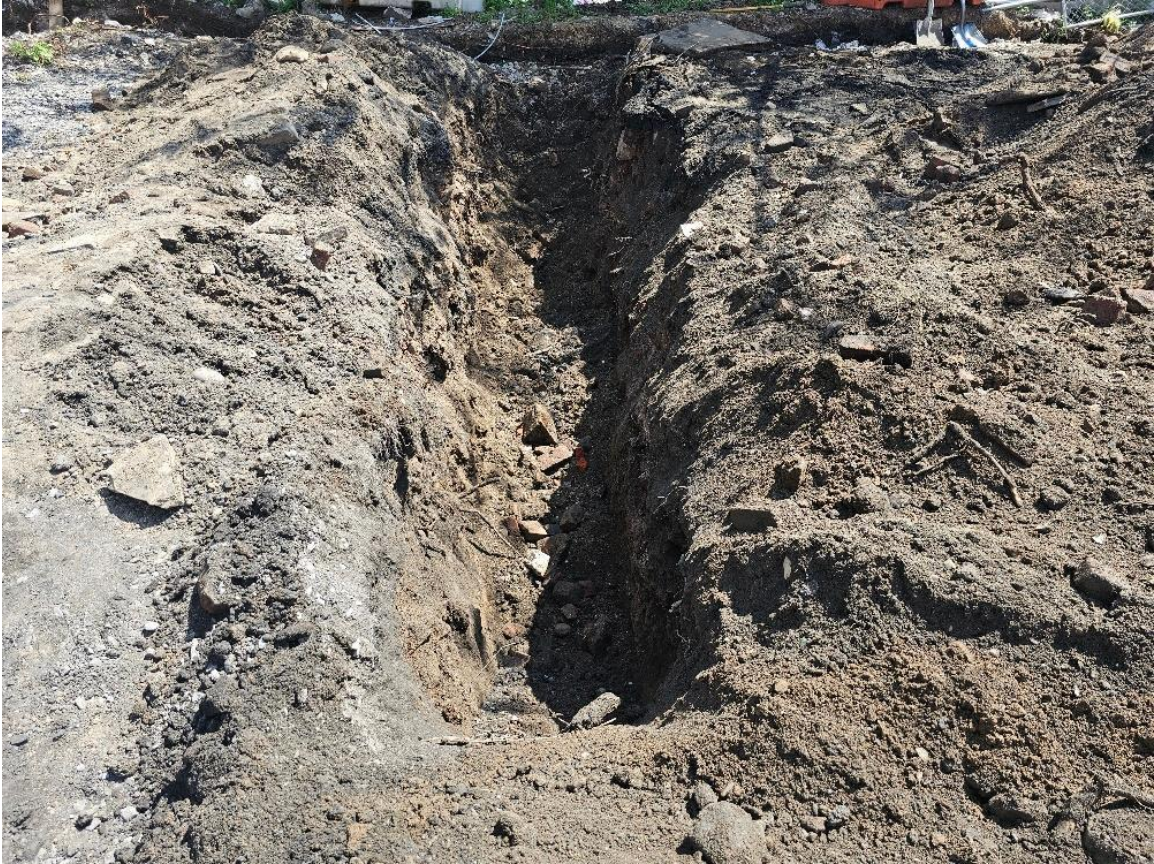
Image 5: Trench 1 – Looking East.
