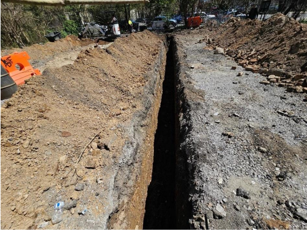
Image 13: Trench 4 -Looking east.
