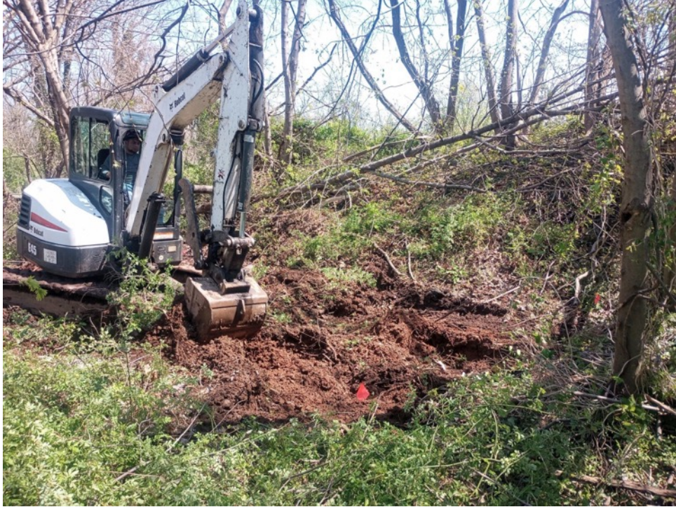
Photograph 7. Large fill pile directly southeast of Trench 2.
