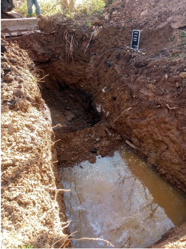
Photograph 13. Earthen wall created in bottom of Trench 2 during excavation of northeastern half.
